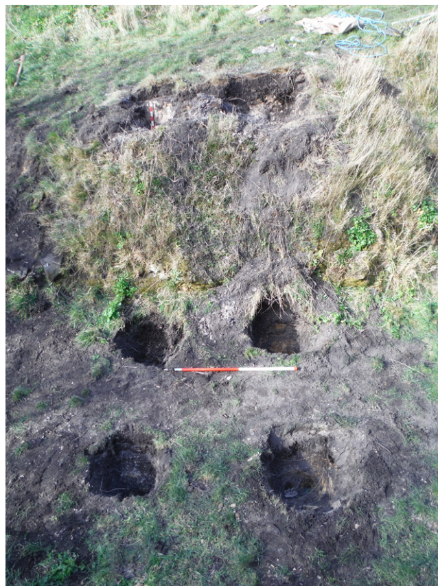
Fig. 3: Post-excitation shot showing foundation holes for staircase footings
