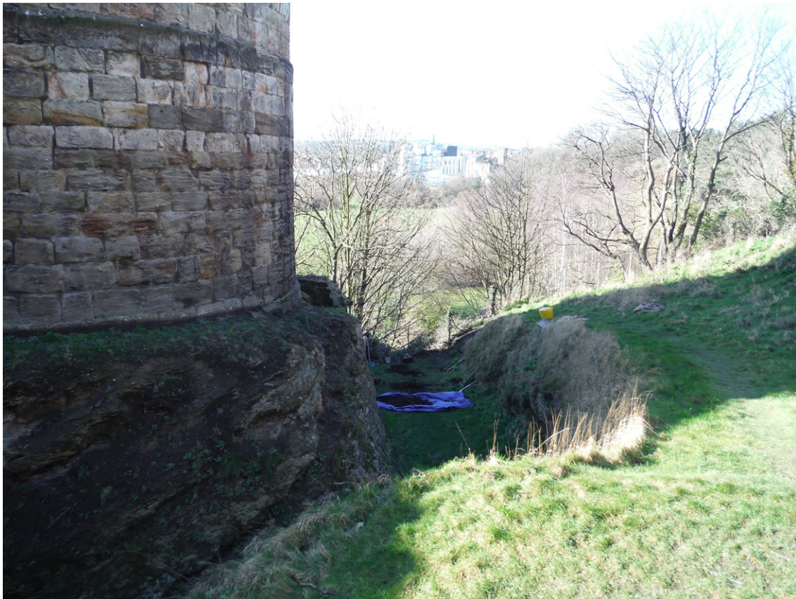
Fig. 2: General location shot showing rock-cut ditch
