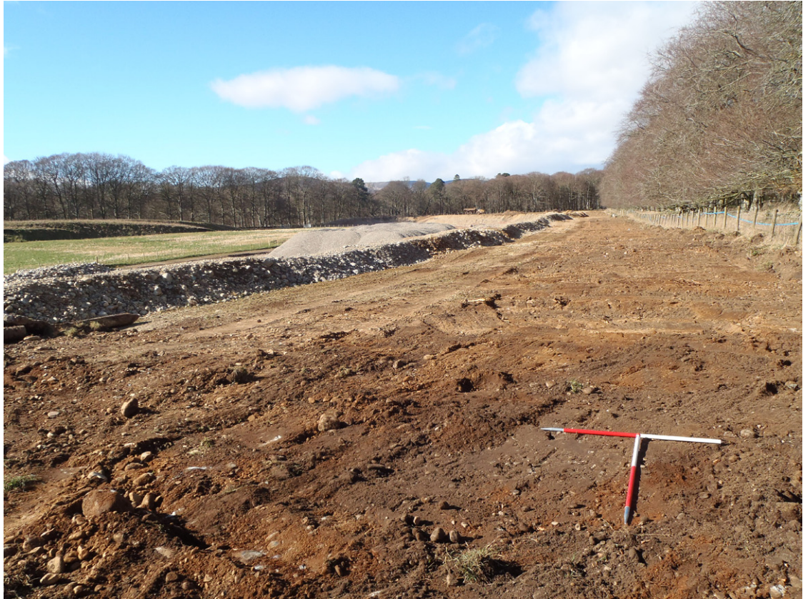
Fig. 6: Post-ex shot of stripped area adjacent to Phase 10/1
