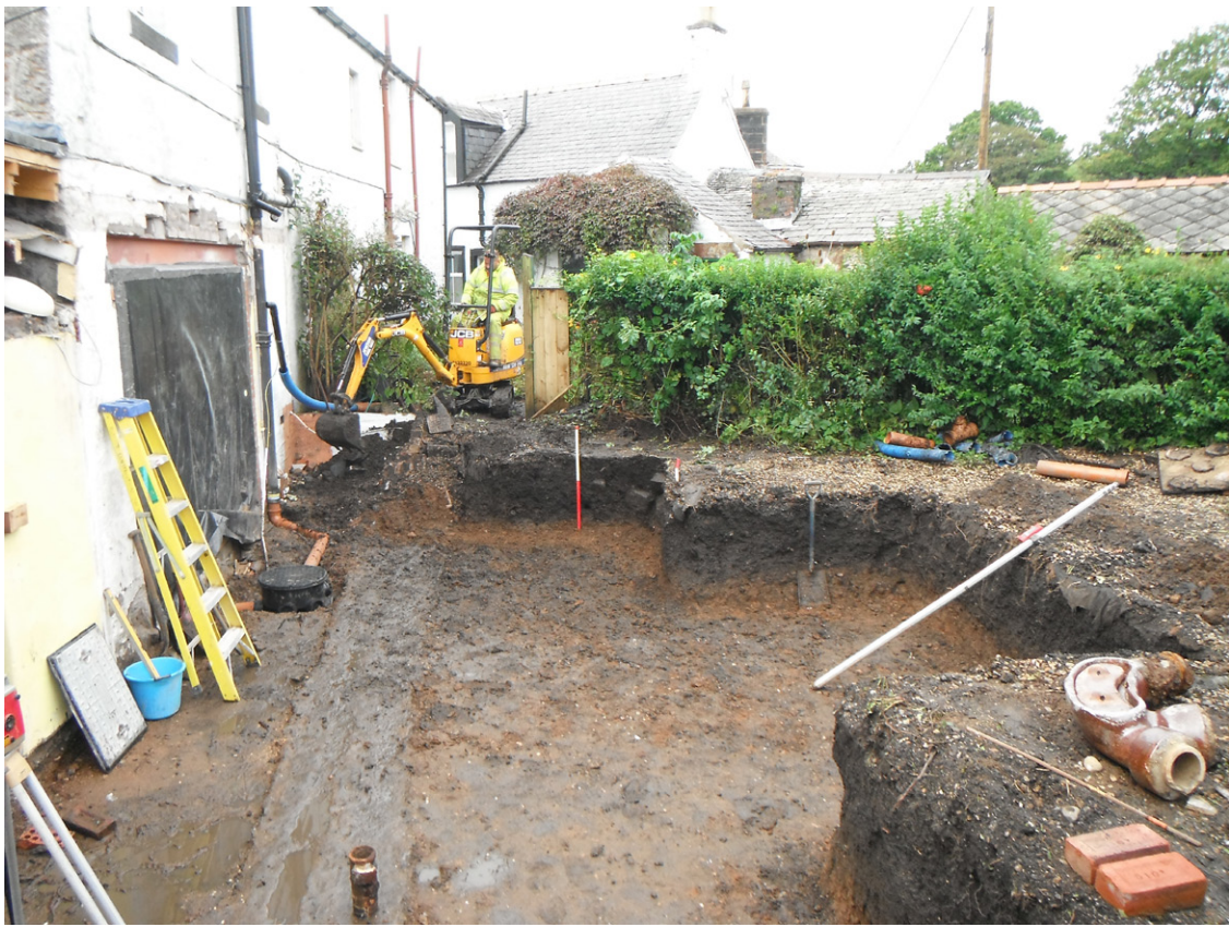
Fig. 5: The completed excavation from the East
