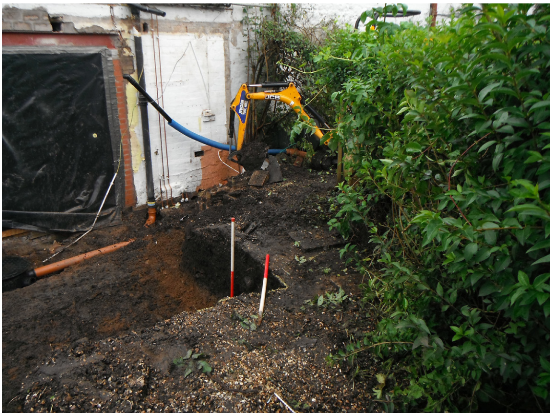
Fig. 8: The alignment of structure 010, roughly parallel with the existing plot boundaries
