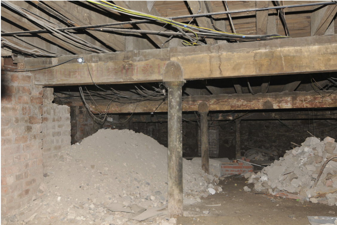
Fig. 16 - Cast iron columns supporting the auditorium floor
