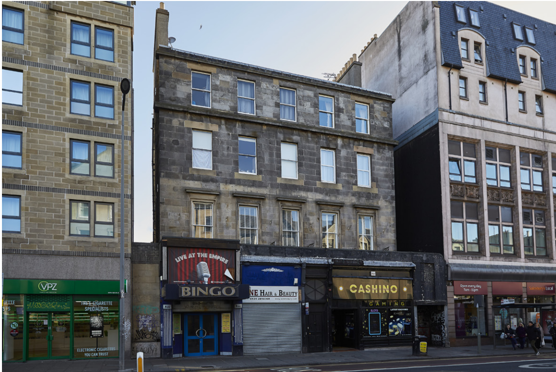
Fig. 4 - 50 Nicolson Street frontage showing the main entrance to the former Empire Bingo Hall
