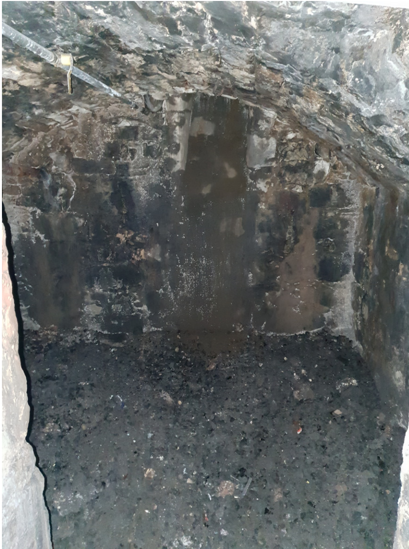
Fig. 18 - Vaulted coal store for a coke fired boiler
