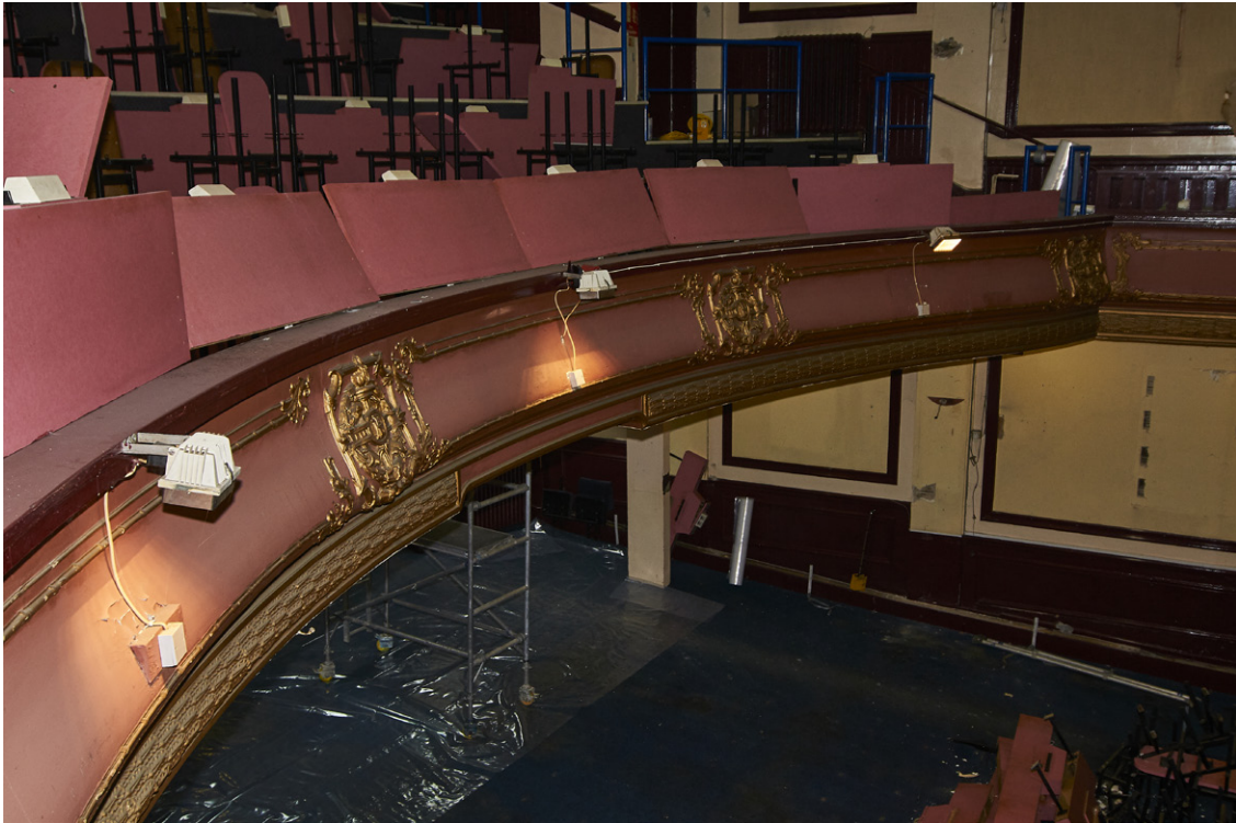
Fig. 12 - Embellished balcony front with heraldic detailing
