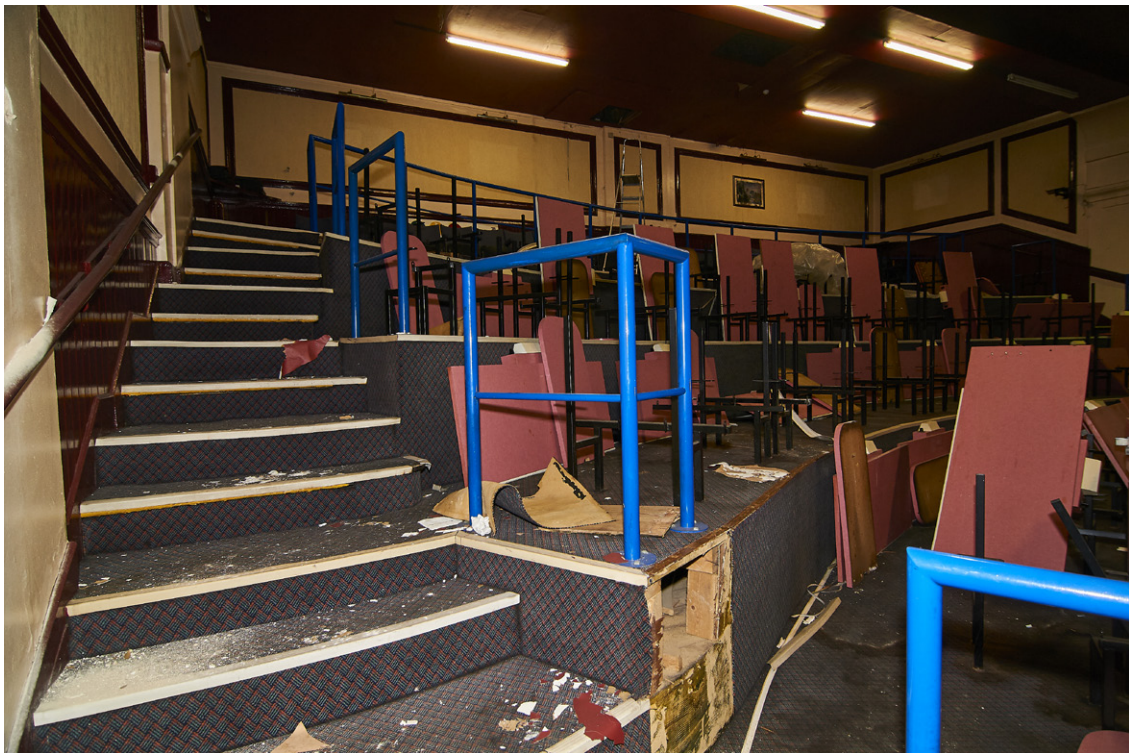
Fig. 11 - Stairs to the rear of the circle floor
