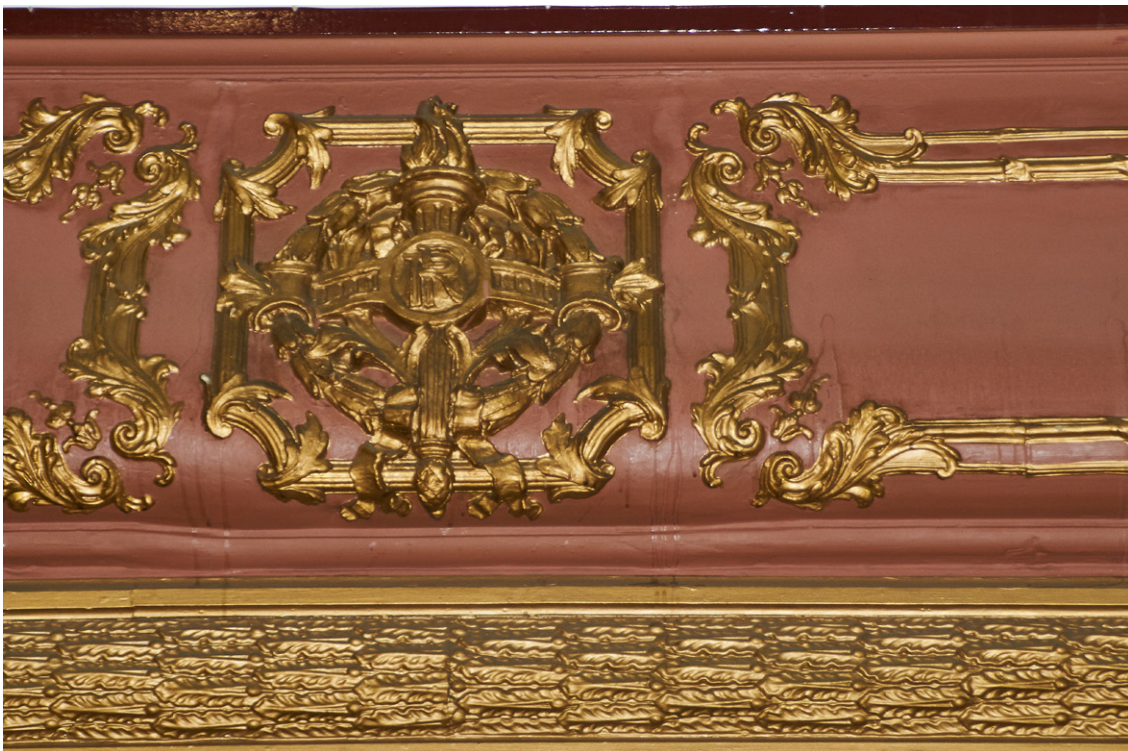
Fig. 13 - Detail of a boss incorporating the initials RP (Royal Princess) and leaf and scroll plasterwork
