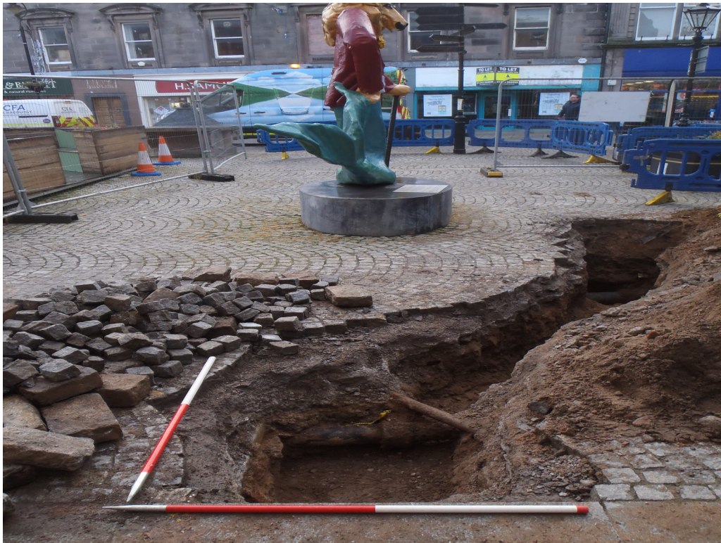
Fig. 3 - General shot of completed excavation
