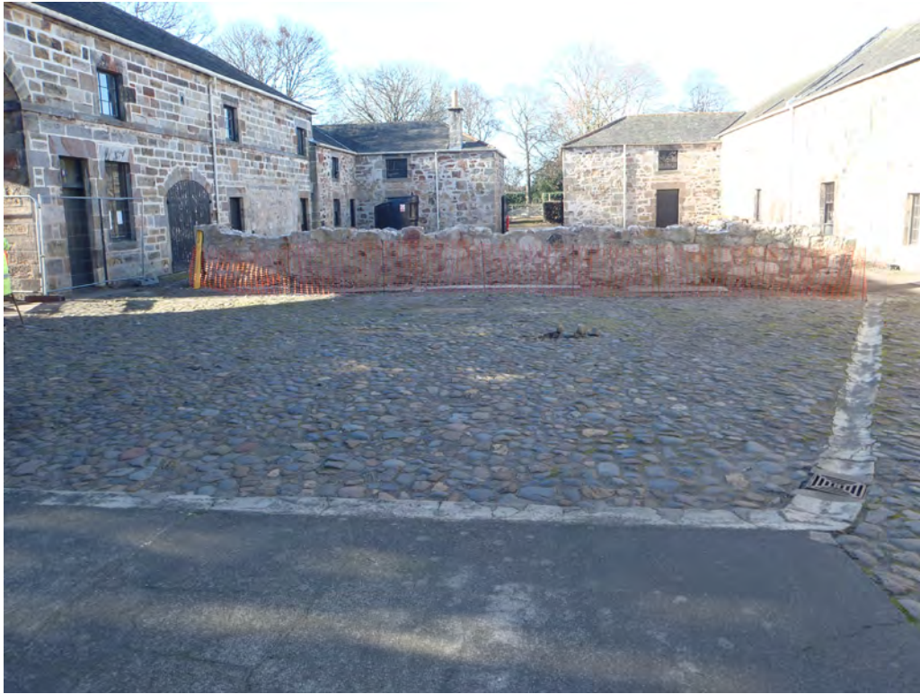
Fig. 5 -Pre-ex view of cobbles (001) and wall (156) in N half of courtyard
