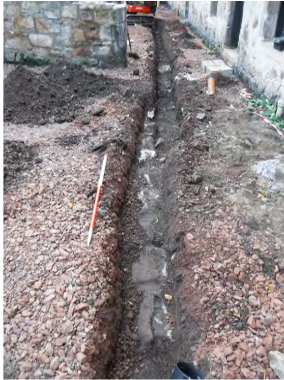
Fig. 21 - Culvert capping stones (096) in Tr12
