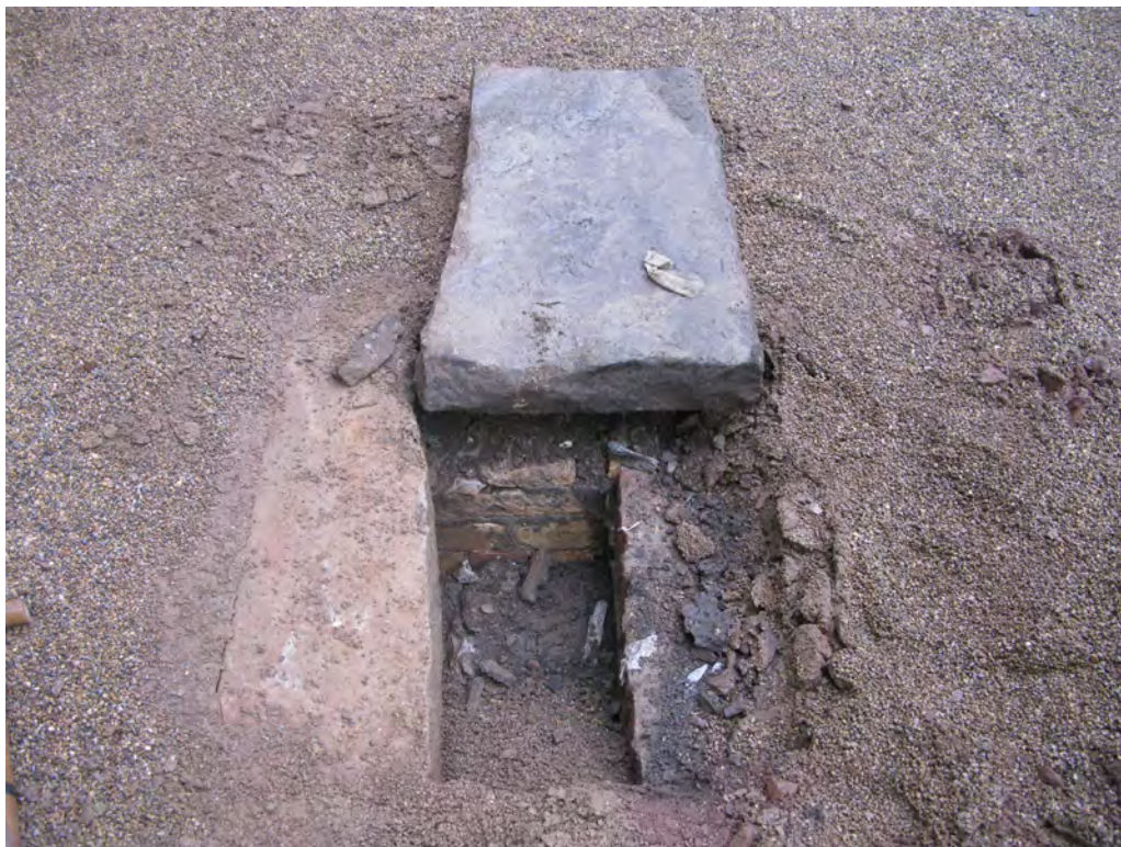
Fig. 22 - Manhole (062) outside Newhailes House, Tr20
