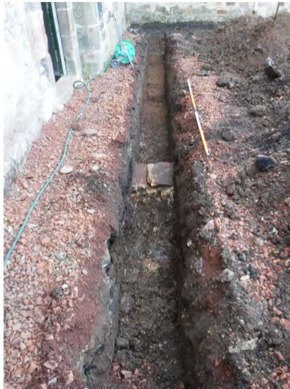
Fig. 16 - Wall (033) in Tr7
