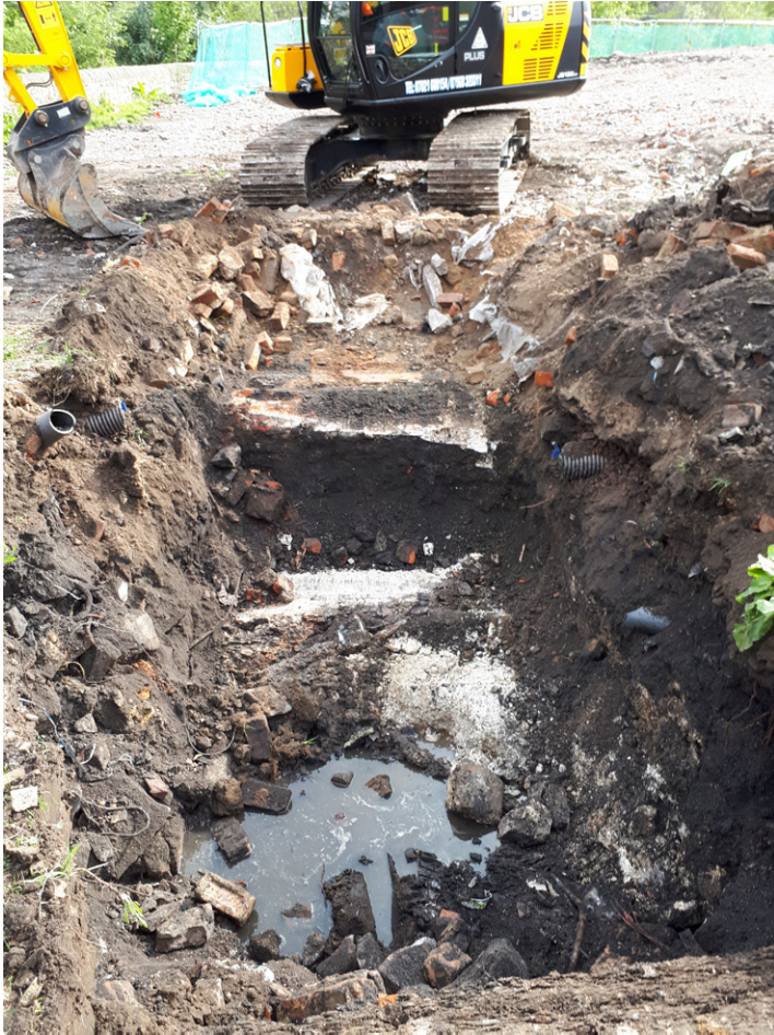
Fig. 19: Trench 5 showing wall (505)
