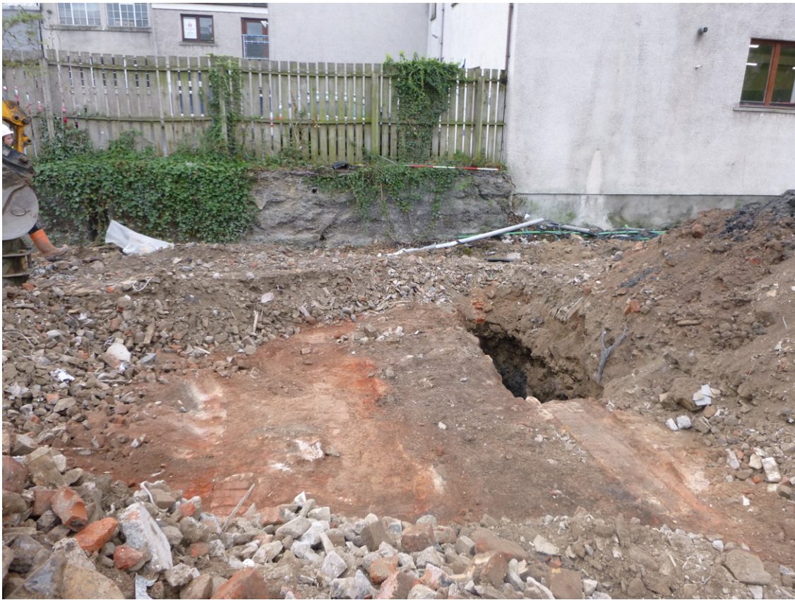
Fig. 24: Site Investigation pit showing surviving brick flue structure
