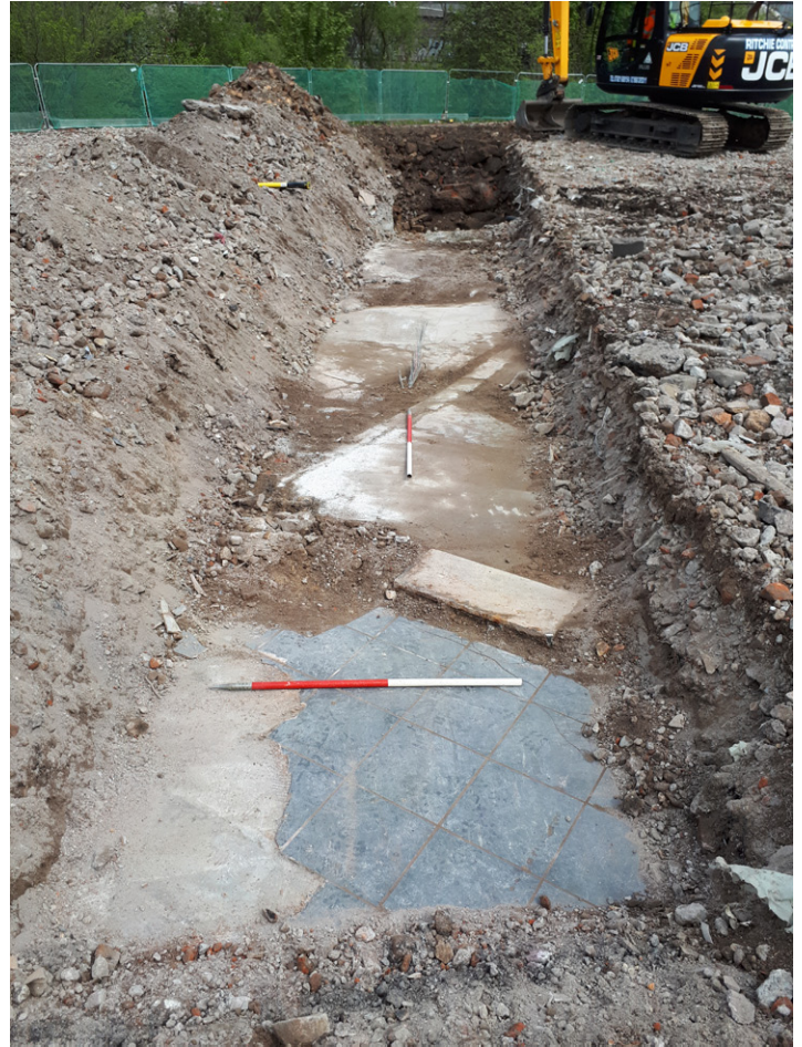
Fig. 20: Trench 6 showing tiles (602), Concrete (603) and stone wall or kerb (604)
