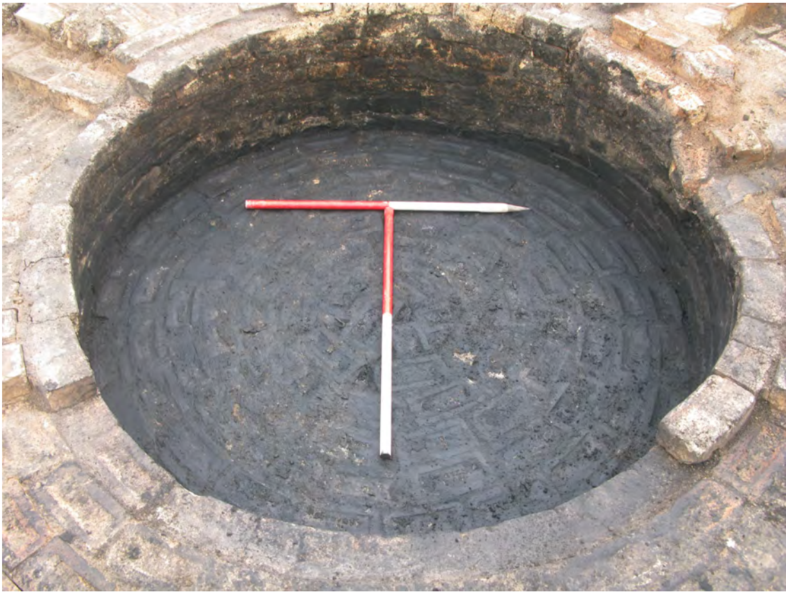
Fig. 11: Brick chimney base (123)
