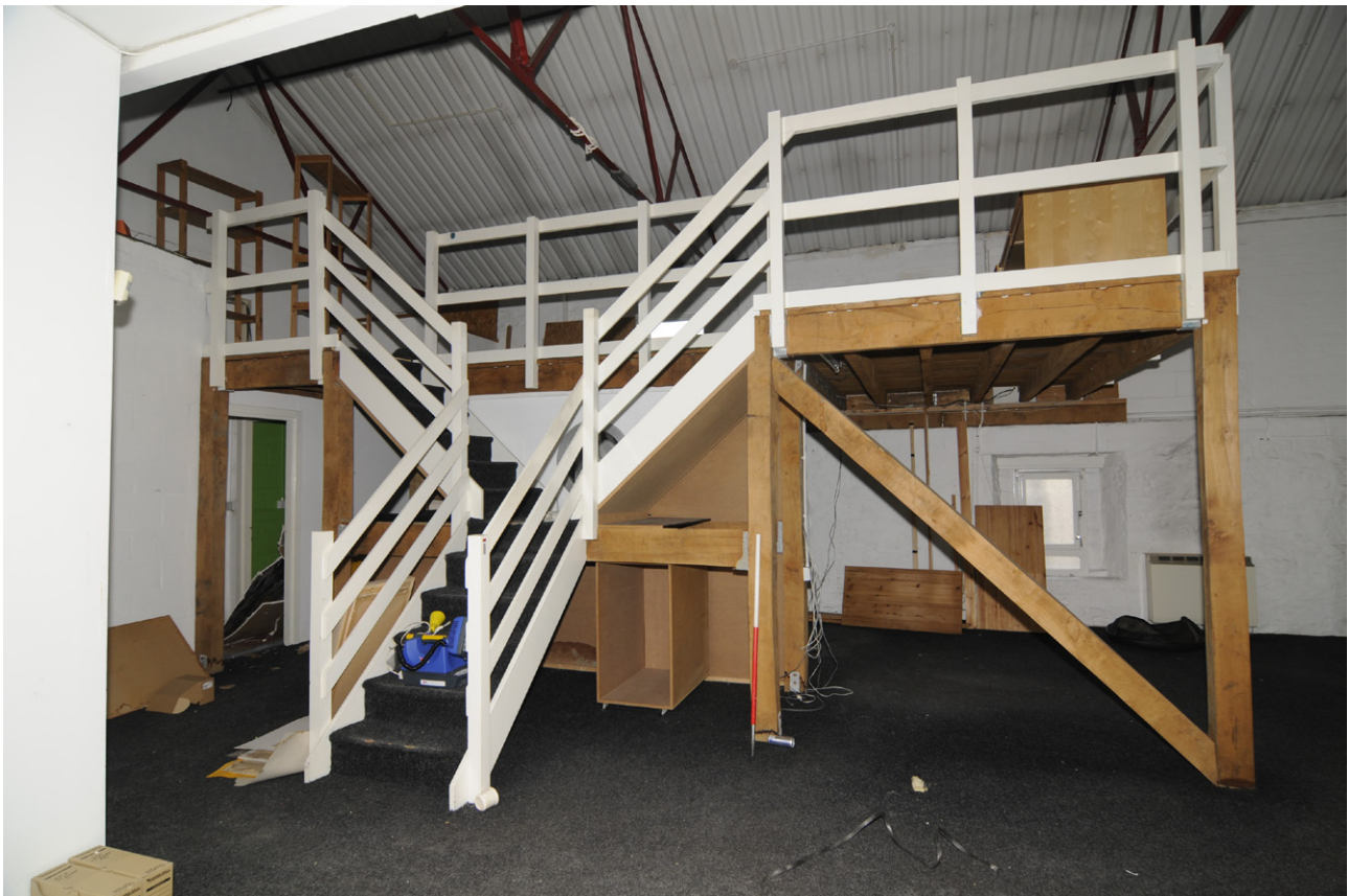
Fig. 22: Timber-framed mezzanine on the second floor in Building H, (Room H1)
