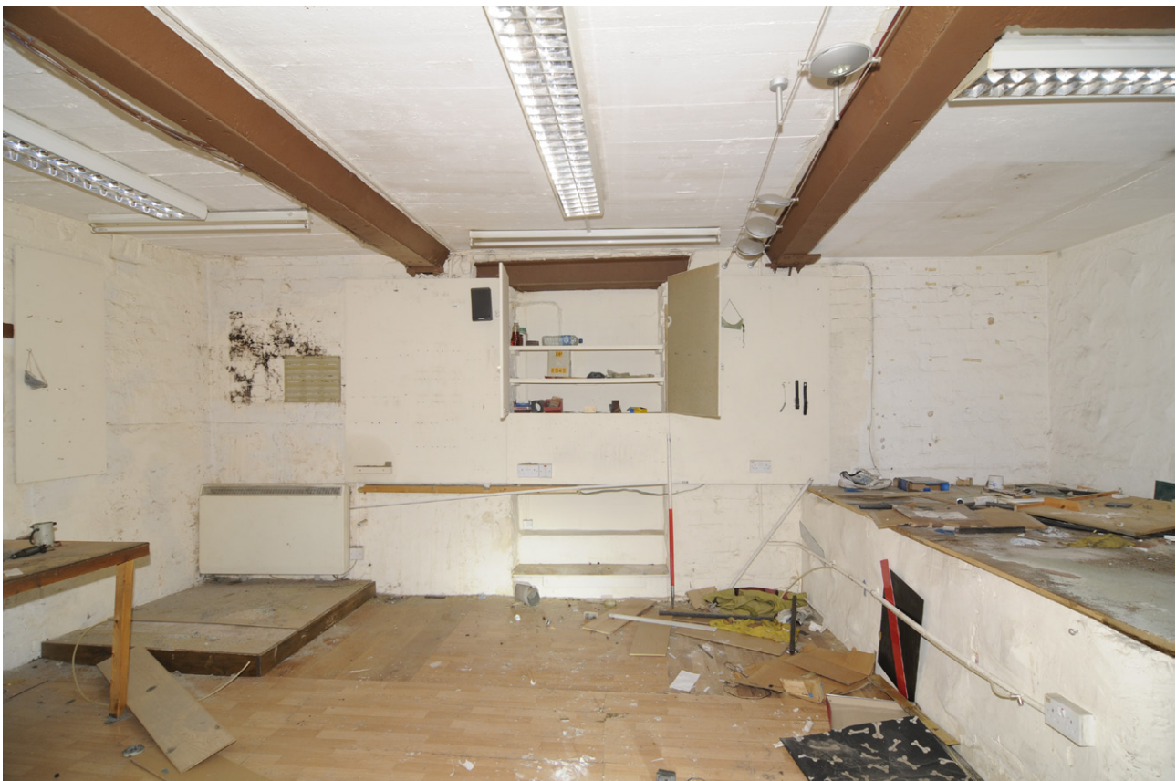
Fig. 19: Earlier blocked doorway on the south wall of the engraving workshop (Building F, Room F1)
