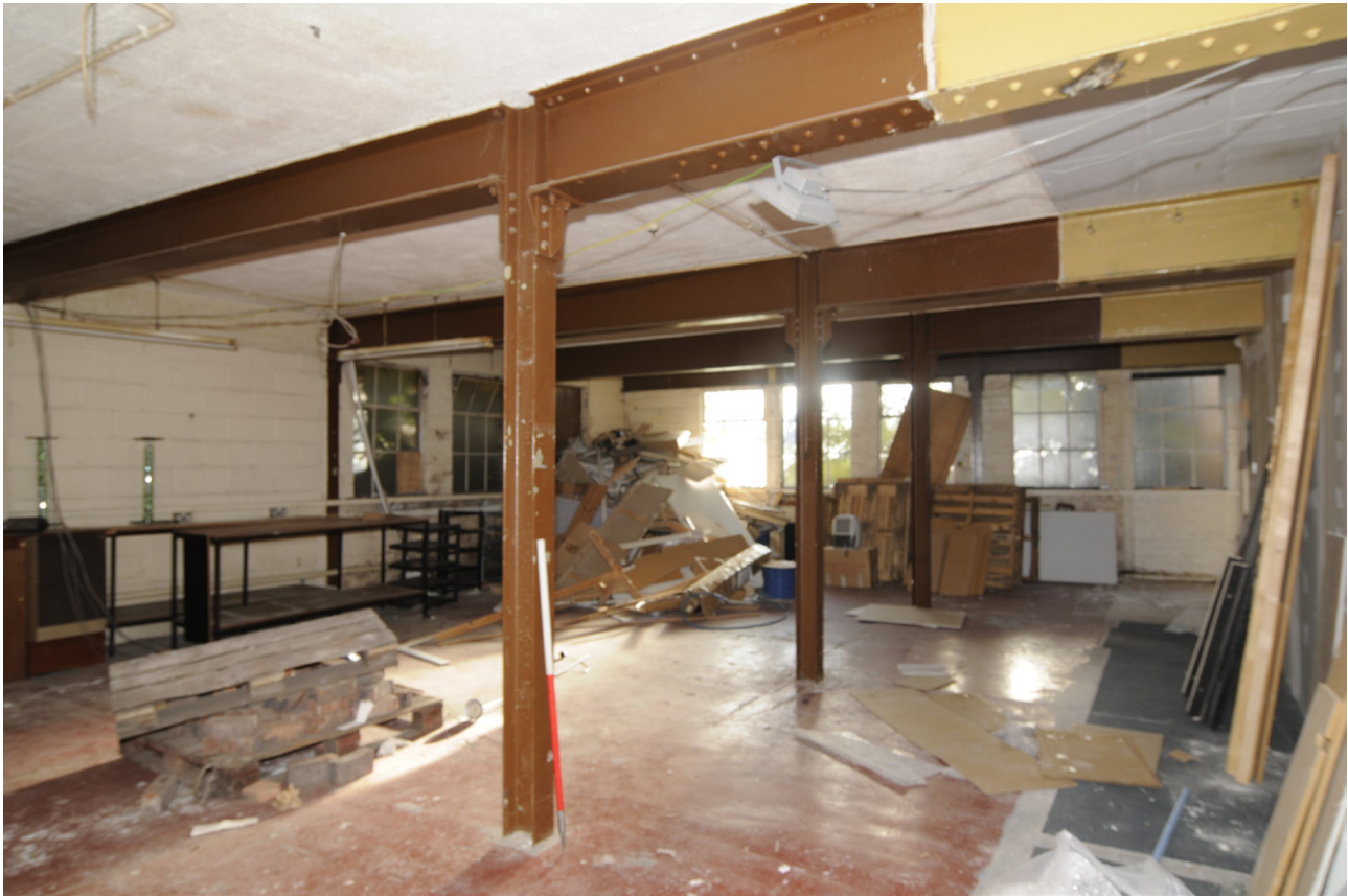
Fig. 24: Ground floor showing load-bearing steel frame Building I, Room I3)
