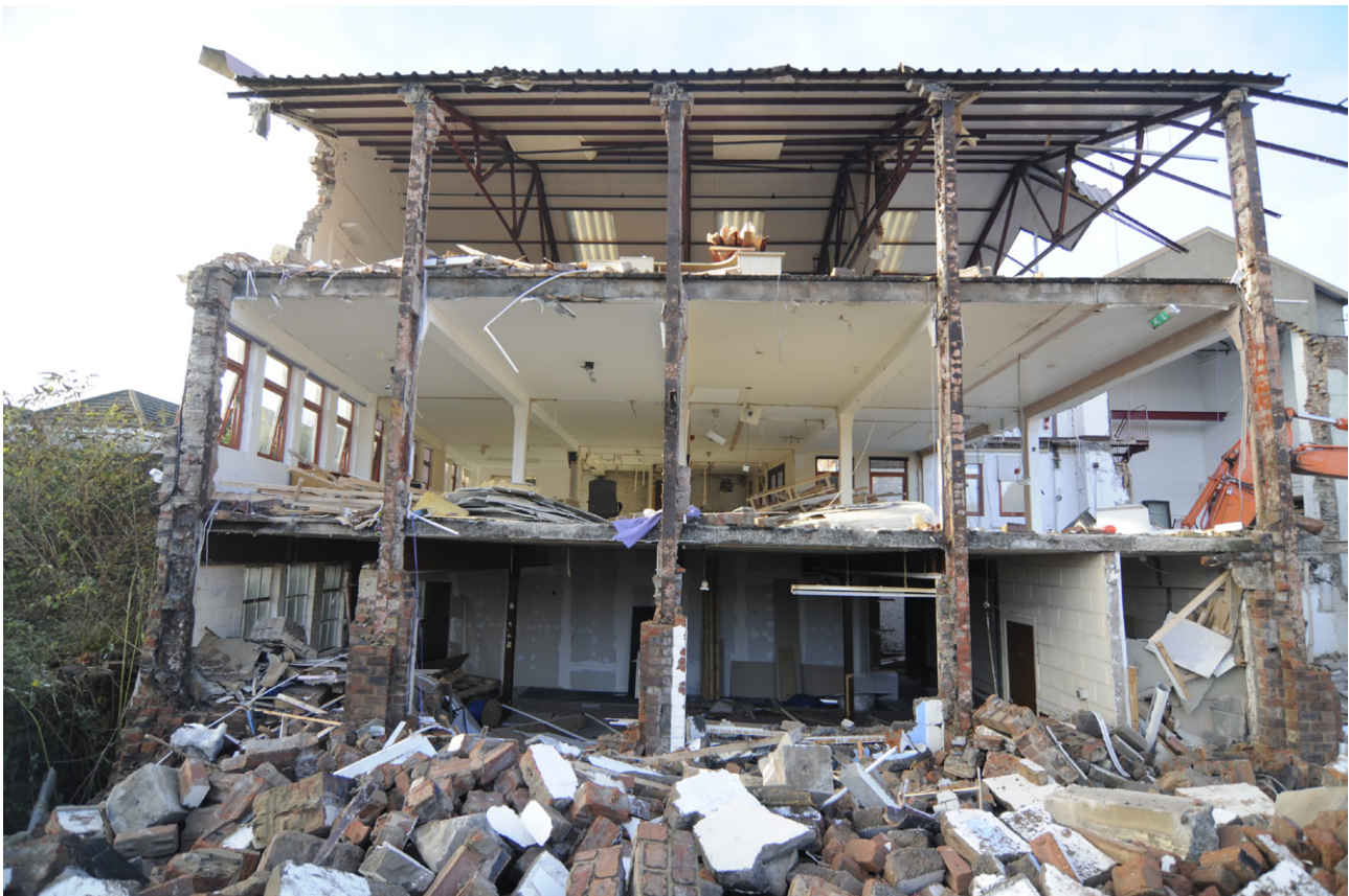
Fig. 35: Building I during demolition showing its exposed steel frame
