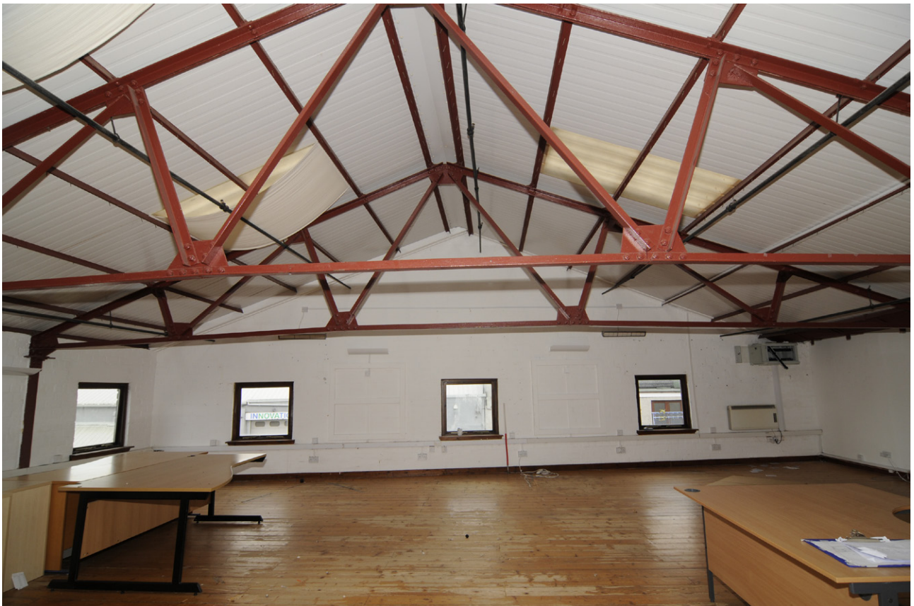
Fig. 27: Second floor of Building I showing composite double-fink wide span joists (Building I Room I20)
