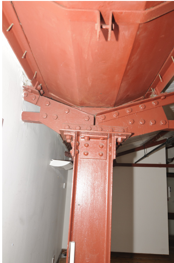
Fig. 28: Load bearing pillar with fish-plates supporting the a steel roof valley (Building I, Room 20)
