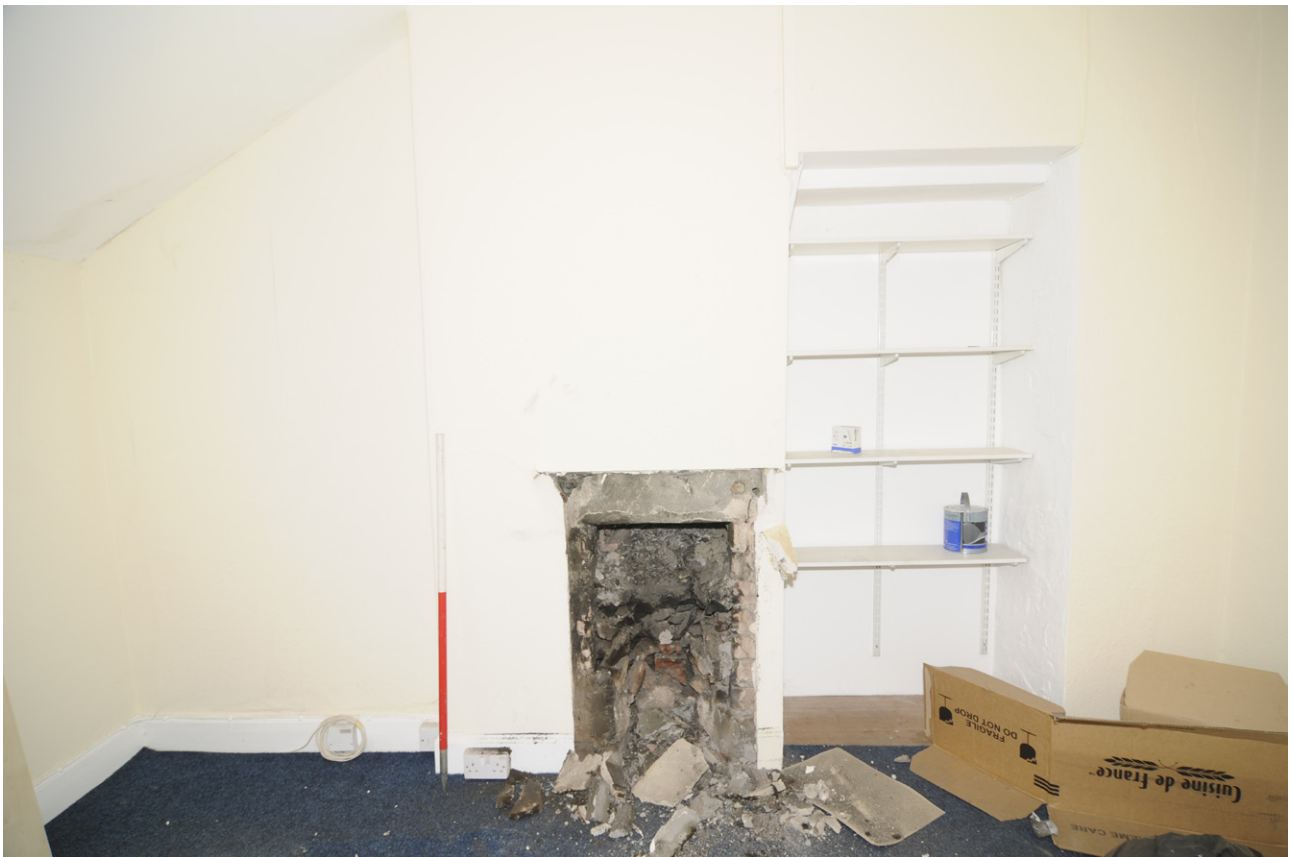
Fig. 11: Interior first floor office with robbed fireplace Building B, Room B12)
