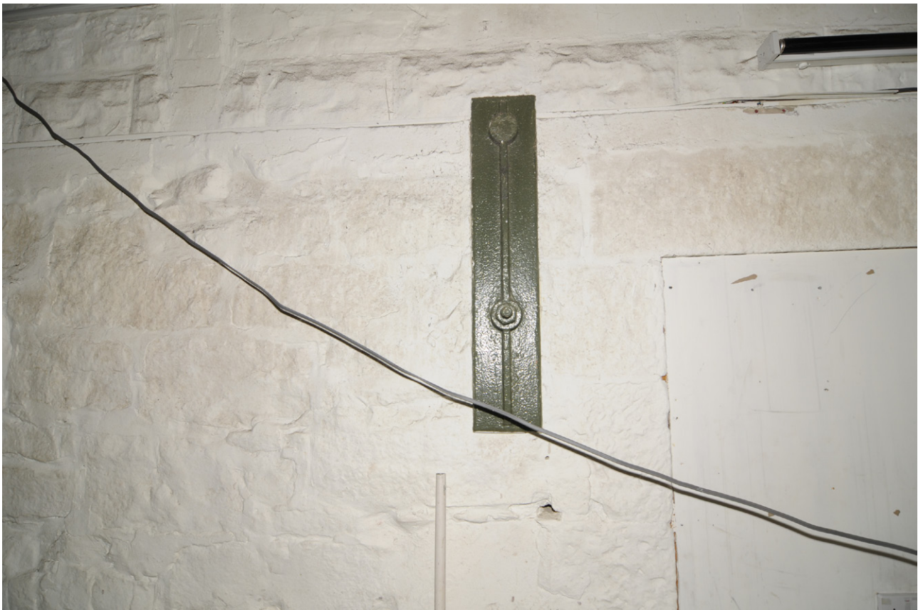
Fig. 13: Detailed shot of one of the tie-plates on a former gable wall of Building D
