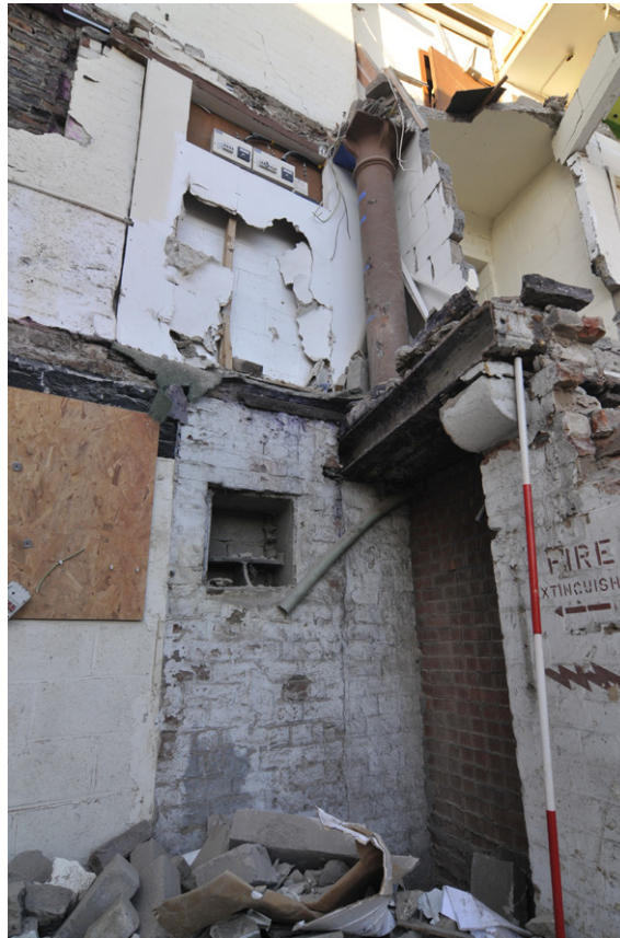
Fig. 36: Exposed cast-iron bearing box and cast-iron column on the floor above (Building F, Room F1)
