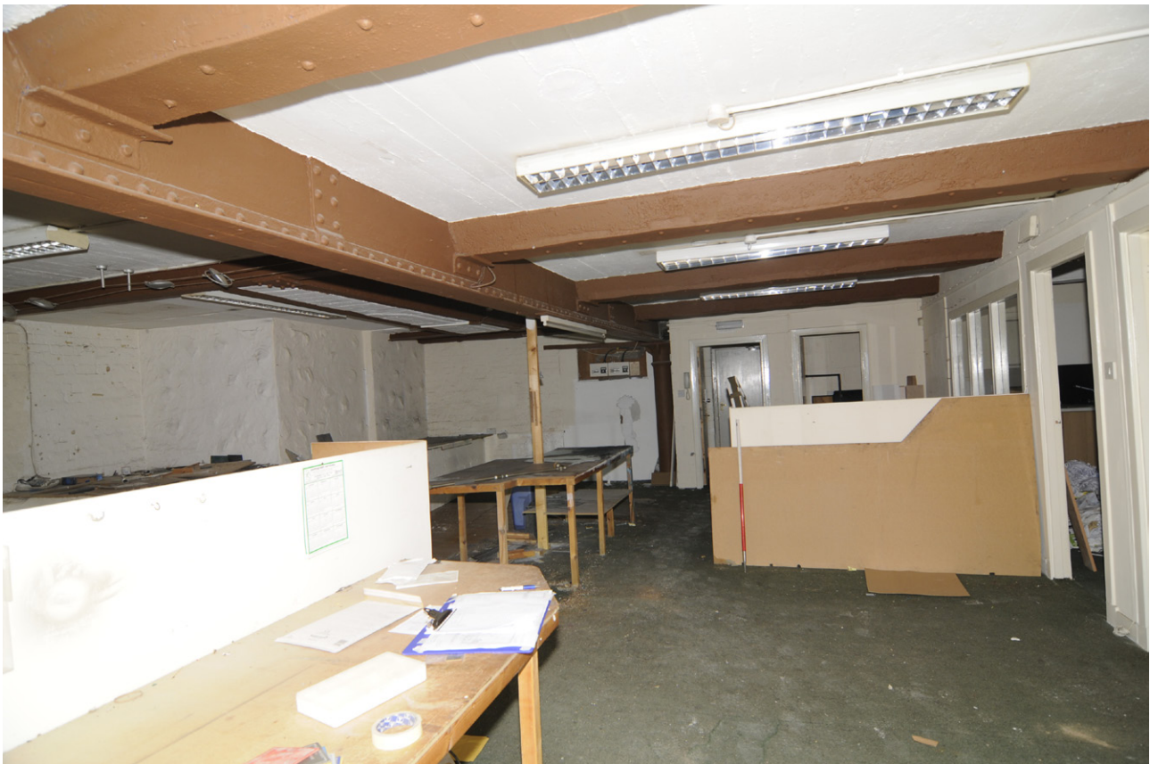
Fig. 18: Open plan workshop and office suite on the first floor of Building F showing riveted steel frame (Room F1)
