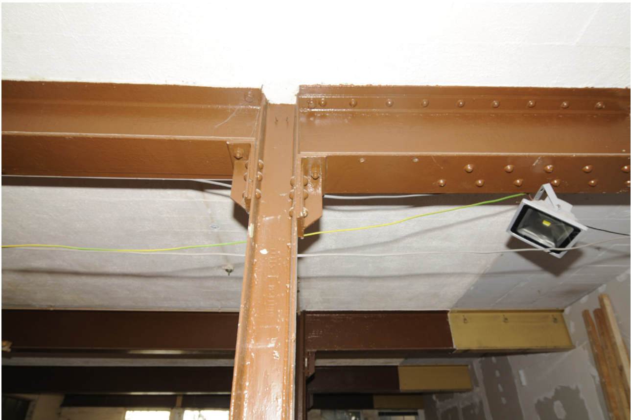
Fig. 25: Detail shot of the I-beams and shoes on the pillar heads that support them (Building I, Room I3)
