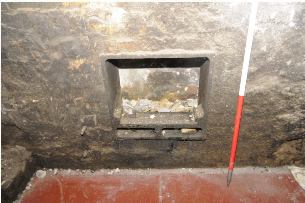
Fig. 17: Detailed shot of the bearing box in Building E1
