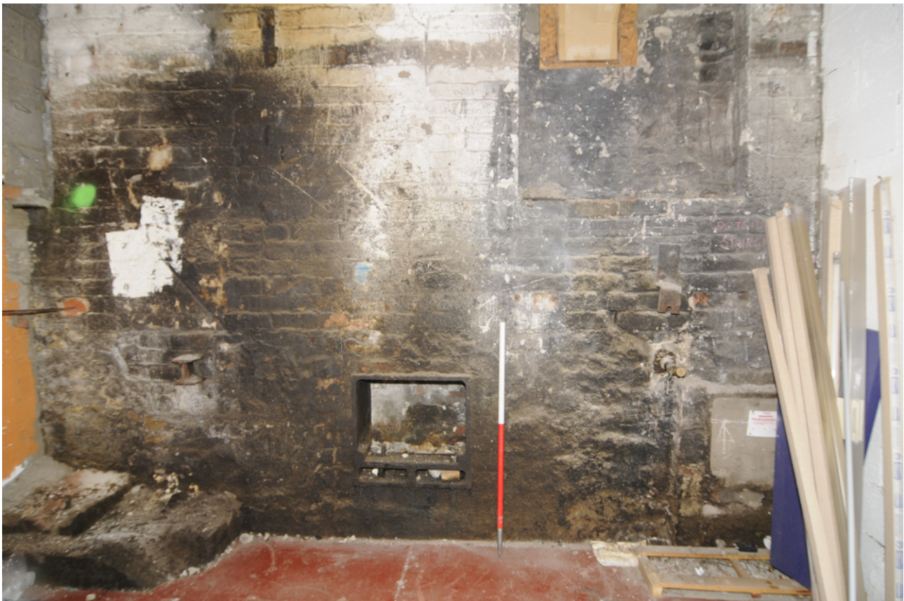
Fig. 16: Central cast-iron bearing box and blocked window on the ground floor of Building E, Room E1
