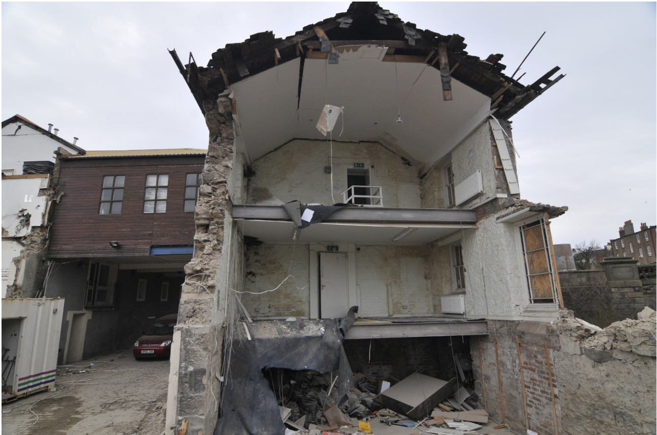
Fig. 38: Section exposed through Building A revealing its gable wall below the pitched roof. Blocked fireplaces and cupboards can be seen to the right of the later inserted doorways
