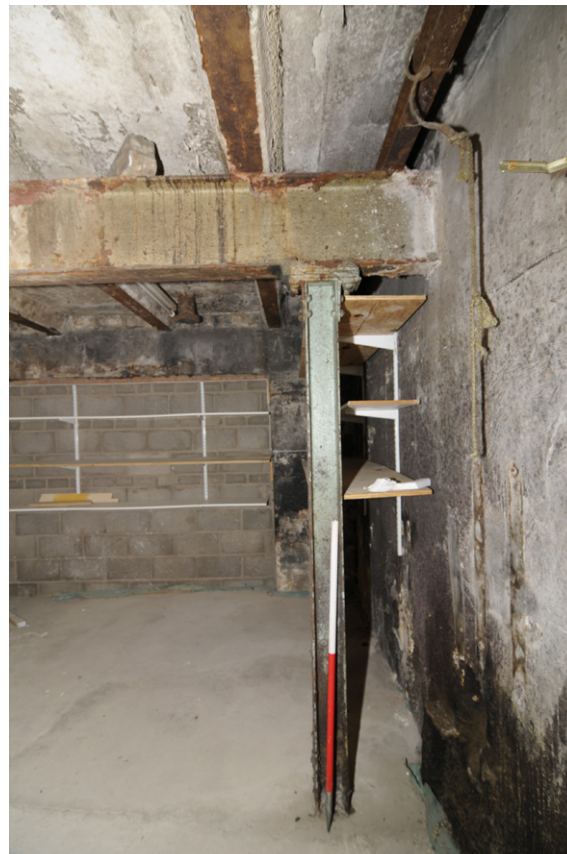
Fig. 15: Part of the load-bearing steel frame at the west end of Building D, D1
