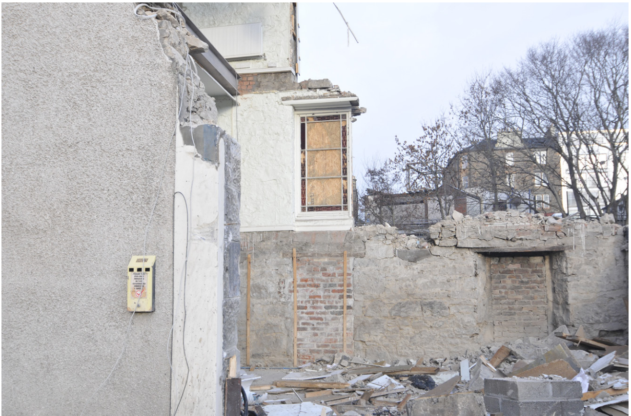
Fig. 37: Blocked ground floor doorways and ornate glazed window on the first floor (Building A, Room A3)
