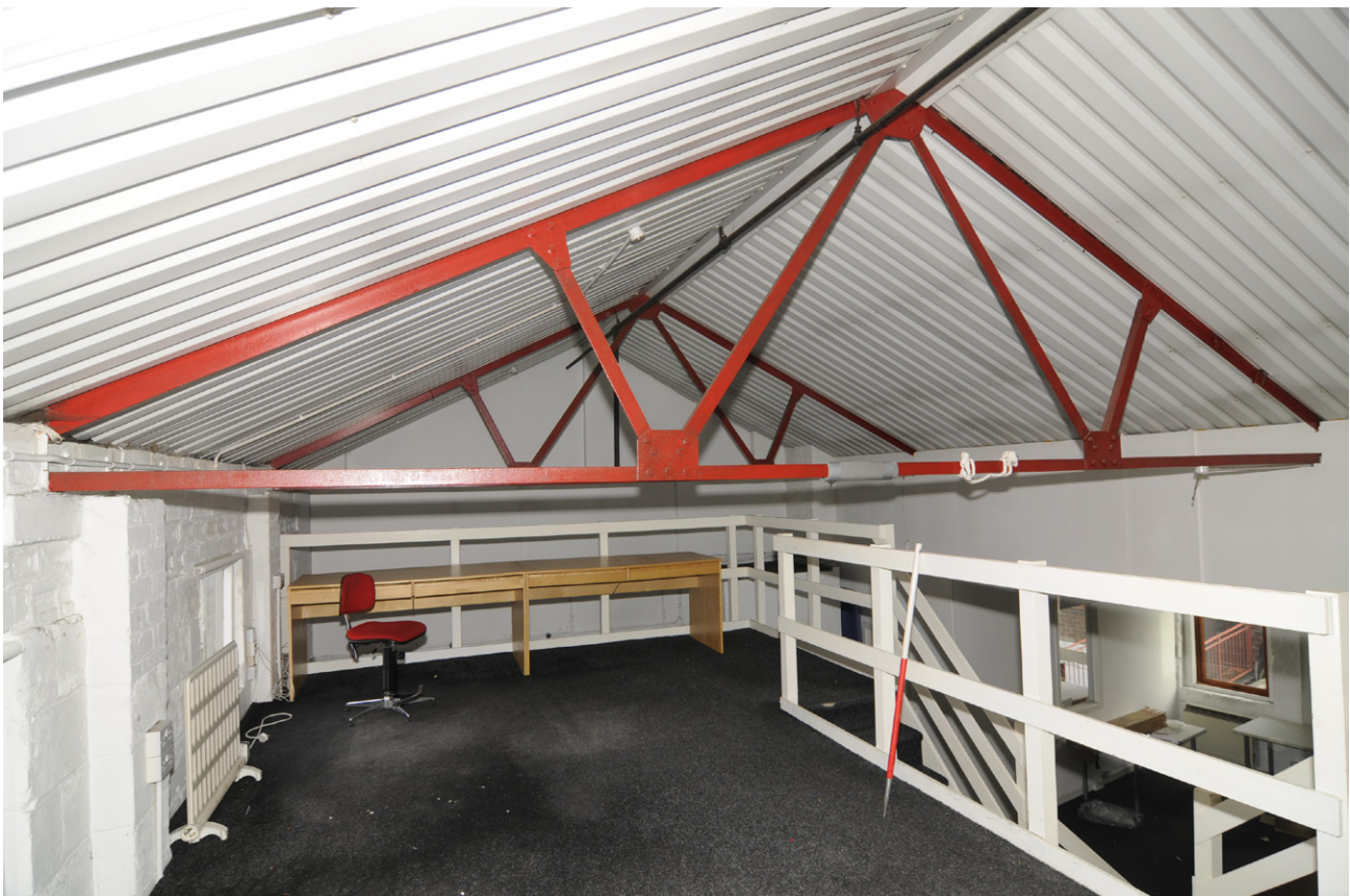
Fig. 23: Composite steel roof truss in Building H (Room H1)
