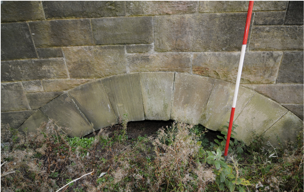
Fig. 32: Detailed shot of the segmented arch of the North Lade
