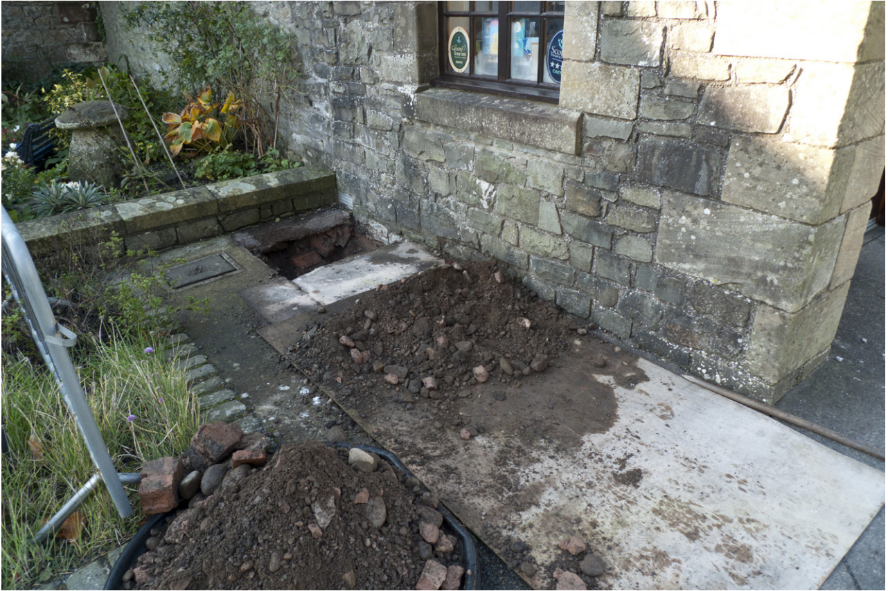
Fig. 2: General view showing area of works, from NE
