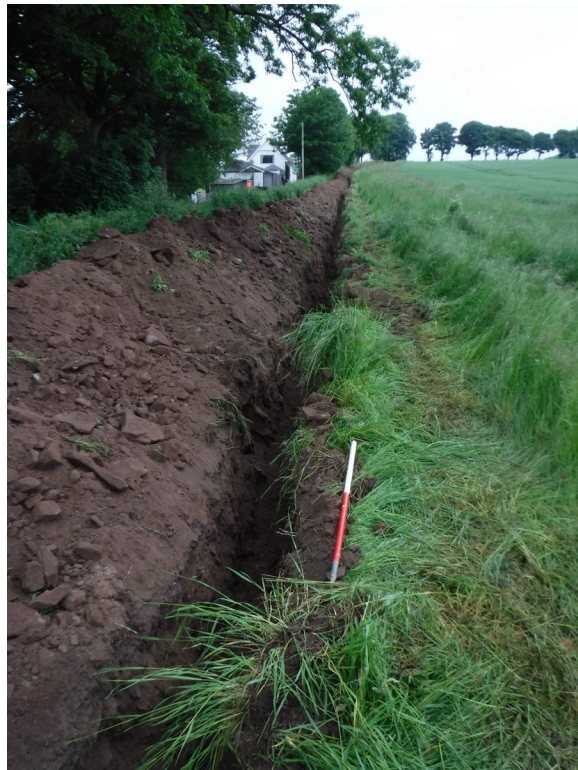
Fig. 3 - Excavated trench from the south-eastern end looking north-west
