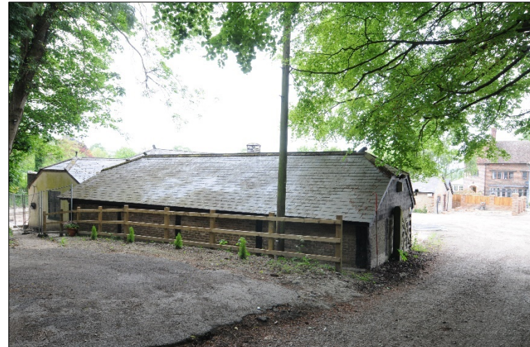
Photograph 4: Setting shot showing garage in relation to manor house
