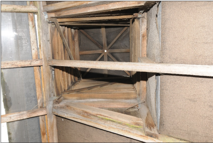
Photograph 27: Inside of the wooden roof ventilator
