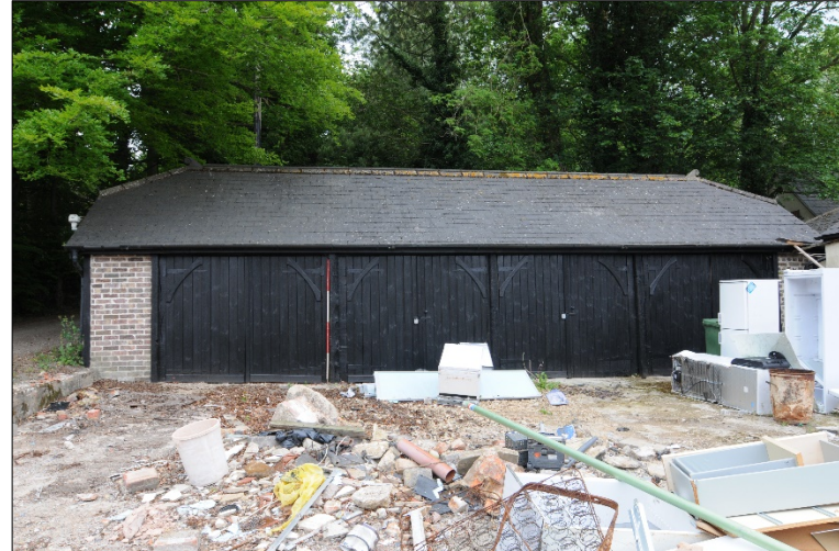
Photograph 2: North-west elevation of garage
