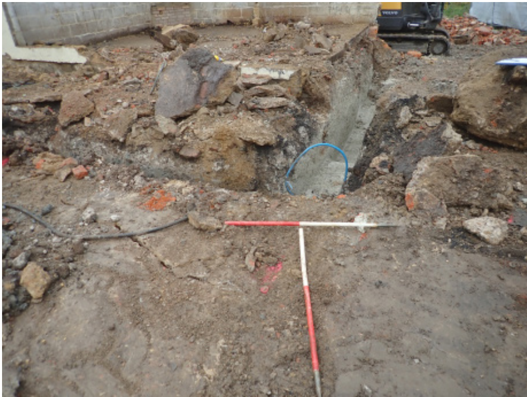
Fig.4.3 - Watching Brief – service trench (east of stables)
