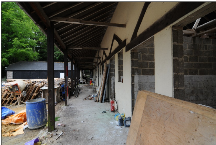
Photograph 11: Covered walkway at north-east side of stable block (looking south-east)
