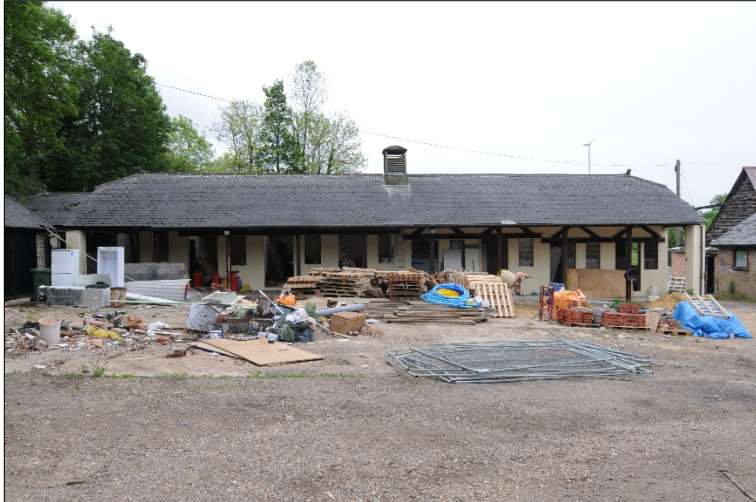
Photograph 1: North-east elevation of stable block
