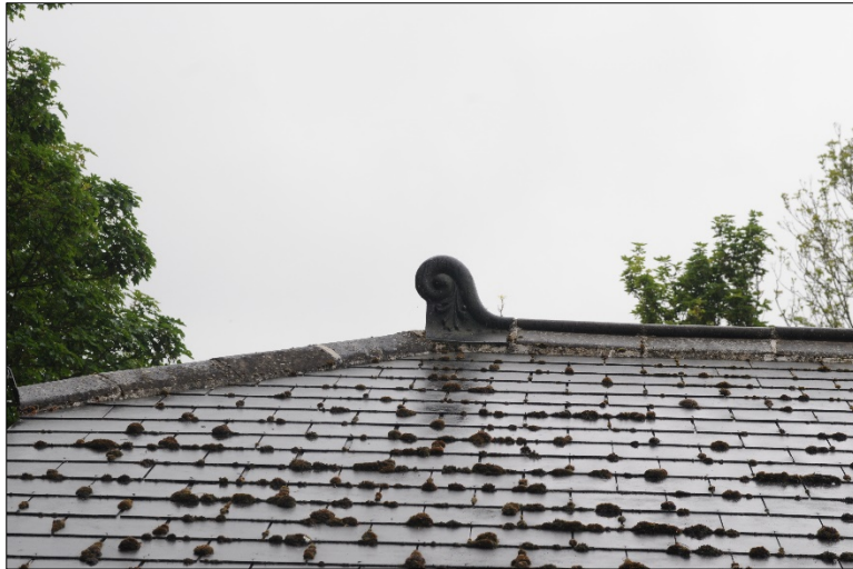
Photograph 21: Spiral finial on the hipped south-east end of stables
