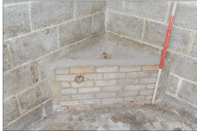
Photograph 30: Detail of the corner trough in Stable No. 3 showing tethering ring
