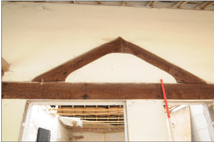
Photograph 17: Inset timber feature above stable doorway
