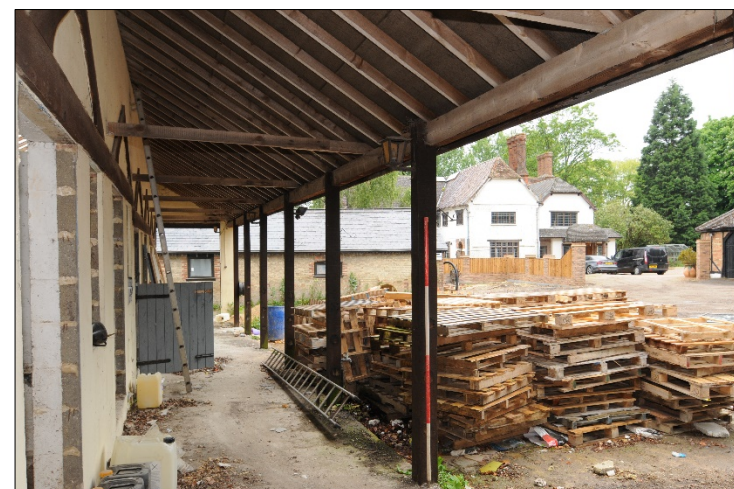
Photograph 12: Covered walkway at north-east side of stable block (looking north-west)
