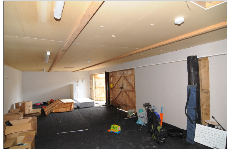
Photograph 22: Interior of the garage showing a suspended ceiling and wall cladding
