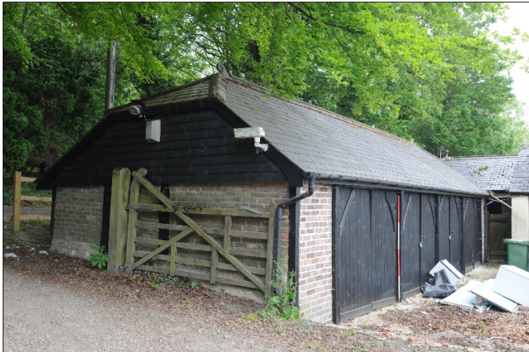
Photograph 3: East corner of garage showing hipped roof and timber posts infilled with modern brick
