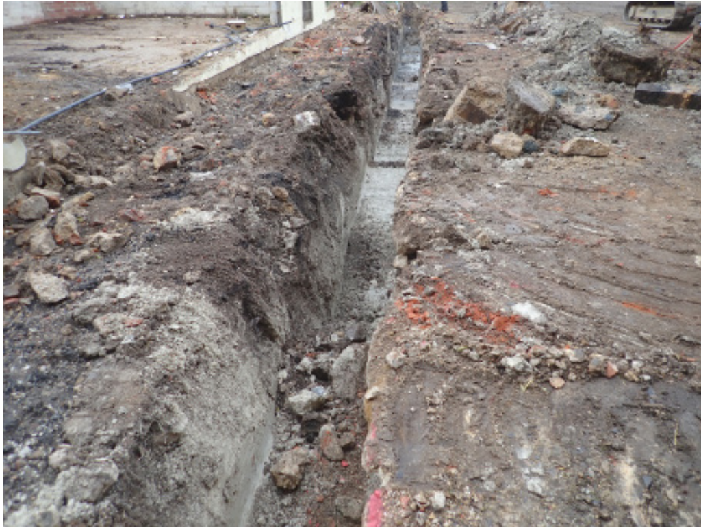
Fig. 4.2 - Watching Brief – service trench (north of stables)
