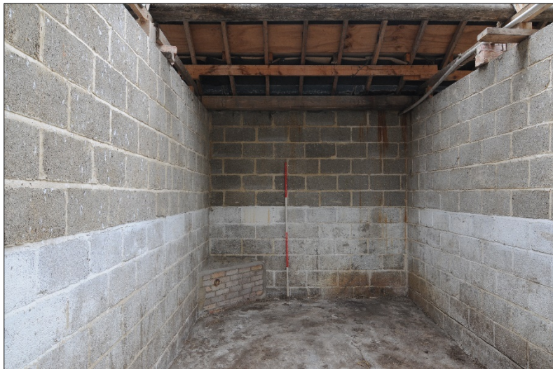
Photograph 31: Internal view of Stable No. 3 showing corner trough
