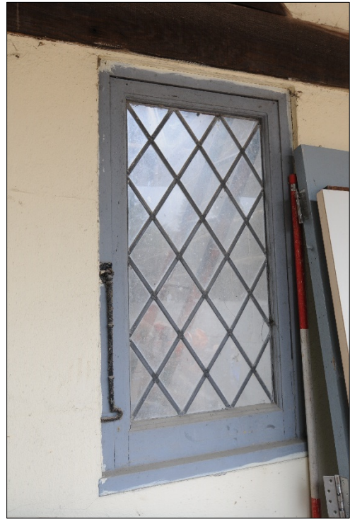
Photograph 14: Casement window in north-east elevation of stable block
