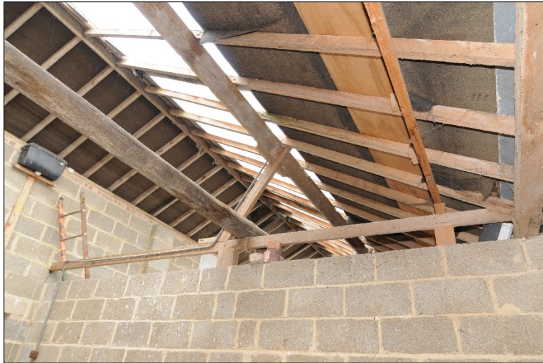
Photograph 29: Softwood purlins and rafters over the stables
