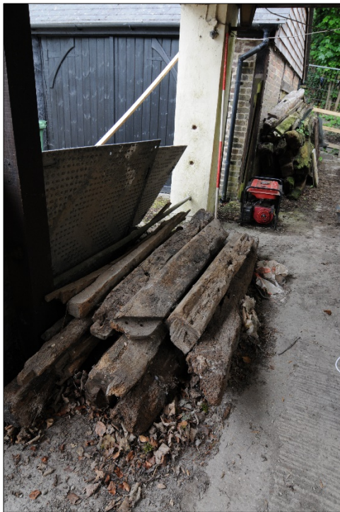
Photograph 15: Old roof timbers, some of which have pegged tenon joints
