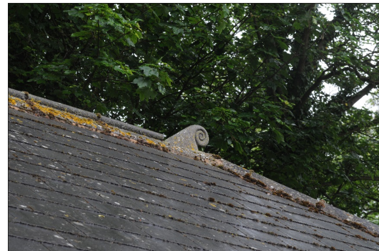
Photograph 20: Spiral finial on the hip of the south west end of the garage
