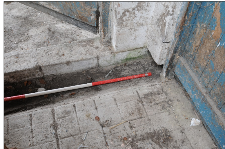
Photograph 24: Drain running along north-east edge of stables
