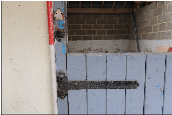
Photograph 13: Strap hinge to the stable doors
