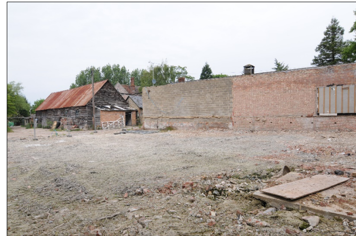
Photograph 8: South-west elevation of stable block with timber-framed barn in background
