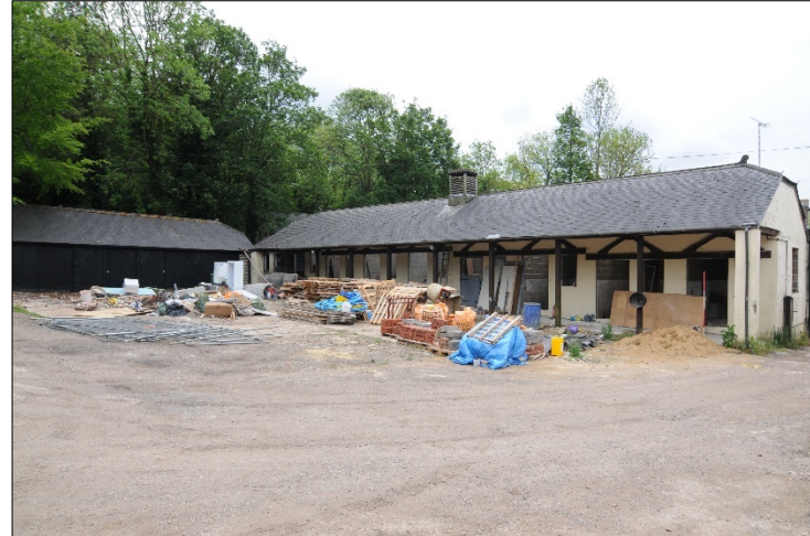
Photograph 10: Setting showing garage and relationship to stable block
