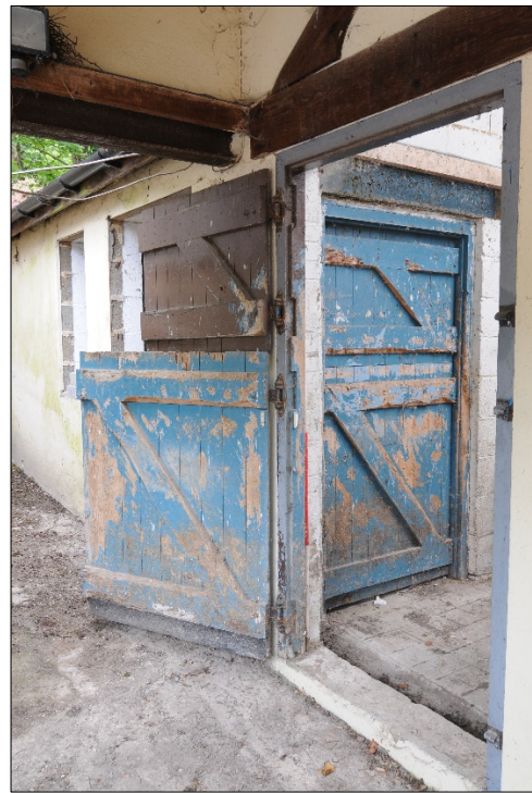
Photograph 16: Wooden stable doors
