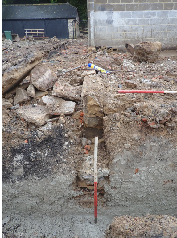
Fig. 4.4 - Overall view of service trenches
