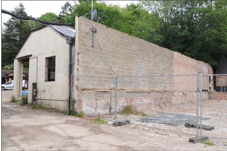
Photograph 9: West corner of stables showing block built up against demolished shed wall
