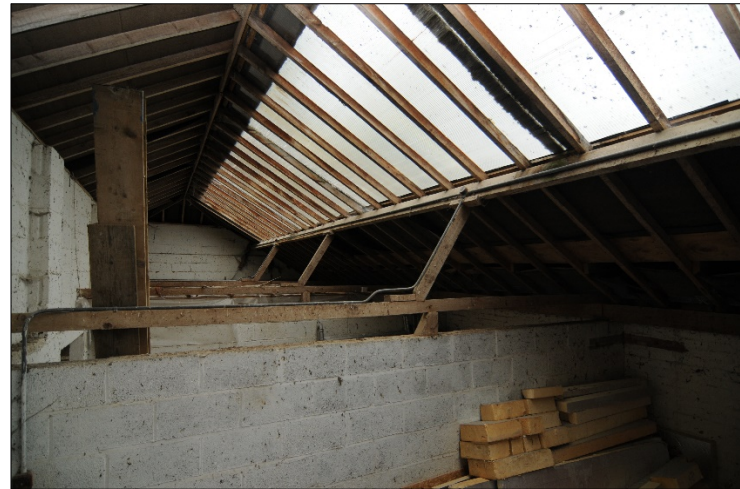
Photograph 26: Roof structure over the stables showing continuous skylight
