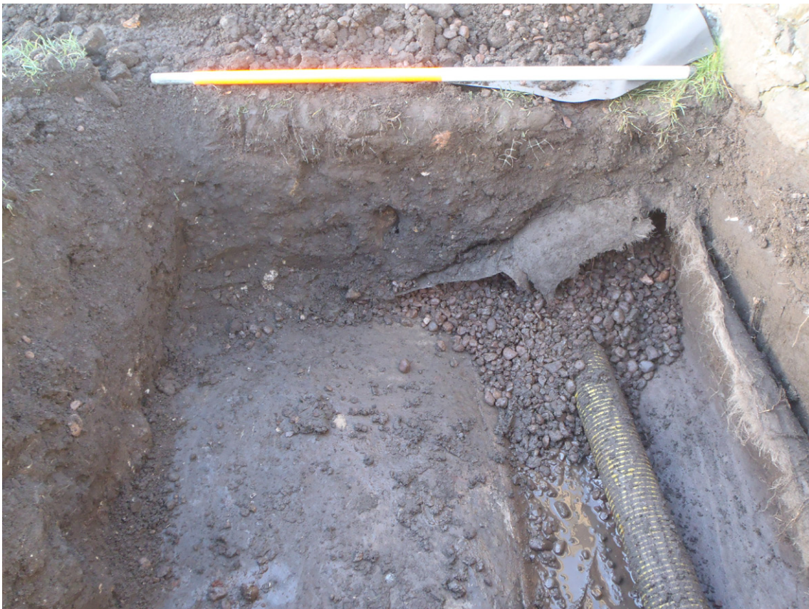
Fig. 3: NE-facing section of Trial Pit 2
