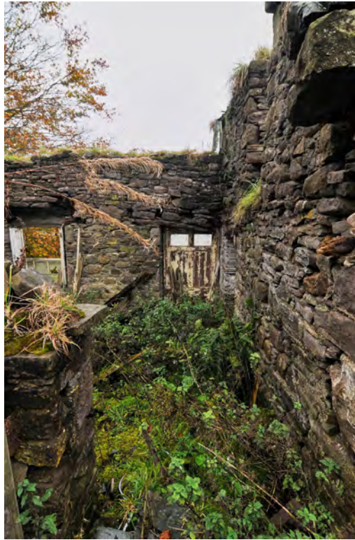
Fig. 11 - Unit 2 interior of the farmhouse with its door and window
