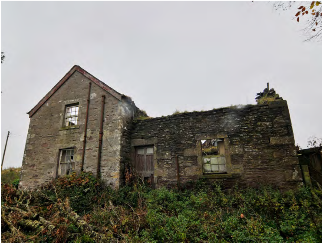
Fig. 5 - The SE elevation of the farmhouse
