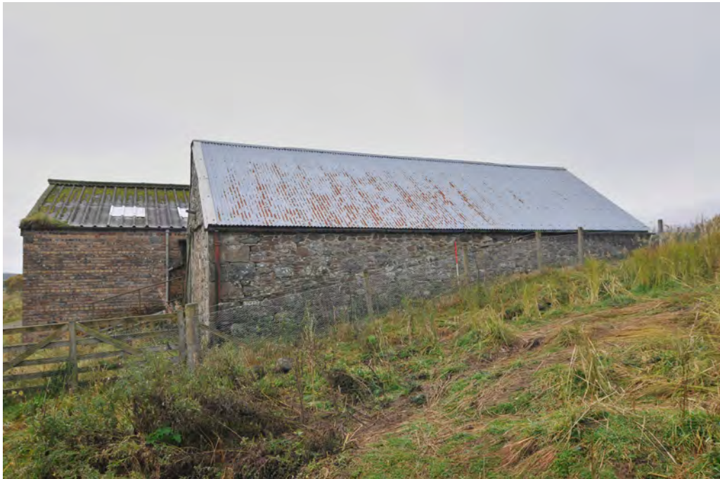
Fig. 16 - Steading exterior, byre wall built into a slope
