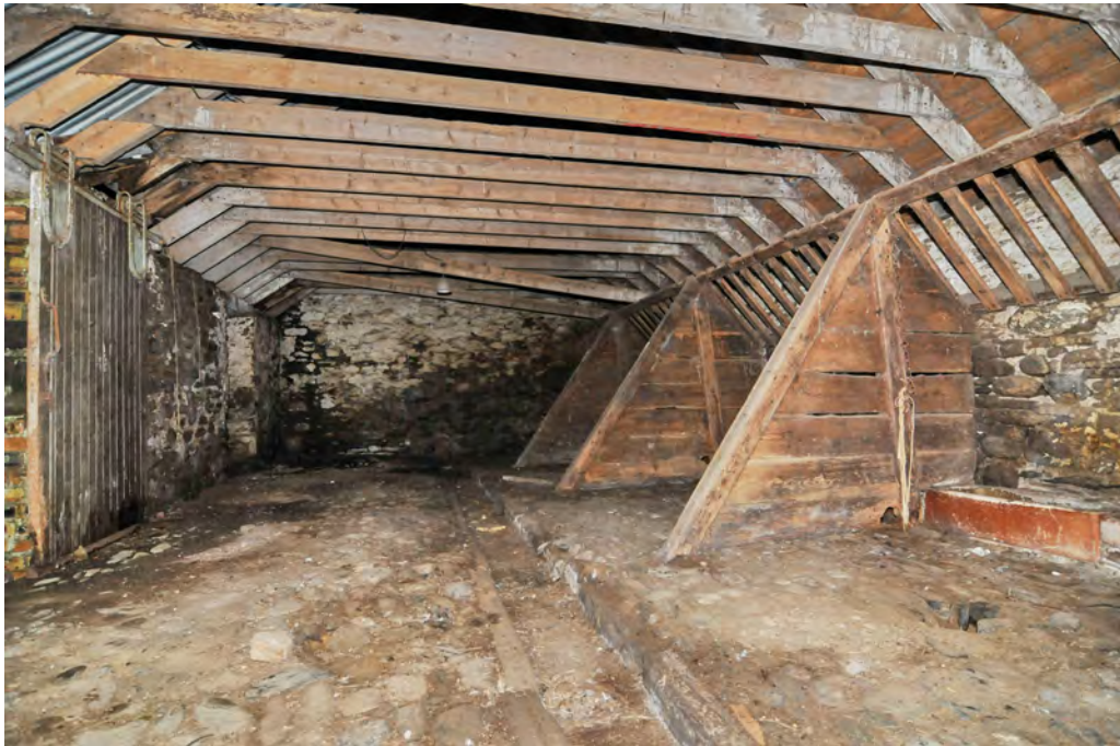
Fig. 22 - Unit 9, interior of the byre with feeding stalls, man
