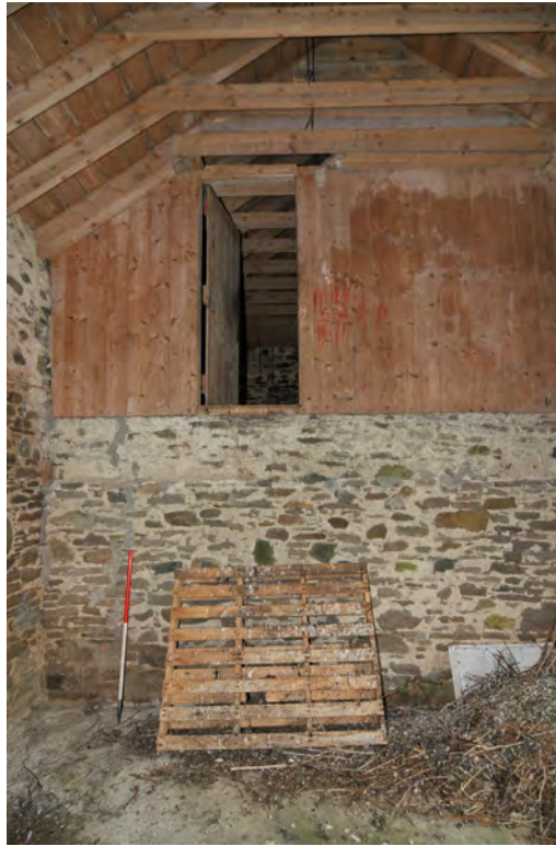
Fig. 19 - Unit 6, partition wall with an opening to the loft Unit 7
