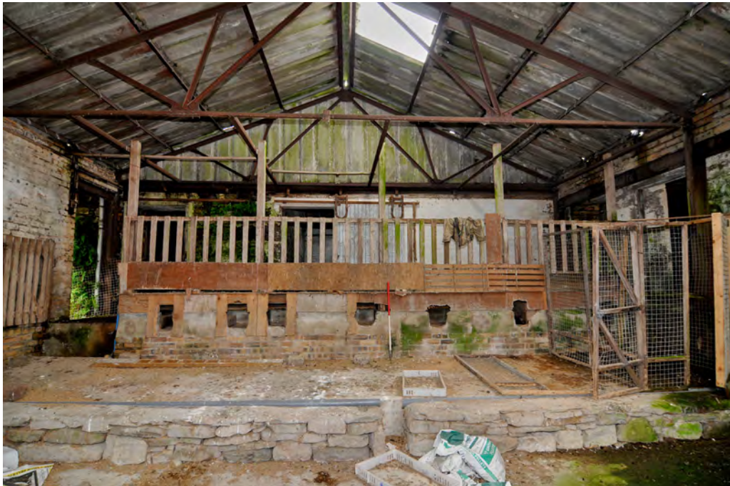
Fig. 24 - Unit 11, interior steel-framed roof and partitioning for cattle stalling
