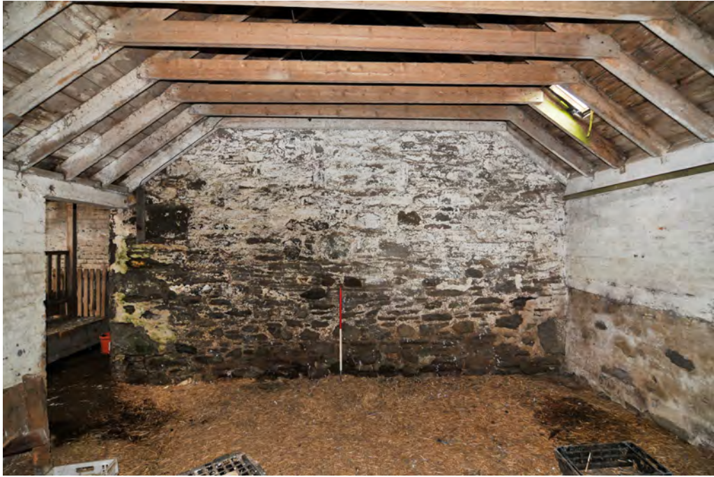
Fig. 23 - Unit 10, interior of the barn
