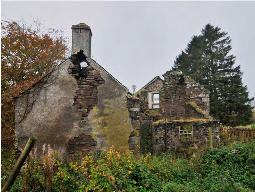
Fig. 7 - The NW rear elevation of the farmhouse with surviving chimney
