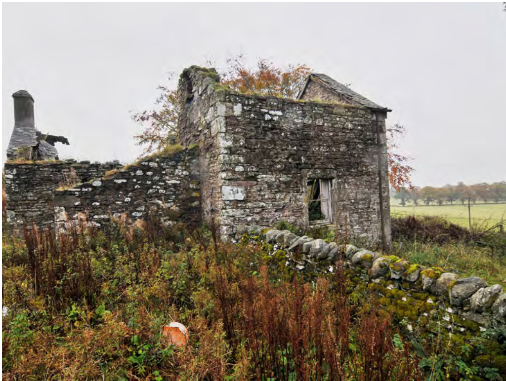
Fig. 6 - The SW side elevation of the farmhouse, fabric detail and ground
