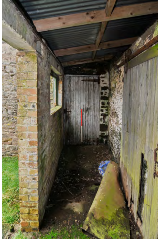
Fig. 25 - Unit 12 small modern brick-built lean-to general view
