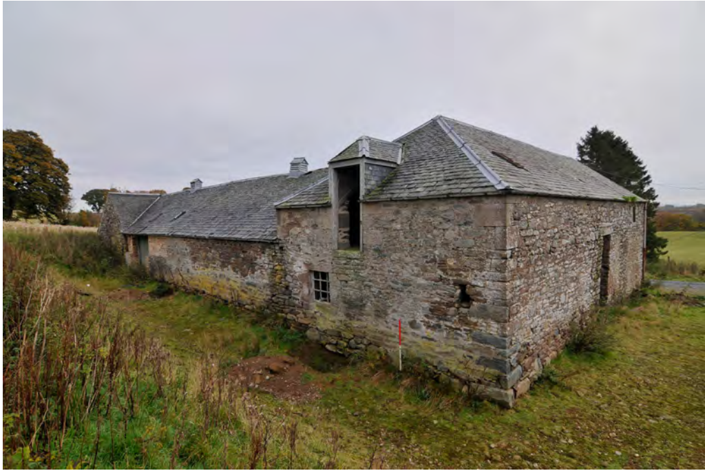
Fig. 15 - Steading exterior NW elevations with a pitching door at loft level
