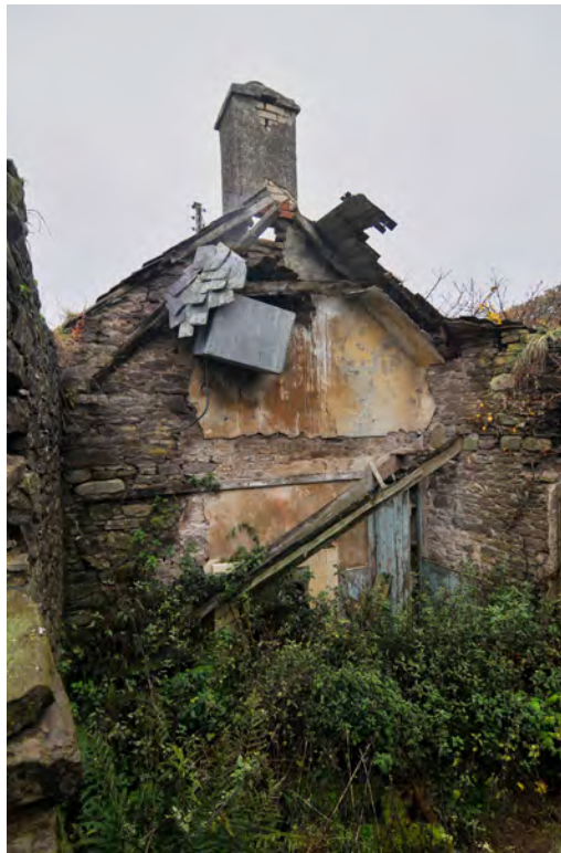
Fig. 10 - Unit 1 of the farmhouse, with plastered gable and rafter
