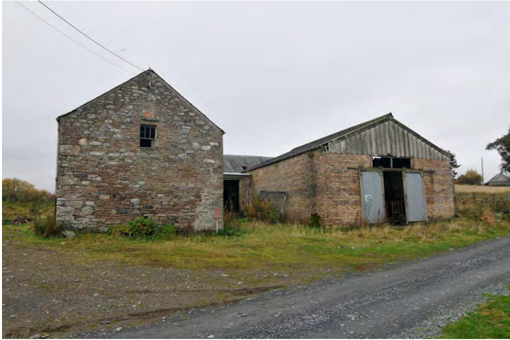
Fig. 13 - Steading exterior with a heightened pitched gable and later brick built shed
