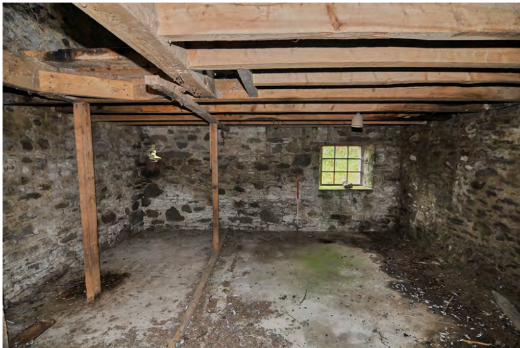
Fig. 20 - Unit 6, general interior view with loft joists and window
