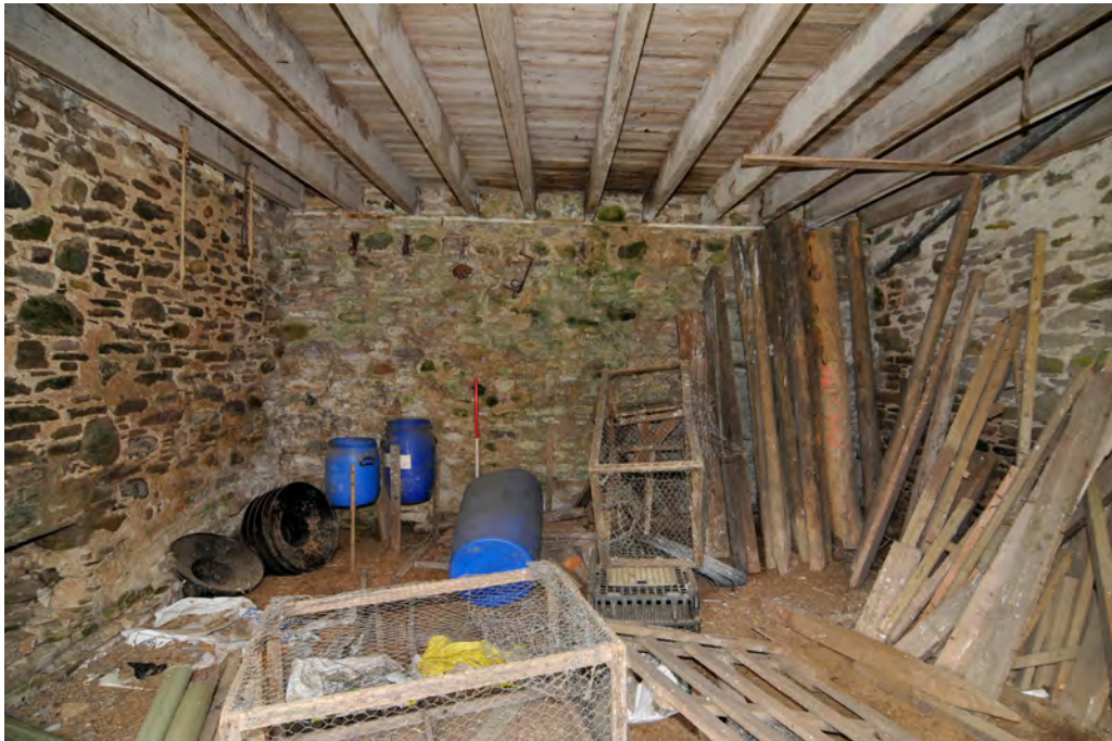
Fig. 18 - Unit 5, interior of the open shed
