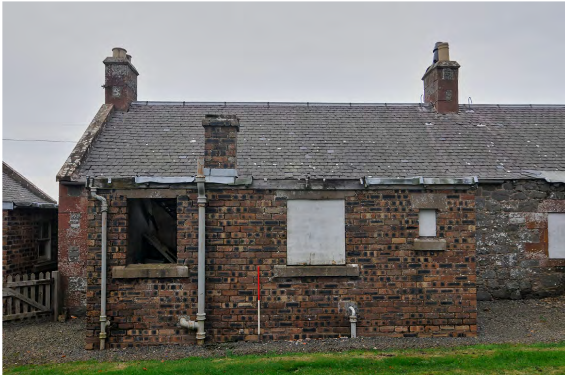
Fig. 15 - Building 2 Exterior west elevation with surviving washhouse chimney
