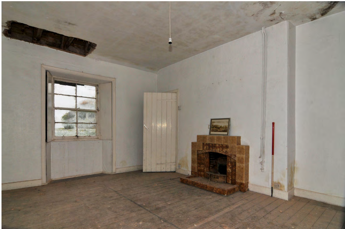
Fig. 24 - Building 3, Unit 36, living room with fireplace and single window
