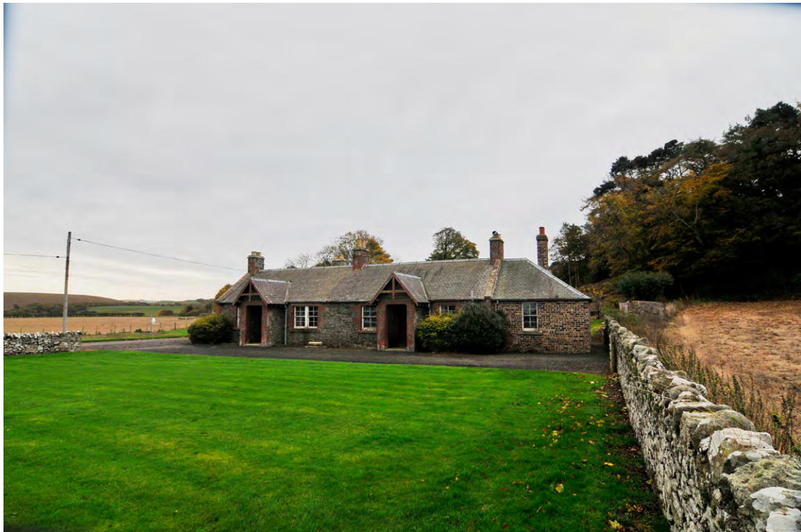
Fig. 6 - North elevation of Building 3
