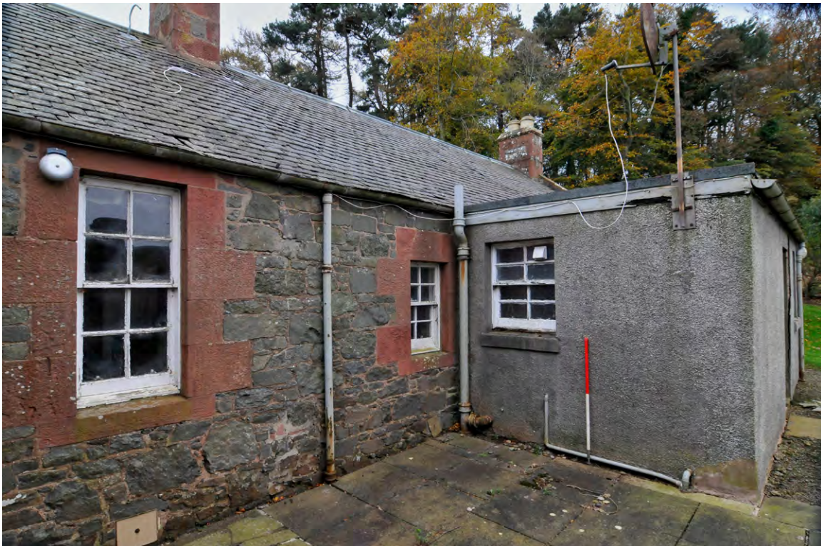
Fig. 10 - Building 1 north elevation, with rear extension
