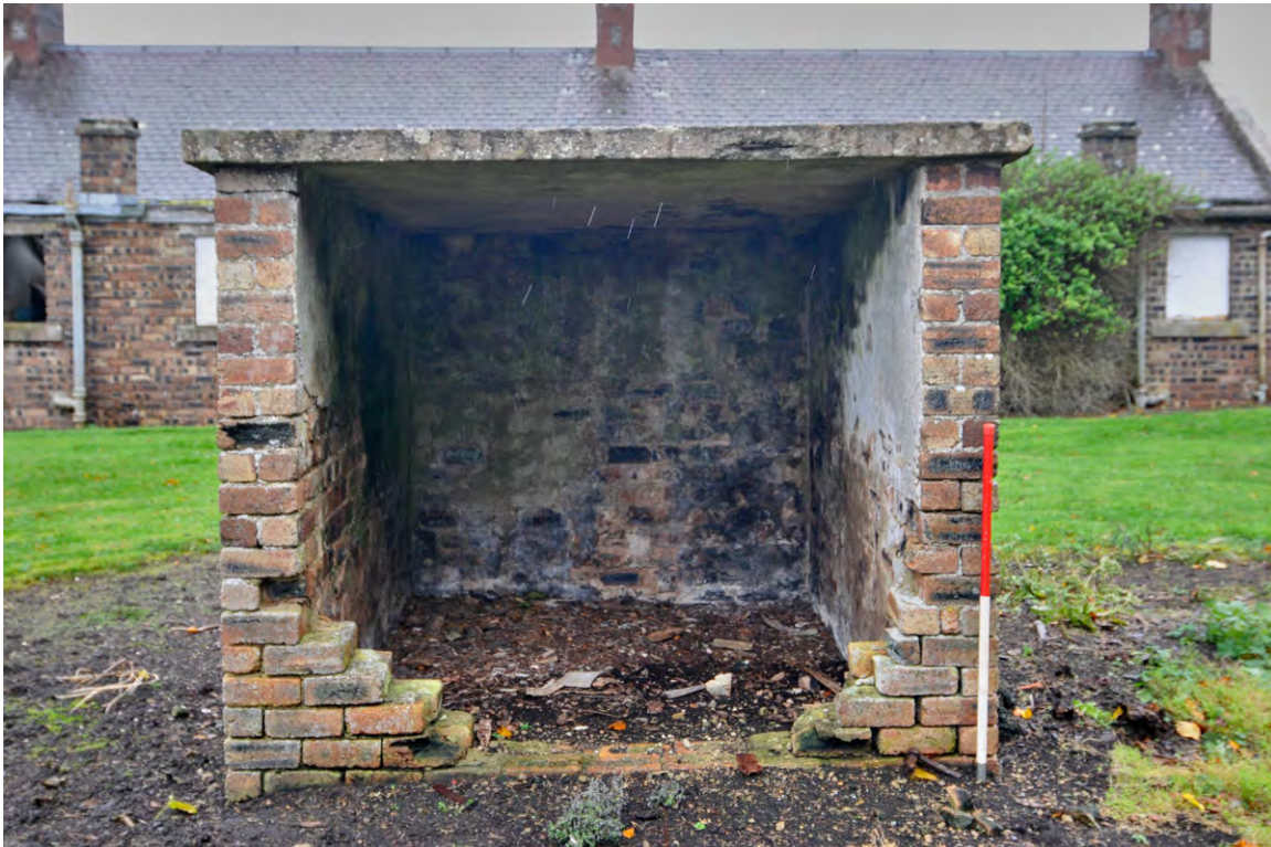
Fig. 31 - Detached building (Unit 46) general view of its west side
