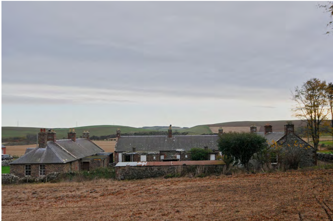
Fig. 7 - West elevations of Building 1-3 from a distance
