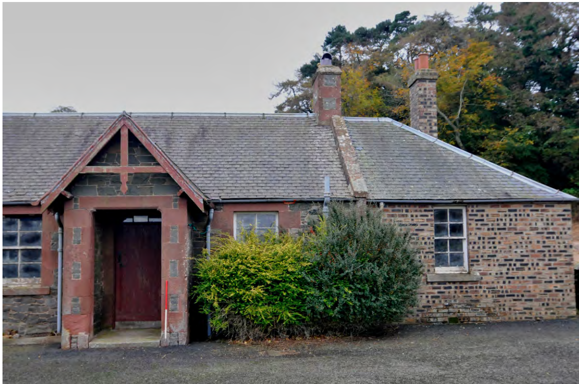
Fig. 20 - Building 3, Exterior north elevation with porch and brick-built extension
