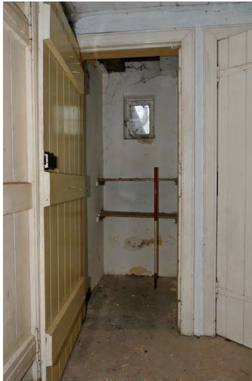
Fig. 29 - Building 3, Unit 44 cupboard
