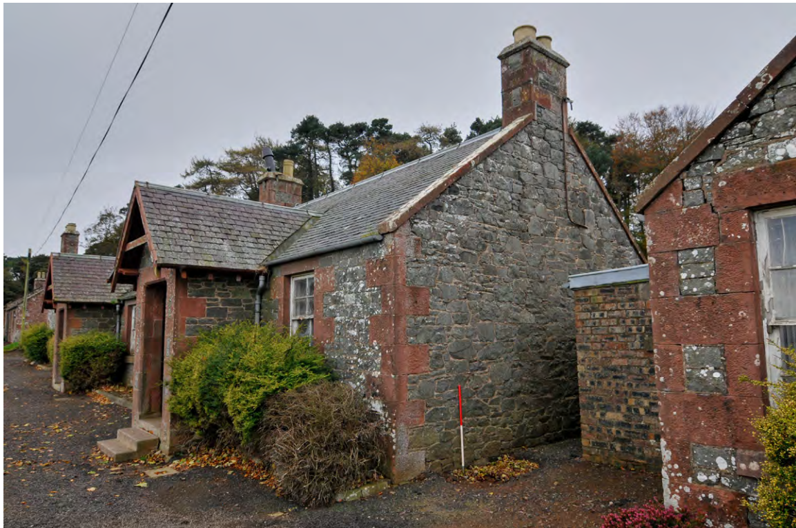
Fig. 14 - Building 2, Exterior east and north gable
