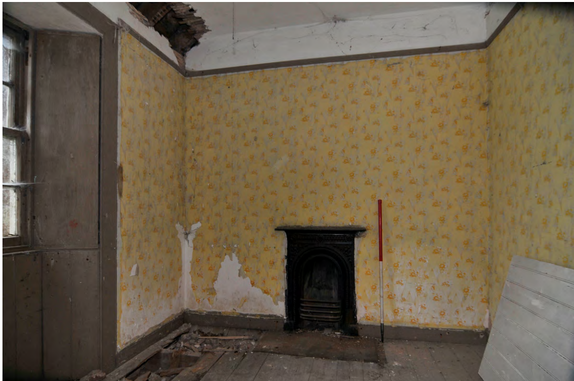
Fig. 16 - Building 2, Unit 14, bedroom with cast-iron fireplace and window shutter
