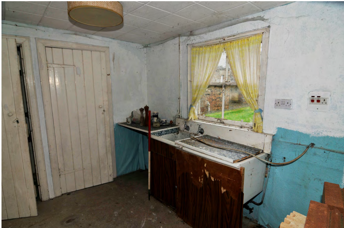
Fig. 28 - Building 3, Unit 43 kitchen with Belfast sink
