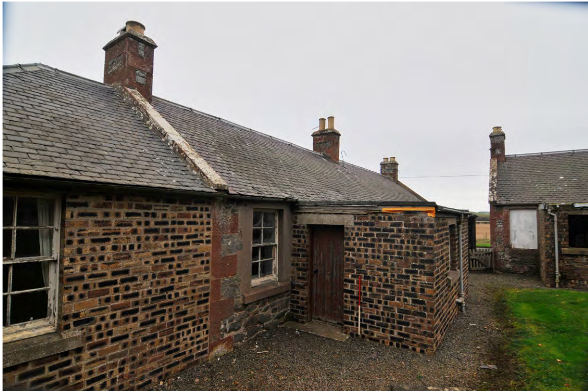
Fig. 21 - Building 3, Exterior south elevation with brick-built extensions
