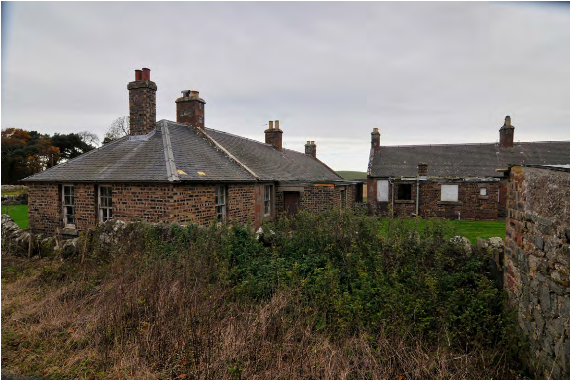
Fig. 9 - West elevation of Building 3 (gable), brick extension
