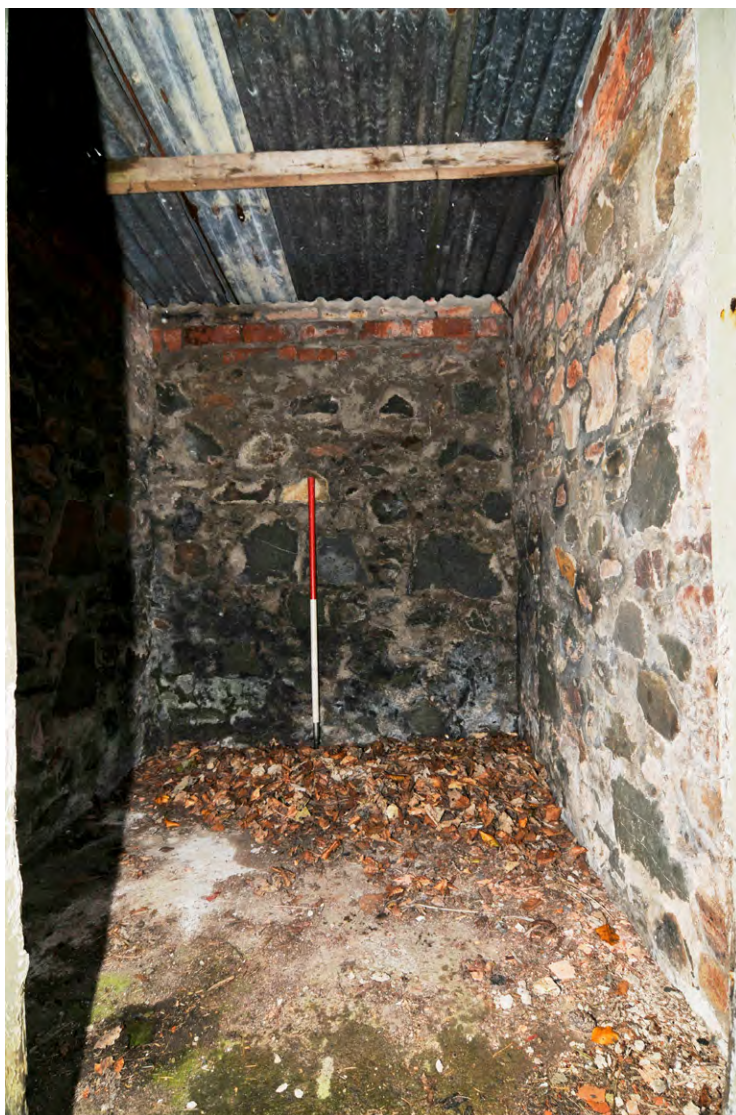
Fig. 33 - Interior of one of the sheds (Unit 27)
