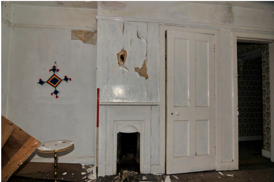
Fig. 26 - Building 3, Unit 41, bedroom with cast-iron fireplace
