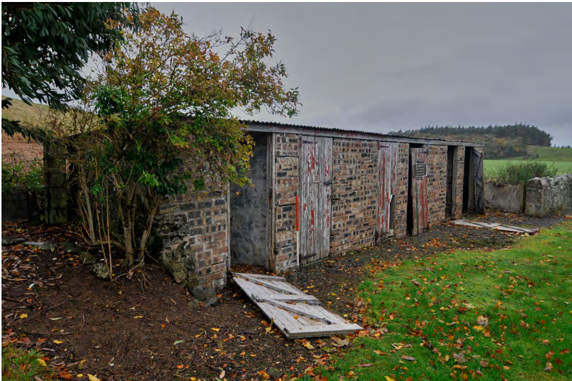
Fig. 32 - Row of sheds (Unit 47) on the west side of the cottages
