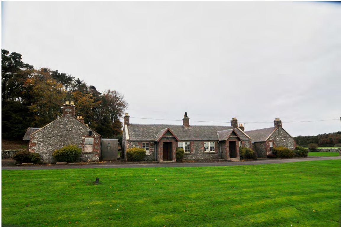
Fig. 5 - East elevations of Buildings 1-3
