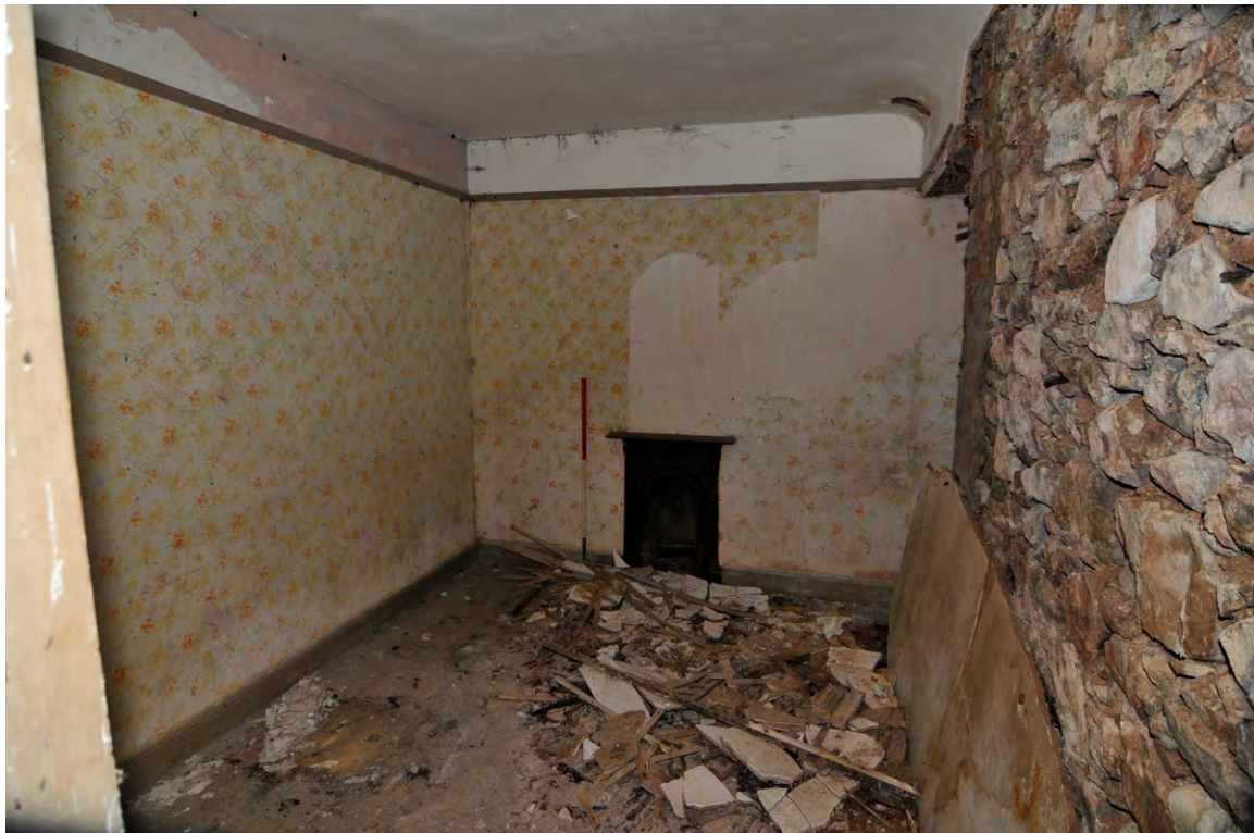
Fig. 18 - Building 2, Unit 18, bedroom with cast-iron fireplace and rubble gable wall
