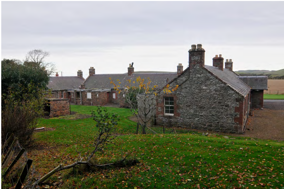
Fig. 8 - West elevation (gable) of building 1
