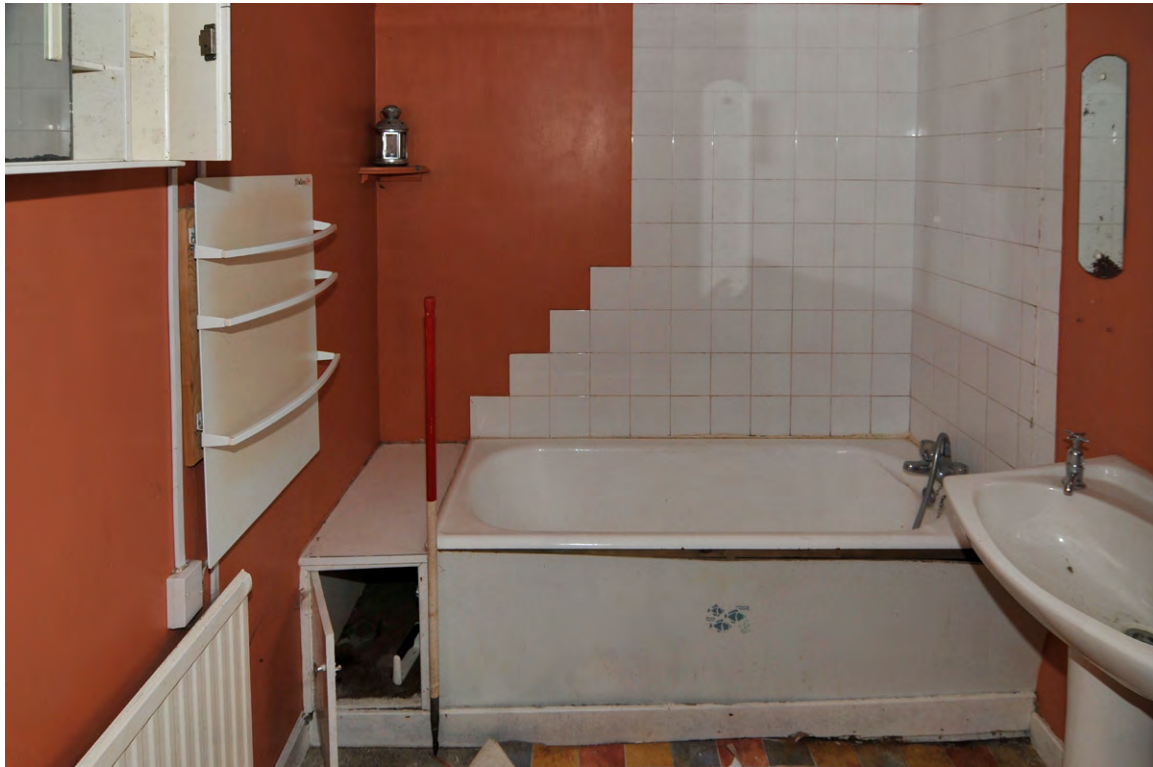
Fig. 13 - Building 1, Unit 11, bathroom
