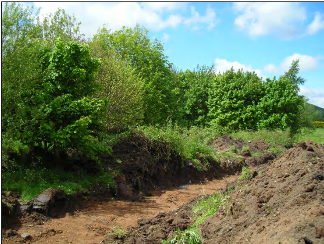
Fig 5 - General Site Photo from South East.
