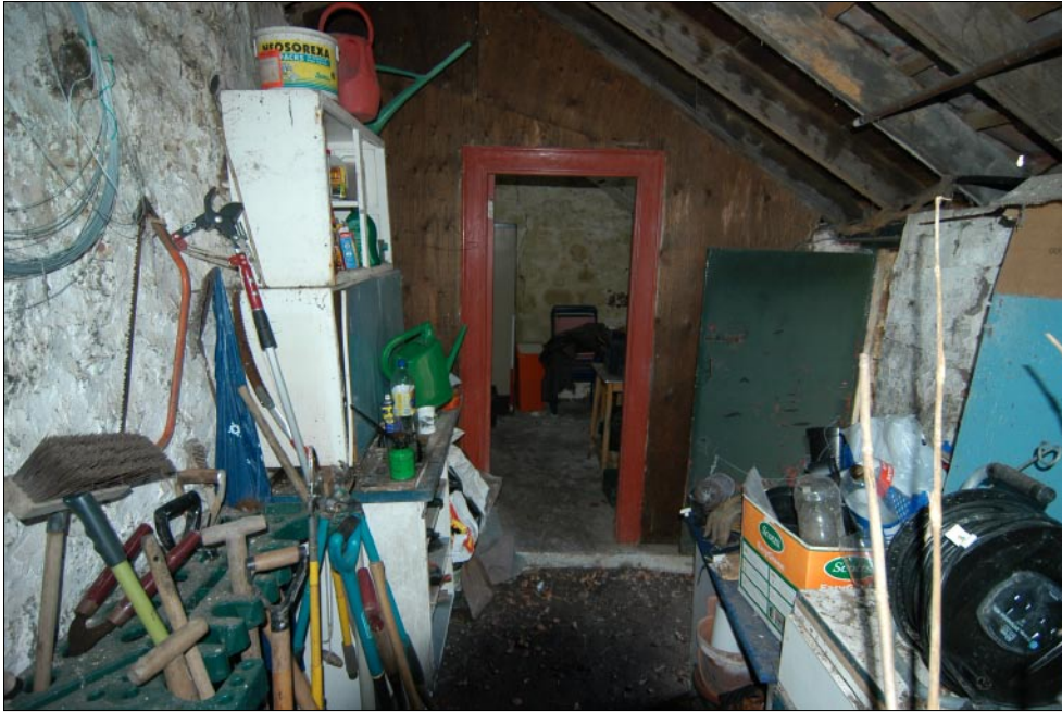
Fig. 22 - General shot of Potting shed western compartment interior from the west
