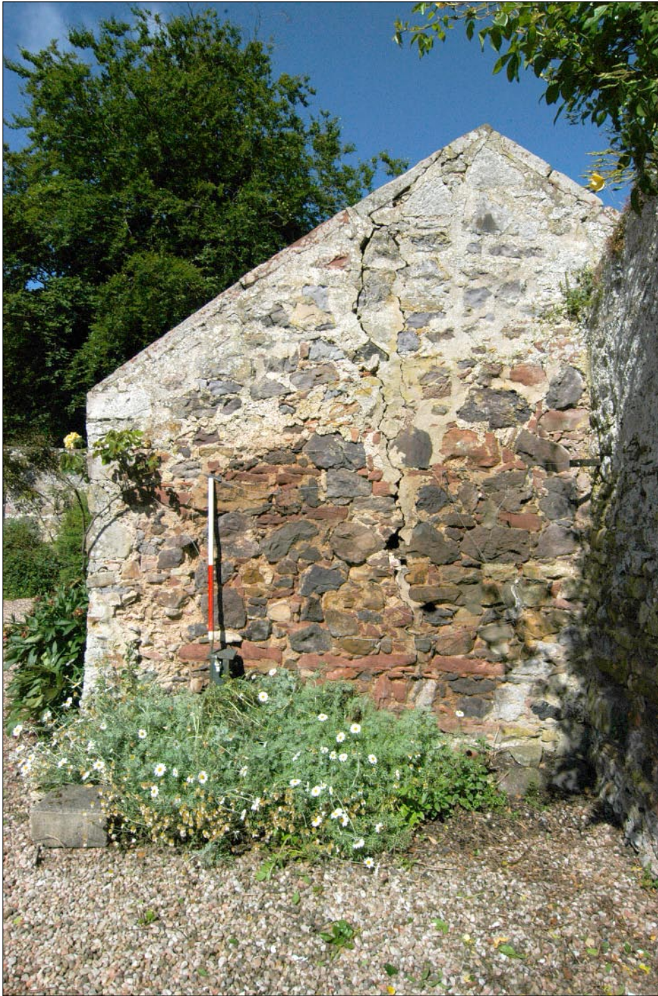
Fig. 18 - East facing elevation of Potting shed
