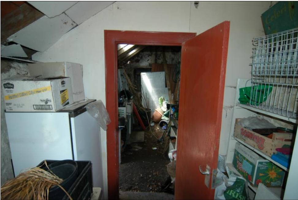
Fig. 23 - General shot of Potting shed eastern compartment interior from the east
