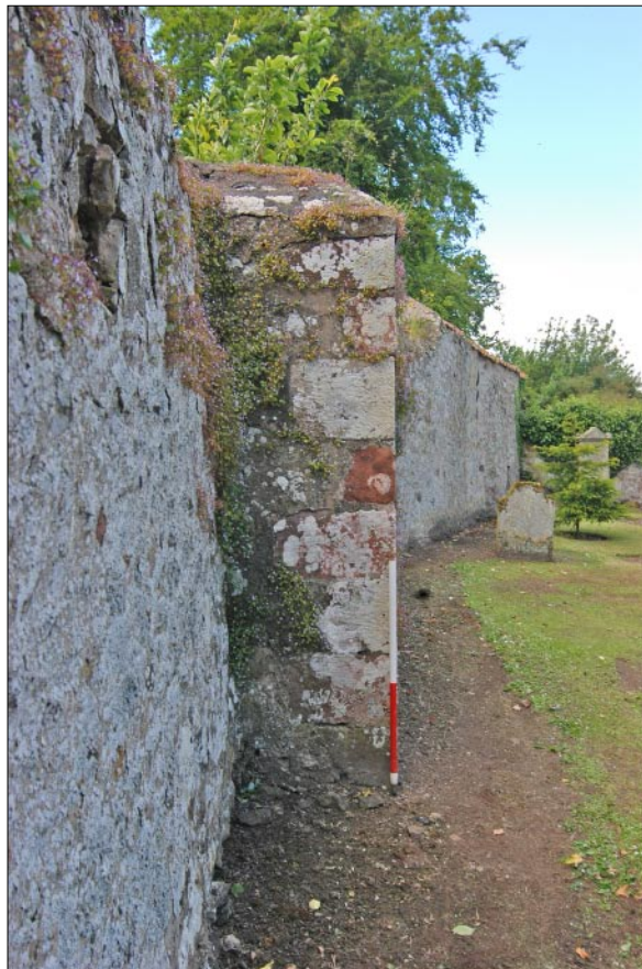
Fig. 33 - General shot of eastern quoins of north facing 'Manse' wall - from east
