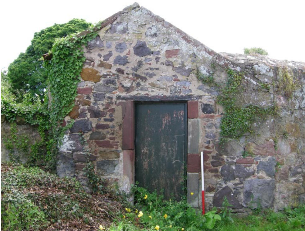
Fig. 17 - West facing elevation of Potting shed
