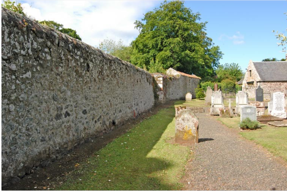
Fig. 34 - General shot of north facing Kirk Yard wall from north-east.
