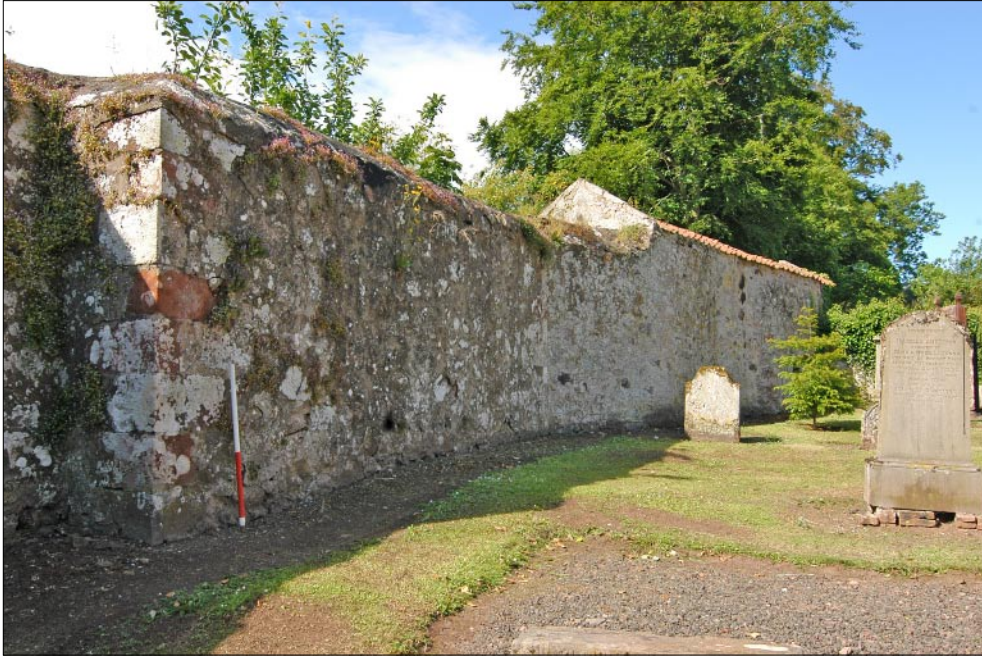
Fig. 32 - General shot of north facing 'Manse' wall - from north-east
