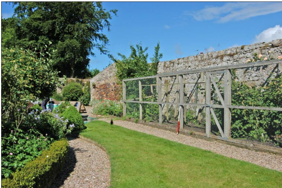
Fig. 29 - General shot of south facing garden wall - from south-east
