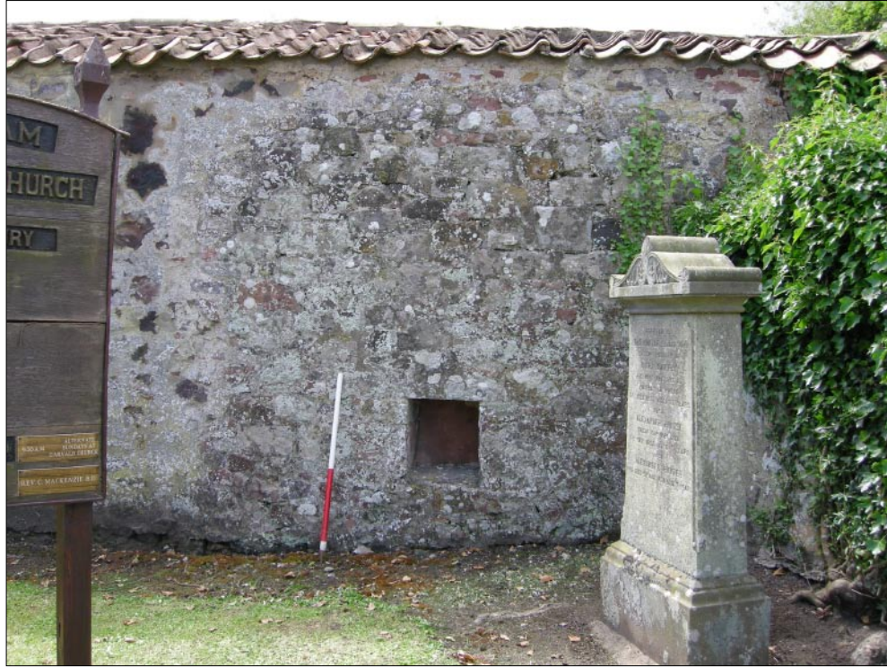
Fig. 21 - North facing elevation of Potting shed - close-up of feature
