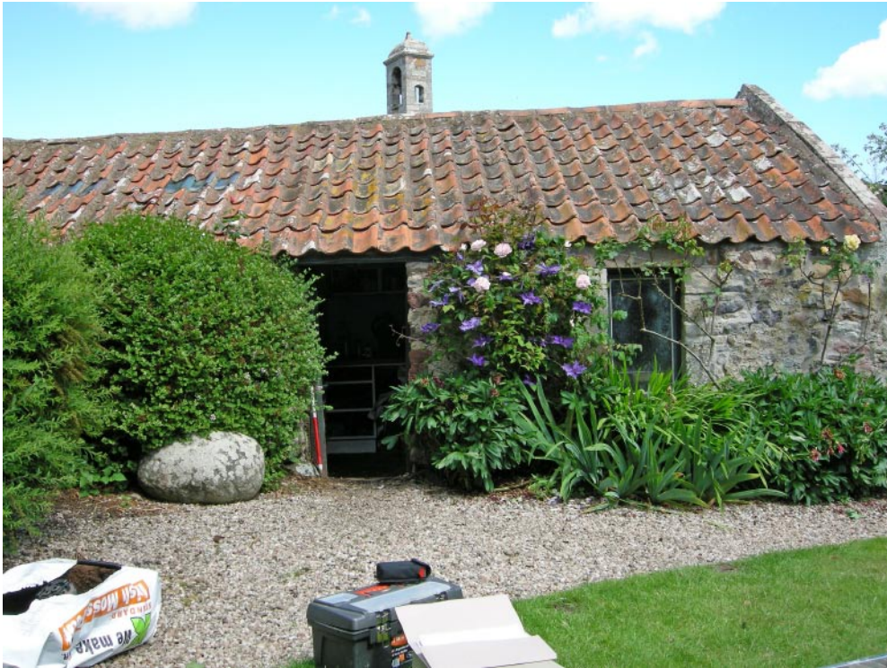
Fig. 16 - South facing elevation of Potting shed
