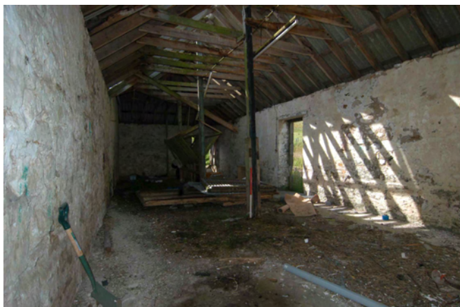
Plate 22 - Unit 11, from the south-east
