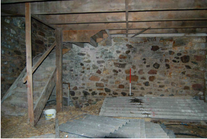
Plate 12 - Unit 3, west-facing elevation
