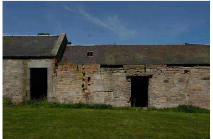
Plate 7 - Central Range, south-facing elevation
