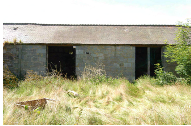
Plate 5 - West Range, east-facing elevation
