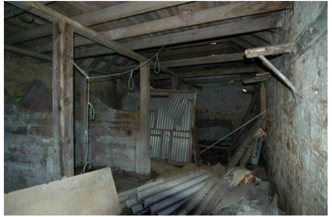
Plate 19 - Unit 9, from the south-east
