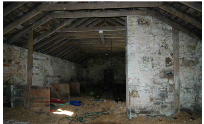
Plate 27 - Unit 18, from the west
