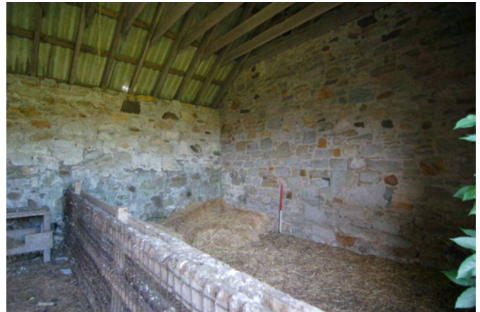
Plate 21 - Unit 10, north of partition, from the south-east
