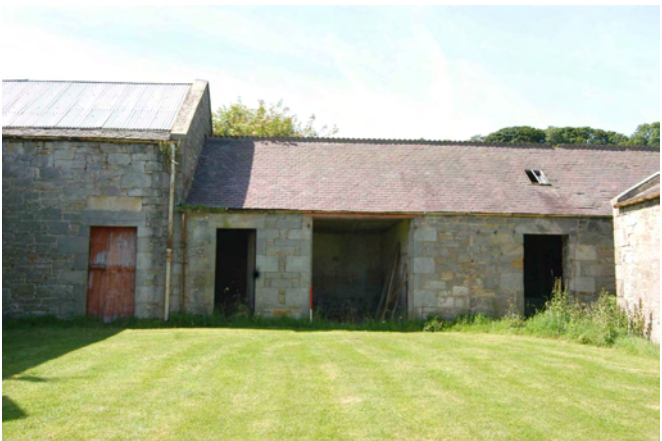
Plate 4 - West Range, east-facing elevation
