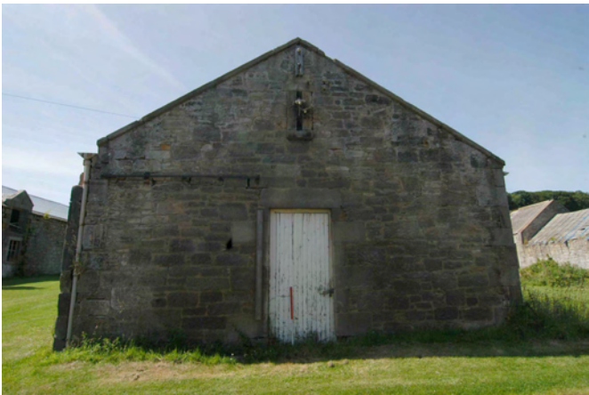
Plate 8 - Central Range, east-facing elevation
