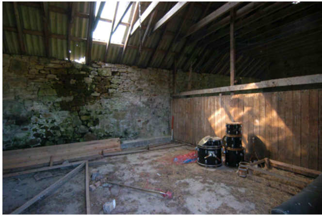
Plate 20 - Unit 10, south of partition, from the south-east
