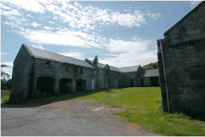
Plate 3 - South Range, north-facing, from the north-east
