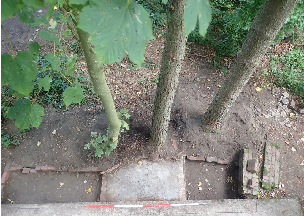
Fig: 6.23 Digital Ref: POWR_153 Direction: N Date: 01/09/2022 Description: Overhead shot of Doorstep 38.003
