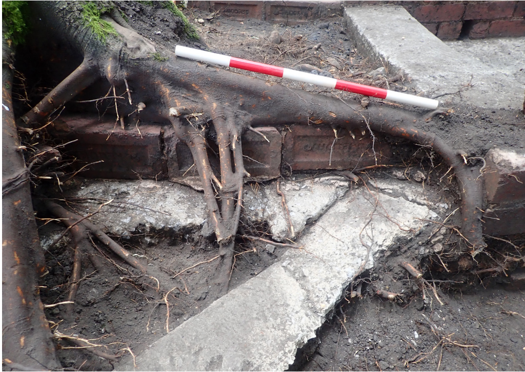
Fig: 6.25 Digital Ref: POWR_167 Direction: W Date: 01/09/2022 Description: Interaction between tree and Doorstep 38.005
