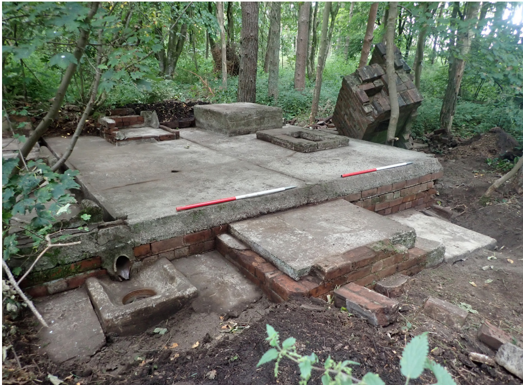
Fig. 6.38 Digital Ref: POWR_099 Direction: NW Date: 29/08/2022 Description: East facing elevation of Ablutions 54
