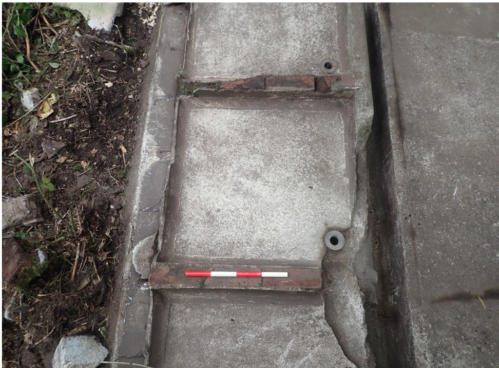
Fig: 6.43 Digital Ref: POWR_114 Direction: SW Date: 29/08/2022 Description: Cubicles 54.003
