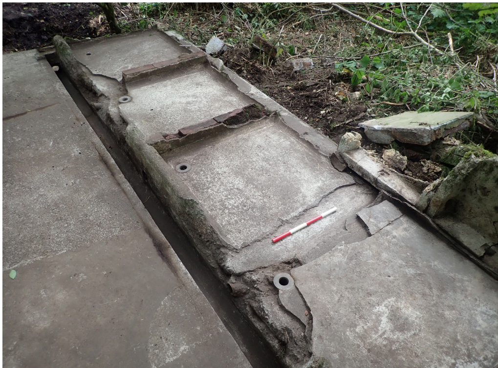
Fig: 6.40 Digital Ref: POWR_118 Direction: SE Date: 29/08/2022 Description: Cubicles 54.003
