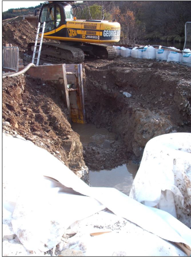
Fig. 2 - View of Trench after full excavation
