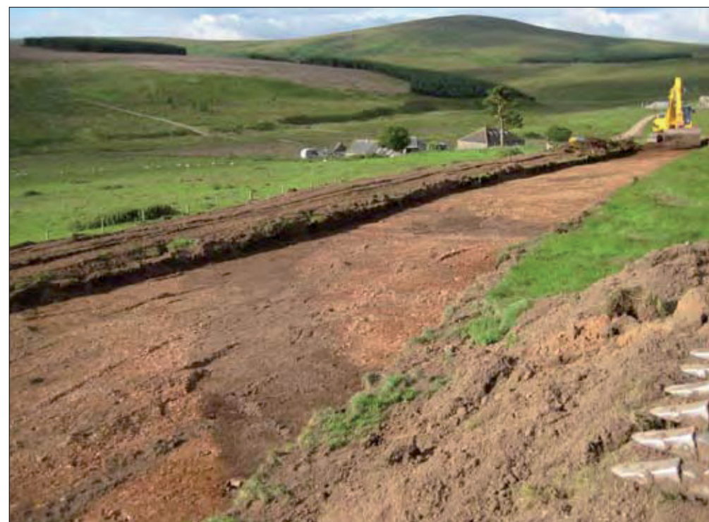
Fig 24. General shot of soil removal for access track to T12
