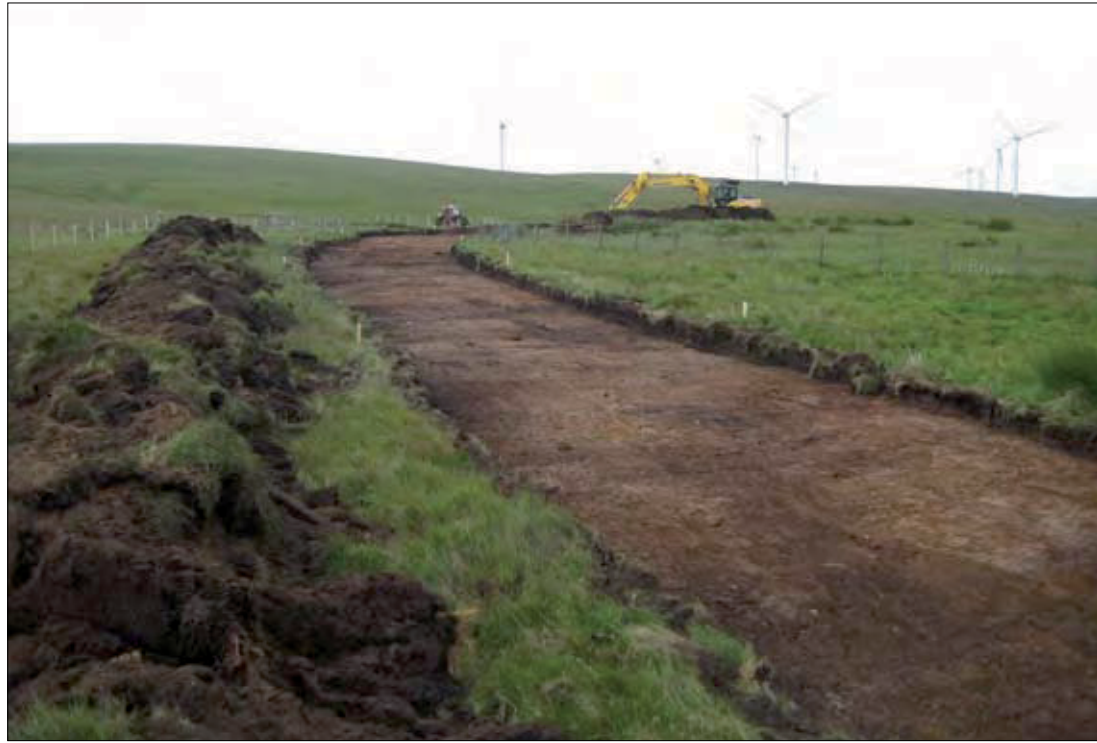
Fig. 48. Soil Removal at T2
