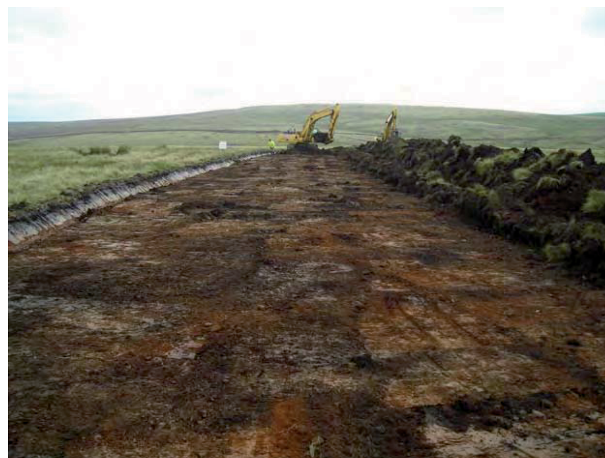
Fig 33. General view of topsoil removal at CFA Site 51, Herring Road
