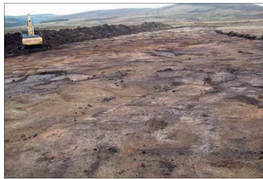
Fig. 51. Topsoil Removal at T58 Crane Pad
