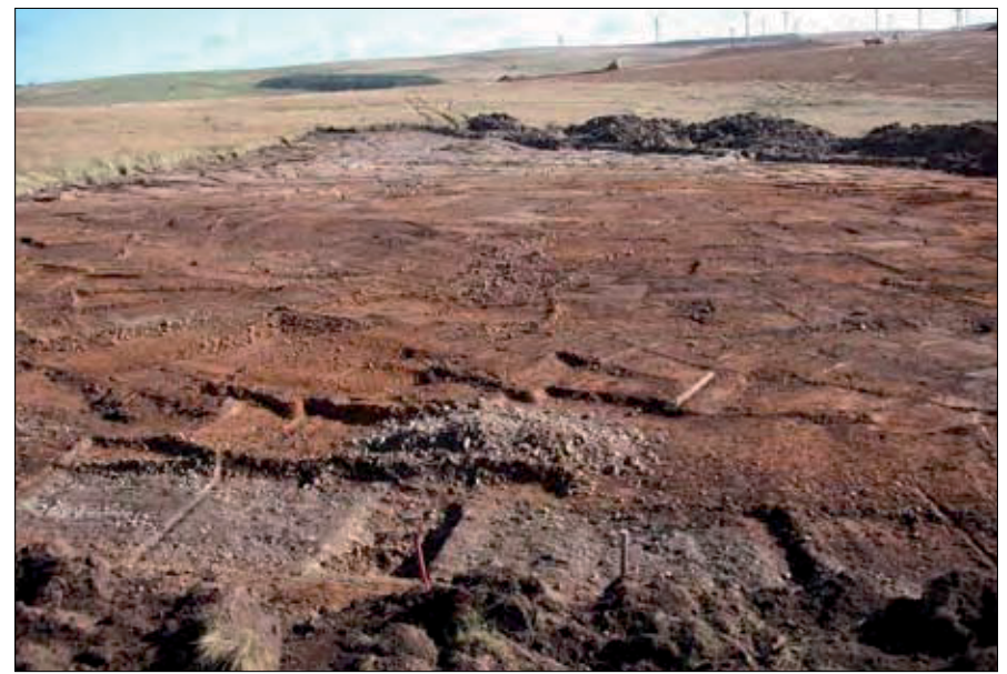
Fig. 50. E Facing Shot of T9 Crane Pad
