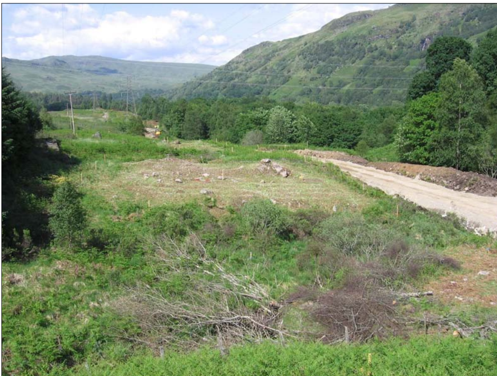
Fig. 6 - Site 5 from South following vegetation clearance
