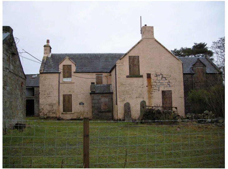
Fig 4b - Samsiston Farm House (Site 1), west-facing elevation
