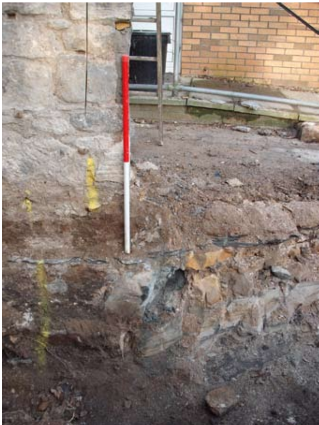
Fig 5 - Shot of fragmented sandstone foundations of demolished eastern annexe
