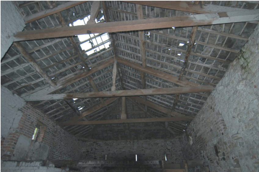
Plate 11 - General view of the A-frame roof structure
