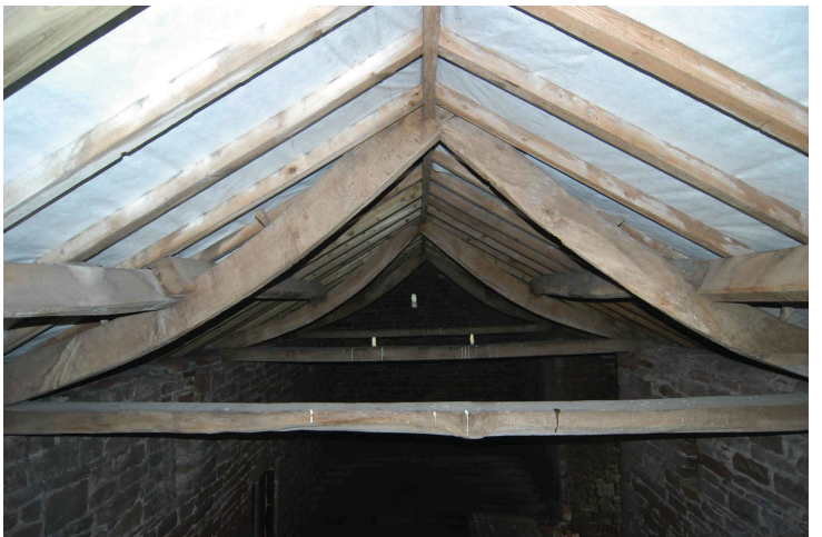
Plate 6 - A-frame cruck's, looking east
