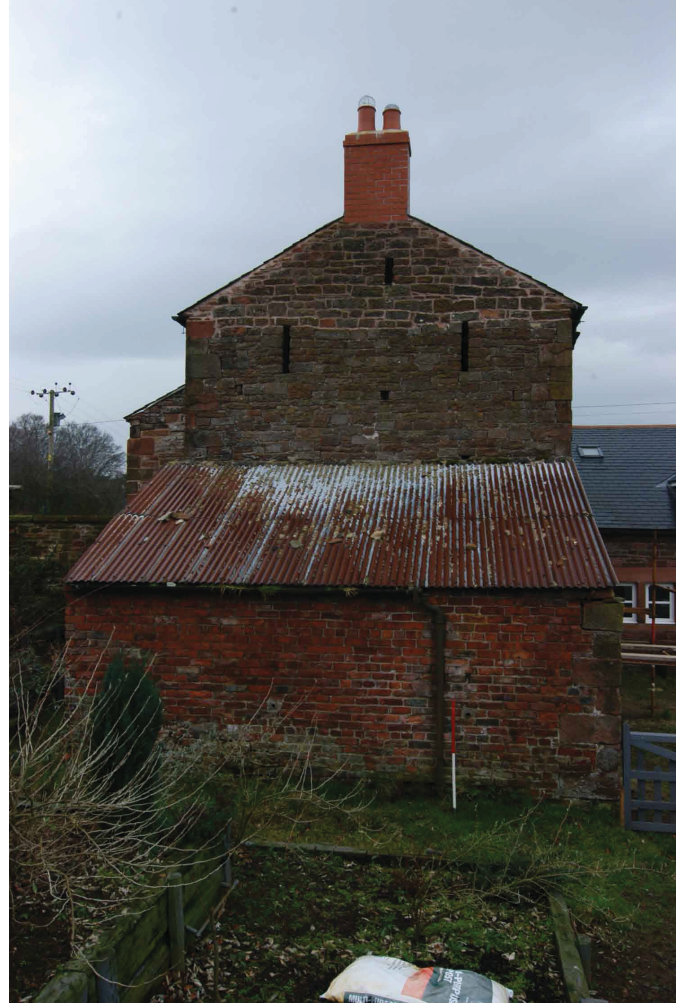
Plate 9 - East-facing gable with brick-built lean-to shed
