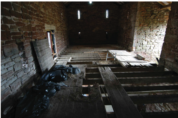
Plate 5 - Interior of the barn from the attic space
