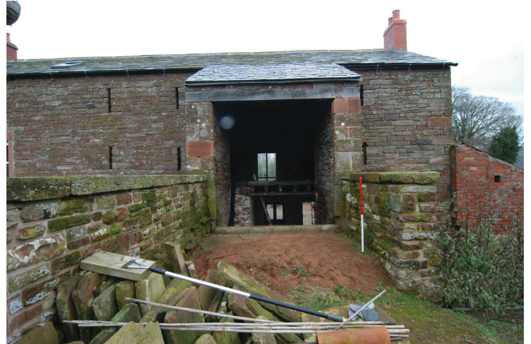
Plate 11 - South-facing elevation with large bay doorway
