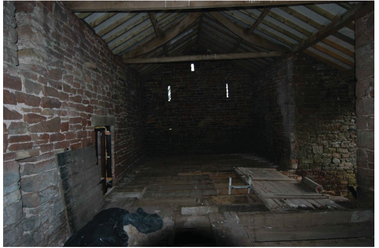
Plate 4 - Interior of the barn looking east
