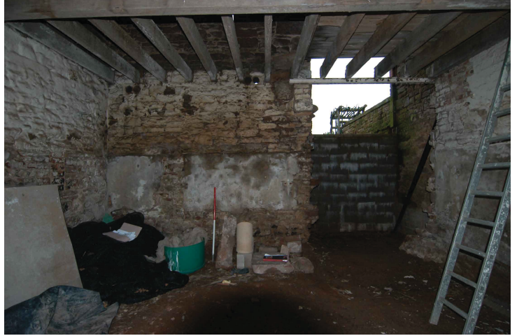
Plate 2 - Unit 2, former byre looking south
