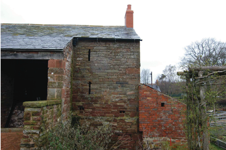
Plate 10 - South-facing elevation of the barn
