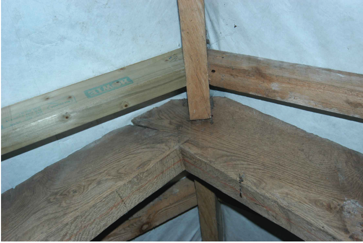
Plate 7 - Scarfe-joined cruck blades and new common rafters
