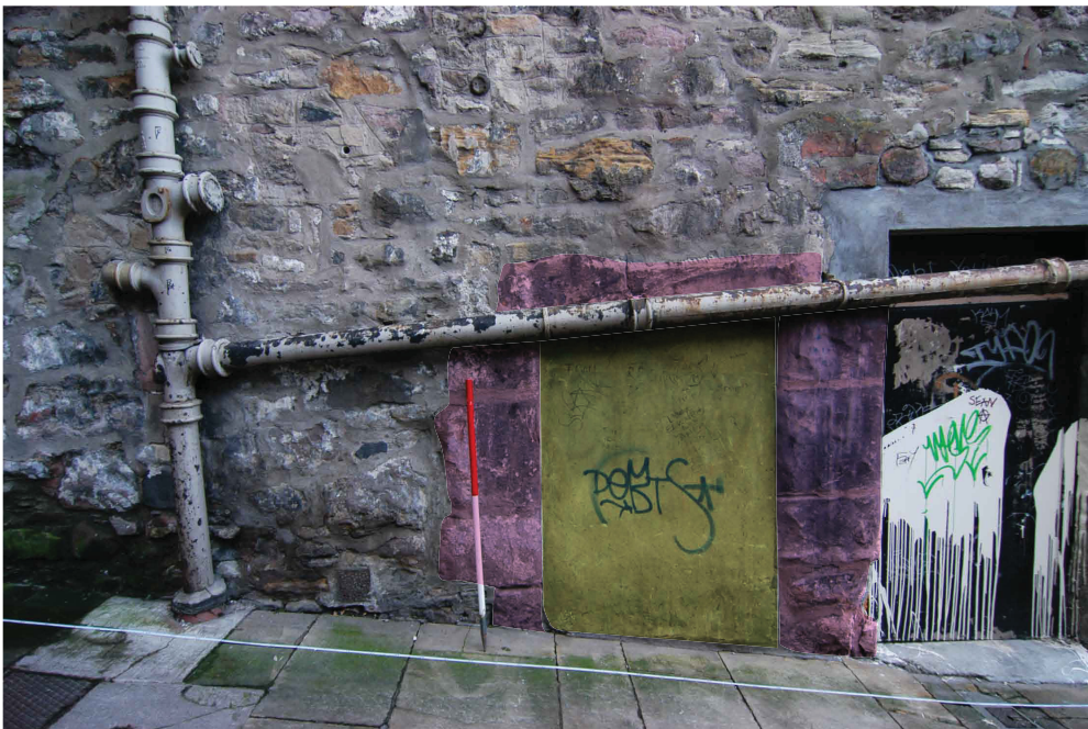
Plate 5 - North Gray's Close, blocked doorway
