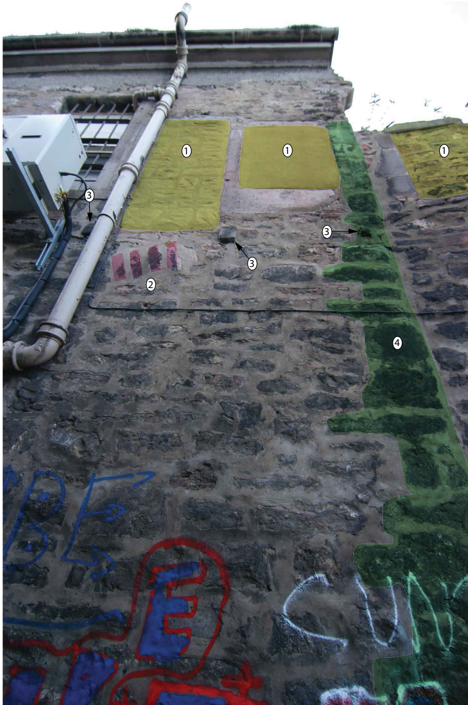
Plate 11 - Blocked features and others on North Gray's Close
