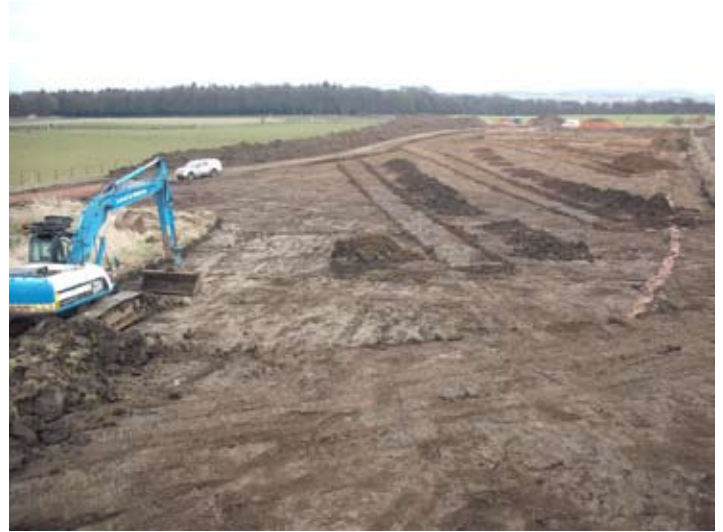
Fig. 11 - General shot of section 10 after monitored subsoil removal
