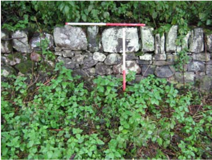
Fig. 16 - Pre-demolition shot of wall FB01
