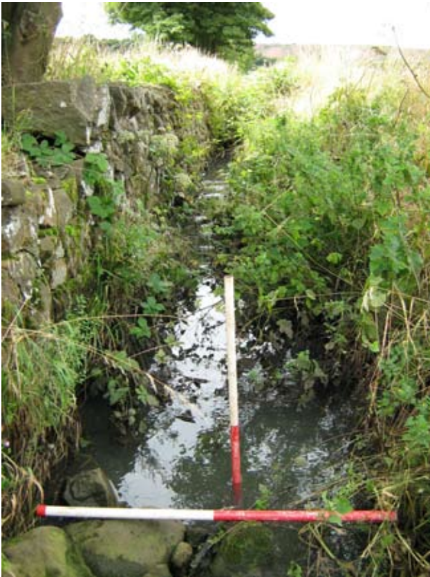
Fig. 22 - Pre-demolition shot of boundary FB05
