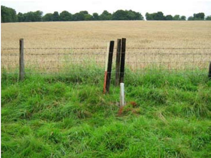
Fig. 18 - Pre-demolition shot of bank/fence FB03
