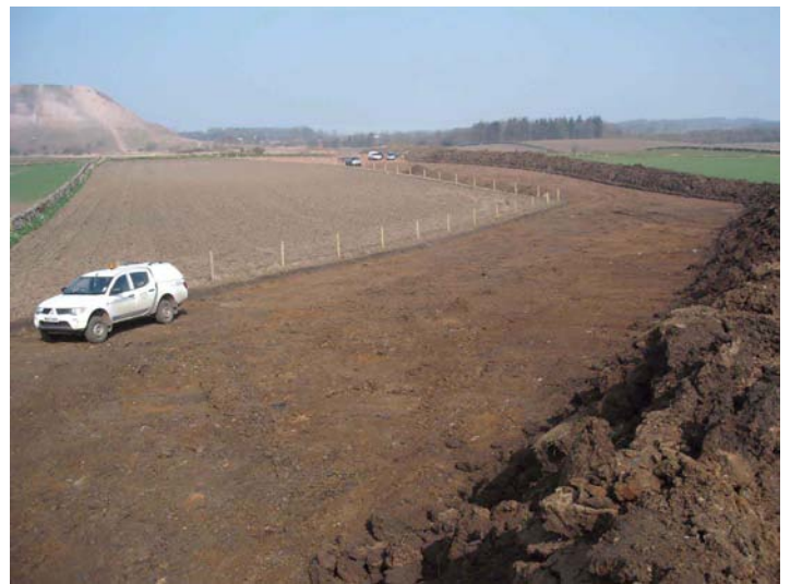
Fig. 9 - General shot of section 9 after topsoil removal
