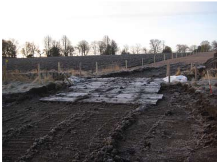
Fig. 25 - Completed access point across the top of the flume pipe and boundary wall FB05
