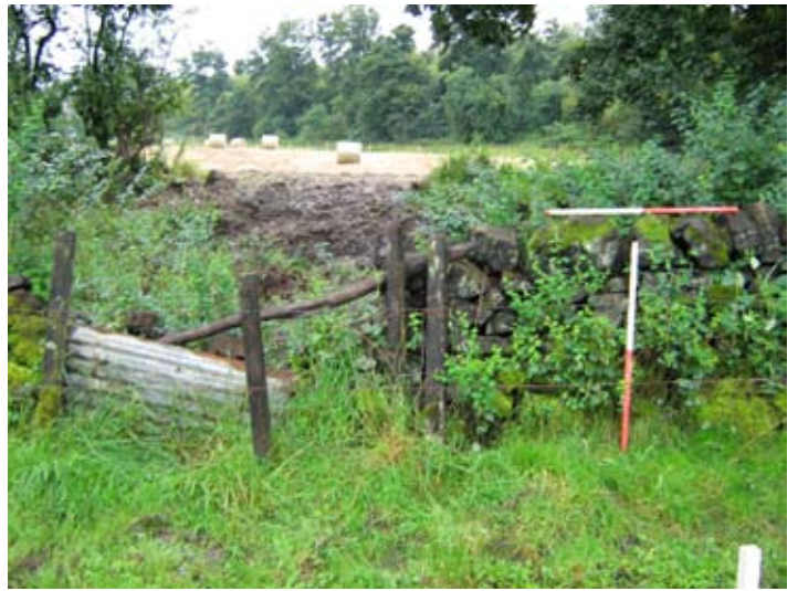
Fig. 17 - Pre-demolition shot of wall FB02
