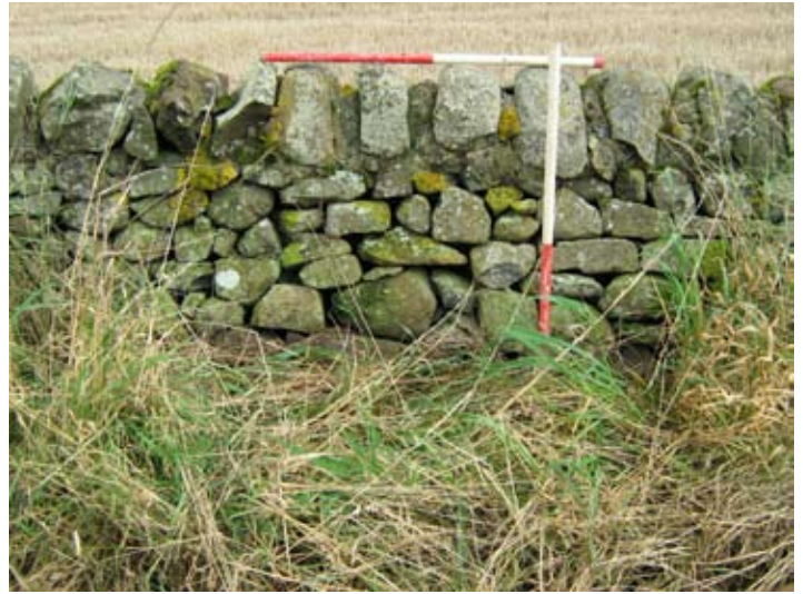
Fig. 19 - Pre-demolition shot of wall FB04
