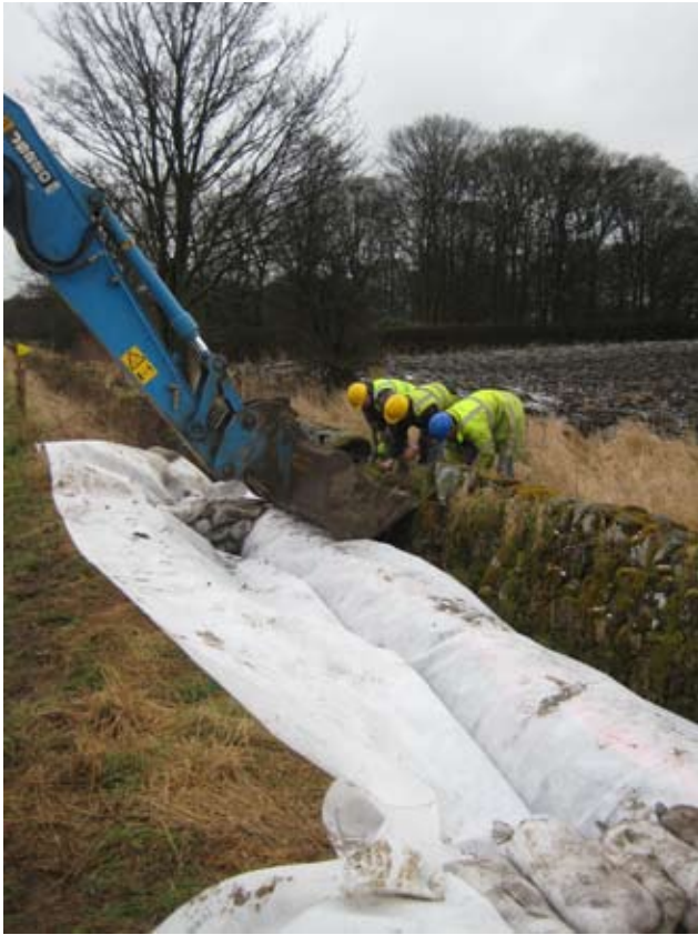
Fig. 24 - Flume pipe in place within ditch and demolition of upper courses of boundary wall FB05 in progress
