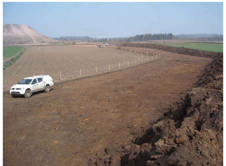
Fig. 9 - General shot of section 9 after topsoil removal
