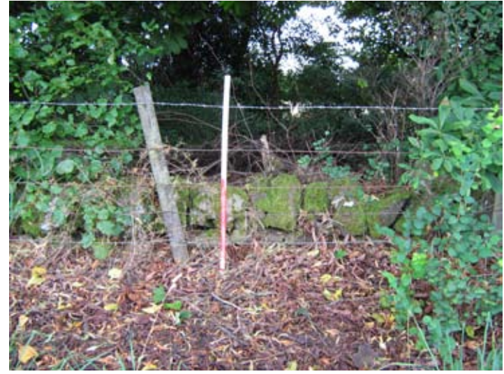
Fig. 21 - Pre-demolition shot of wall FB06
