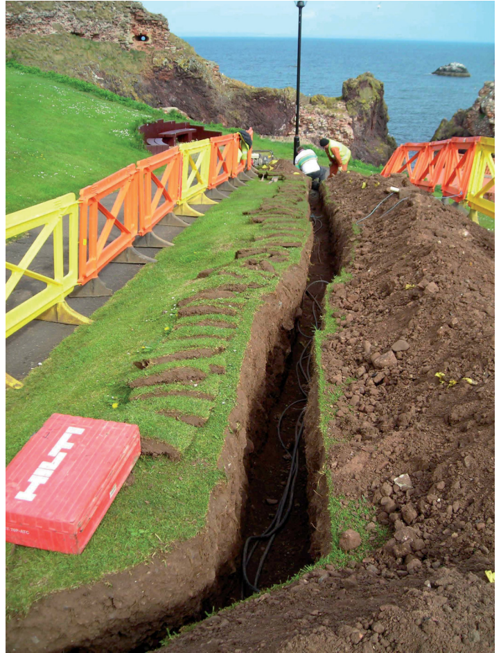
Fig.3 - General shot of Trench 2 facing North
