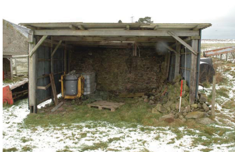
South-facing Elevation of Building 2
