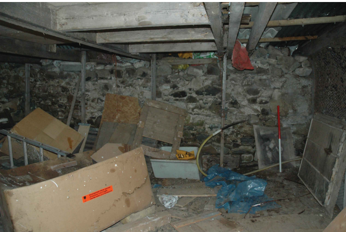
Plate 3 - Building 2 interior shot of Unit 2, animal house
