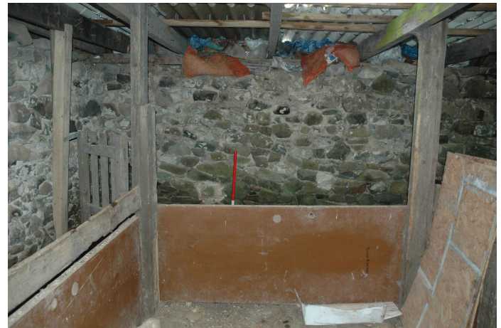
Plate 4 - Building 2 interior shot of Unit 2, animal pens
