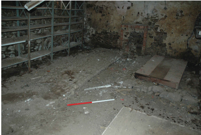
Plate 7 - Building 3 interior shot of Unit 1, central drain on the byre floor
