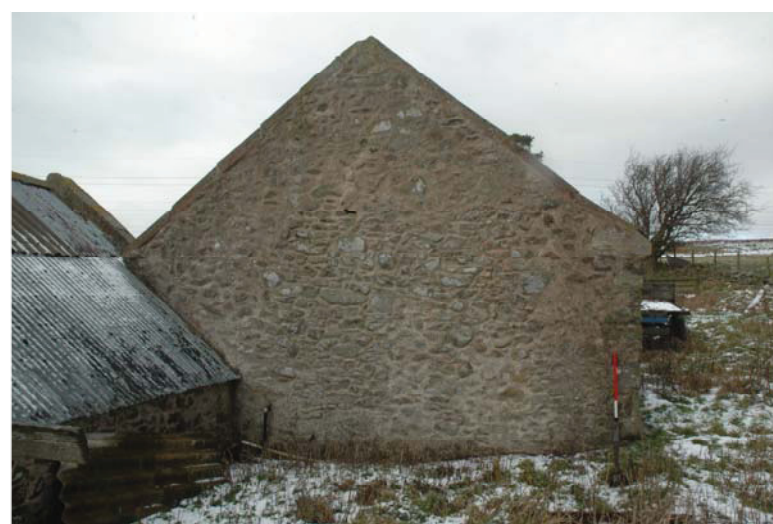
South-facing Gable of Building 3
