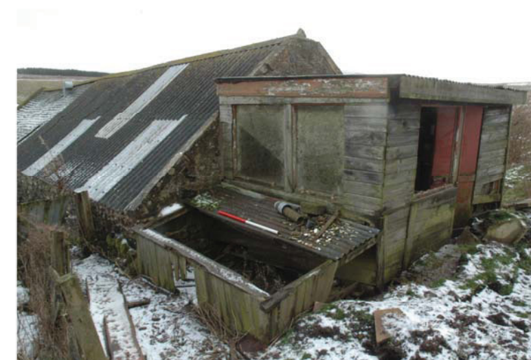
North-facing Gable & Shed of Building 3
