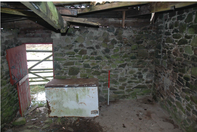
Plate 5 - Building 2 interior shot of Unit 4, animal house
