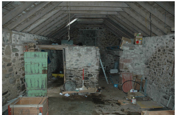
Plate 2 - Building 1 interior shot of the south end, of Unit 2, loft
