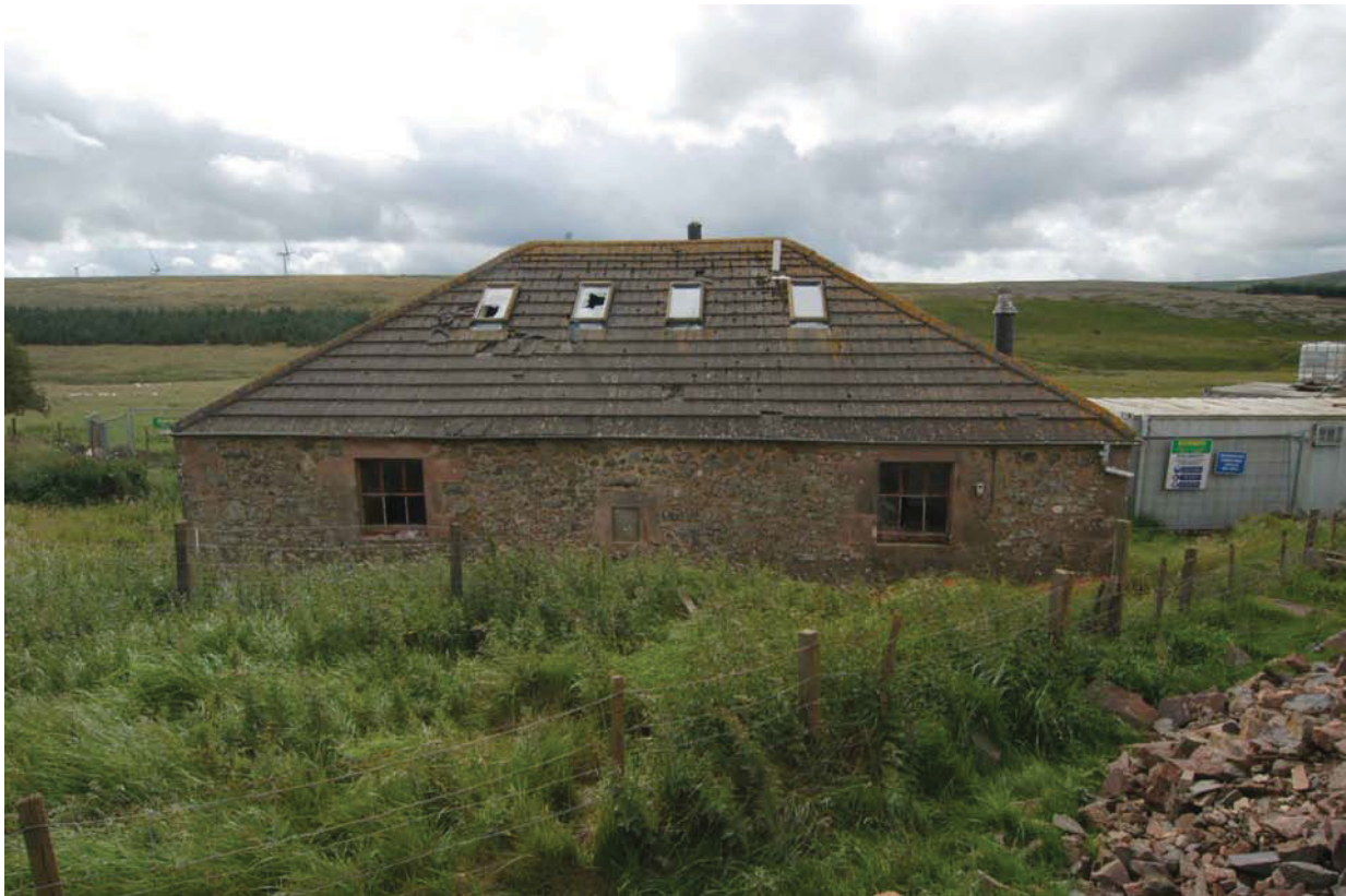
Plate 1 - General view of the cottage from the north
