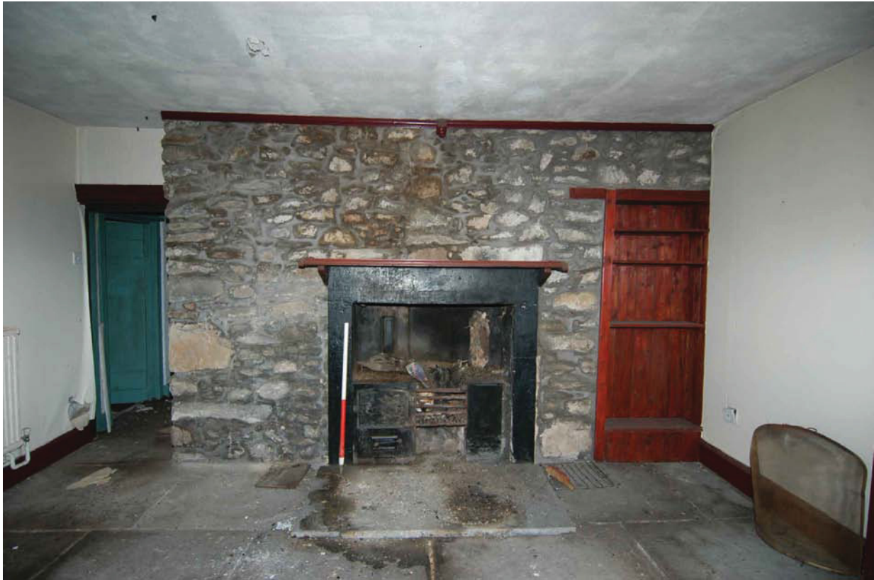
Plate 3 - Room 1 living room range, formerly the kitchen
