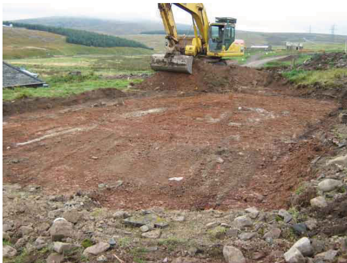
Fig. 4 General shot of building footprint after foundation removal, from N
