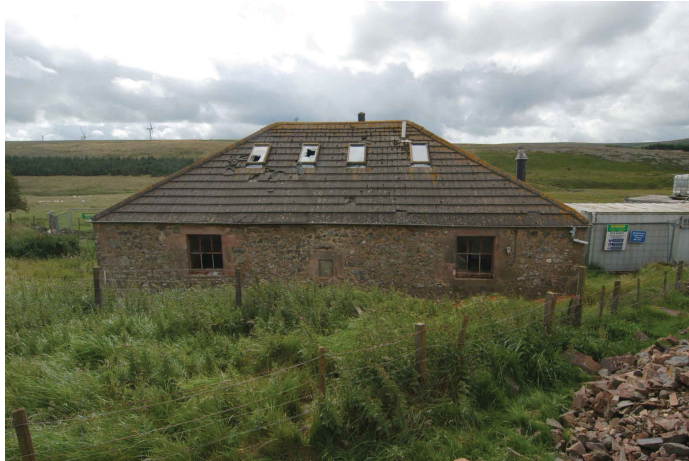
Fig. 2 General view of cottage prior to demolition, from N
