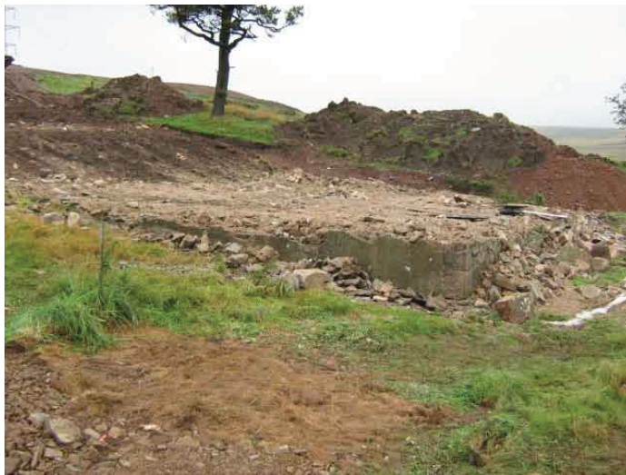
Fig. 3 Building foundations prior to removal, from S
