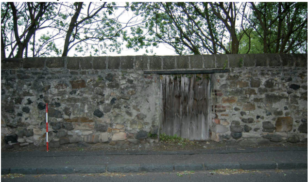
Plate 4 - Blocked openings 3 and 4 on the south-facing elevation
