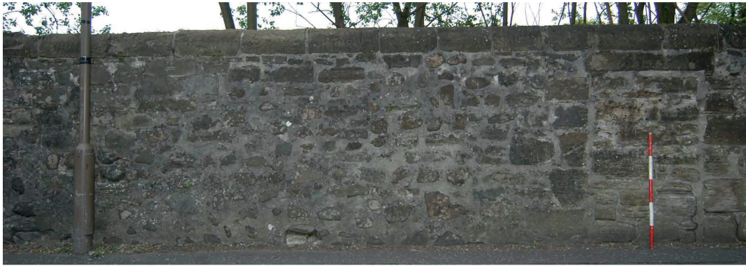
Plate 5 - Blocked openings 4 and 5 on the south-facing elevation
