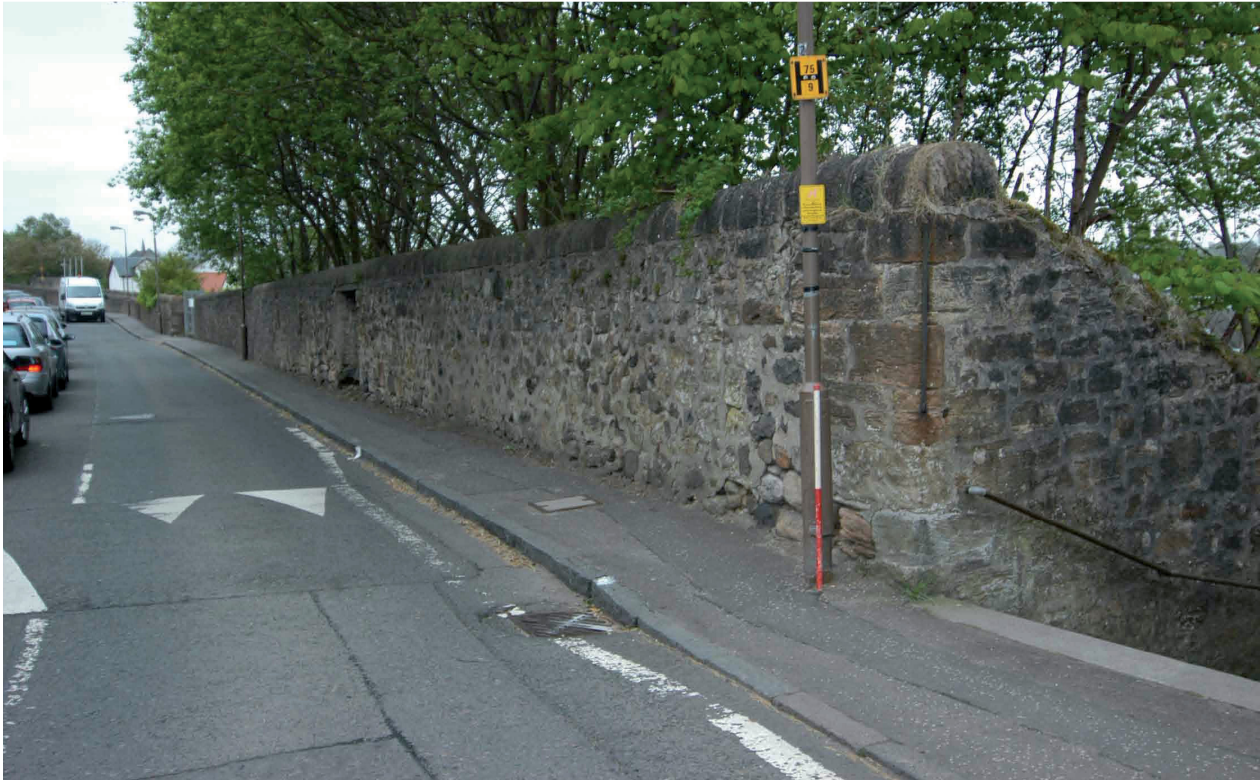
Plate 1 - General view of the south-facing elevation at Avon Place, looking east
