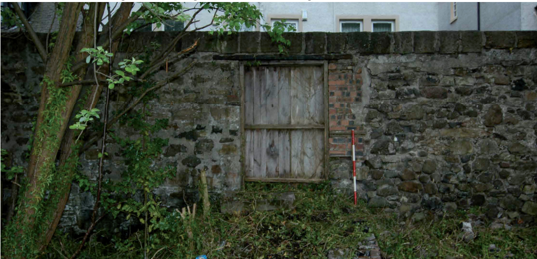
Plate 7 - North-facing elevation, blocked opening 3, general shot
