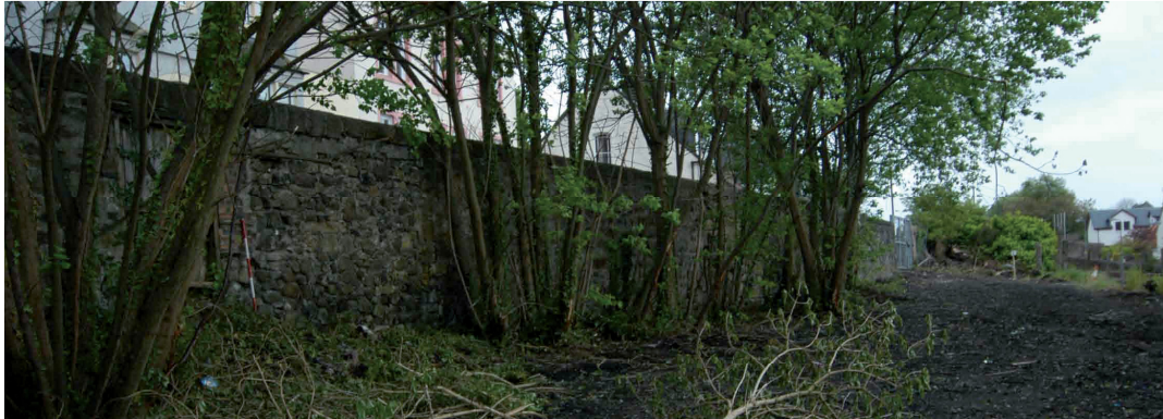
Plate 6 - North-facing elevation, general view looking east
