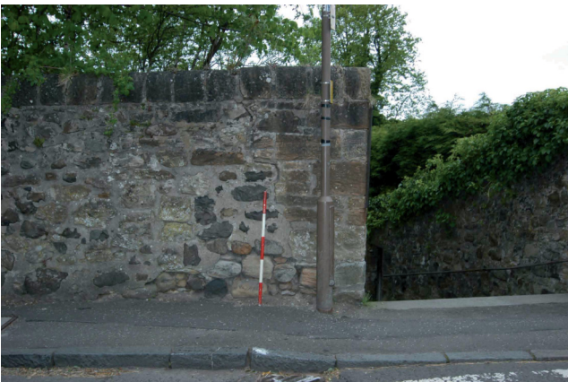
Plate 2 - Section of ashlar re-build associated with the railway underpass
