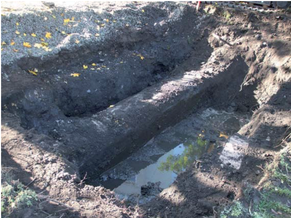
Figure 2 - View of CSO chamber excavation
