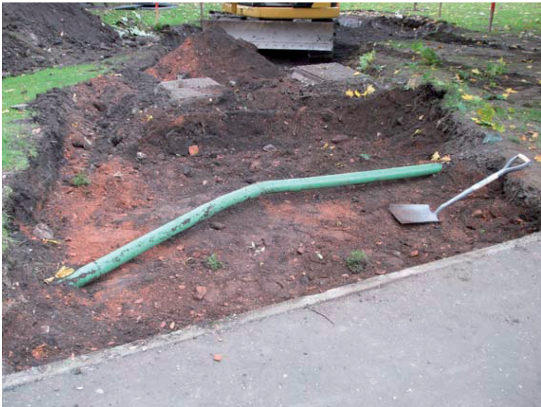
Figure 3 - View of access track excavation
