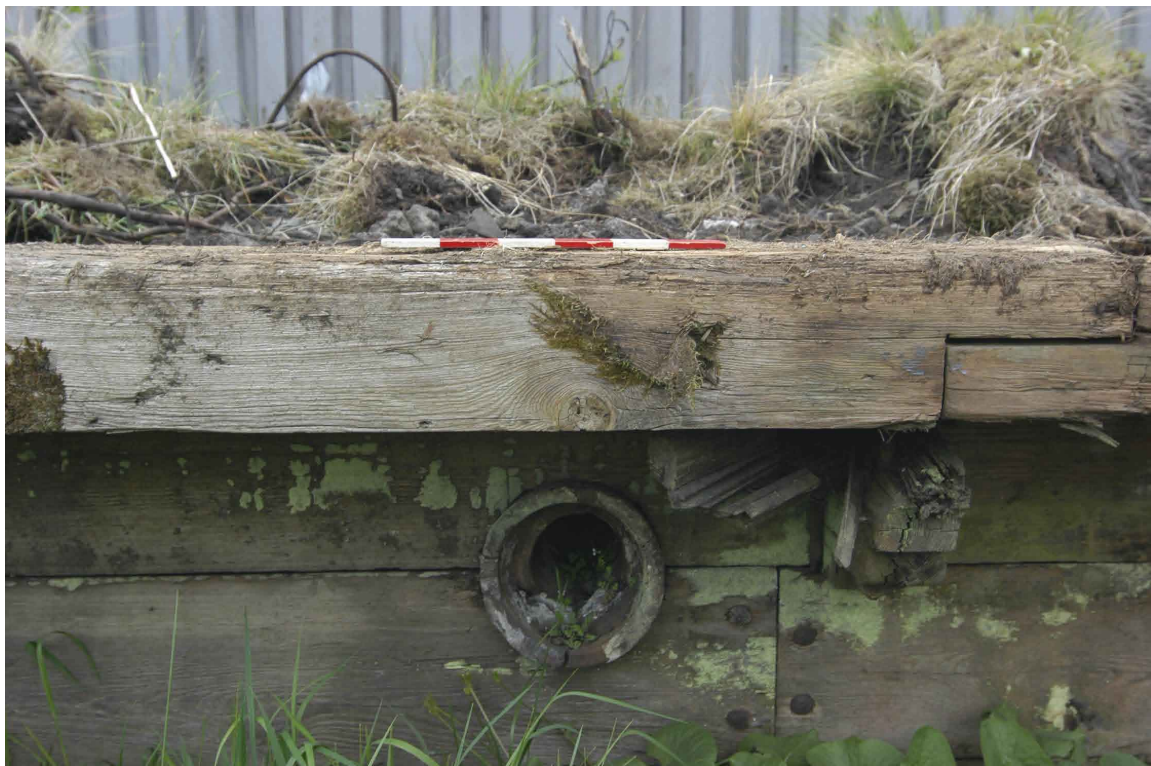
Plate 4 - Timber curb with drain pipe through the lower cladding
