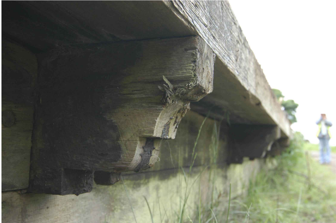
Plate 3 - Moulded timber joist supporting the timber curb
