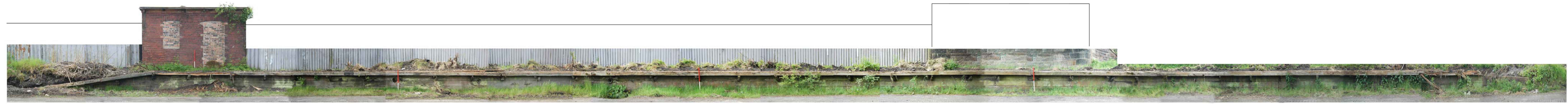
Fig. 3 - Rectified Photograph of the North-facing elevation
