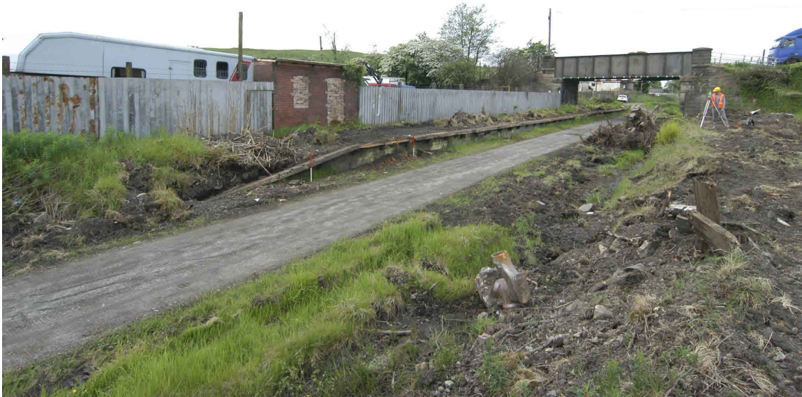
Plate 2 - Forrestfield station; general view of the west-bound platform
