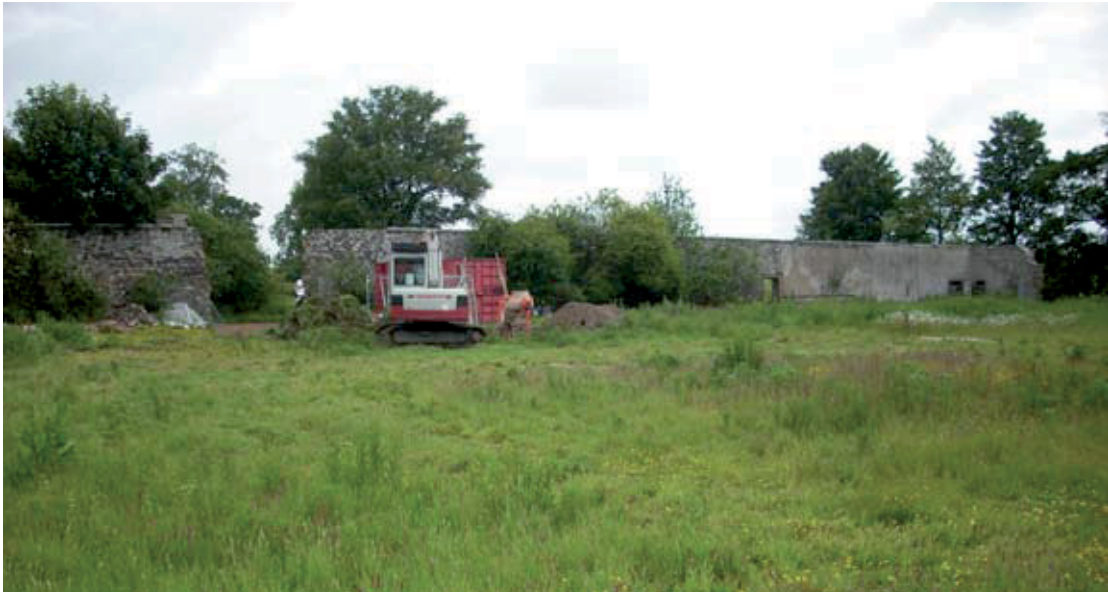
Fig 2 - General pre-ex condition shot of site
