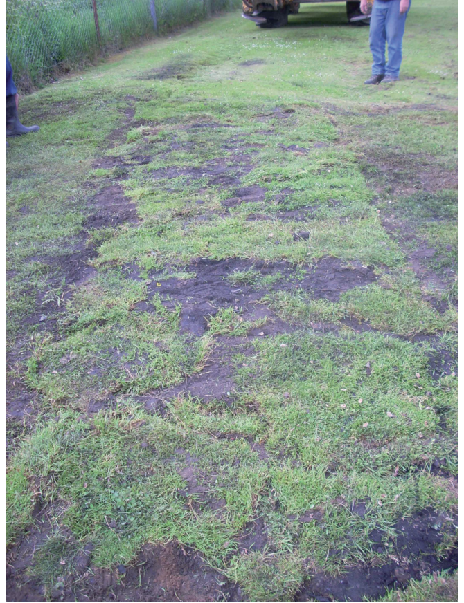
Fig. 3 - Trench 16 after backfilling
