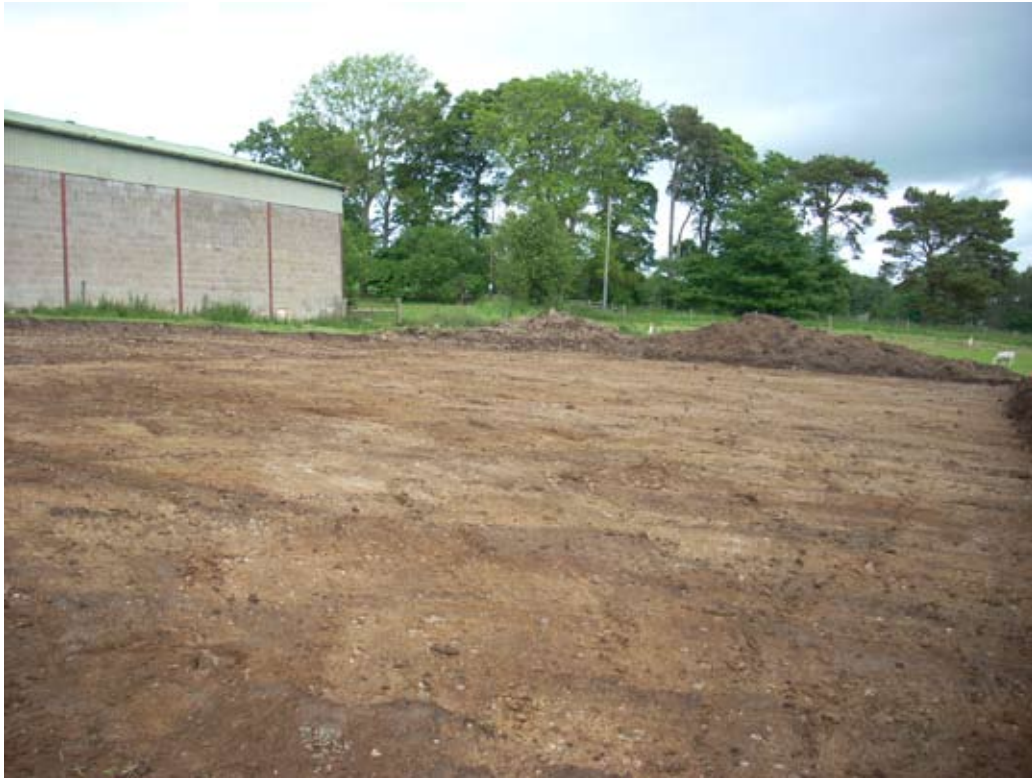
Fig. 2 - Stripped area, looking north
