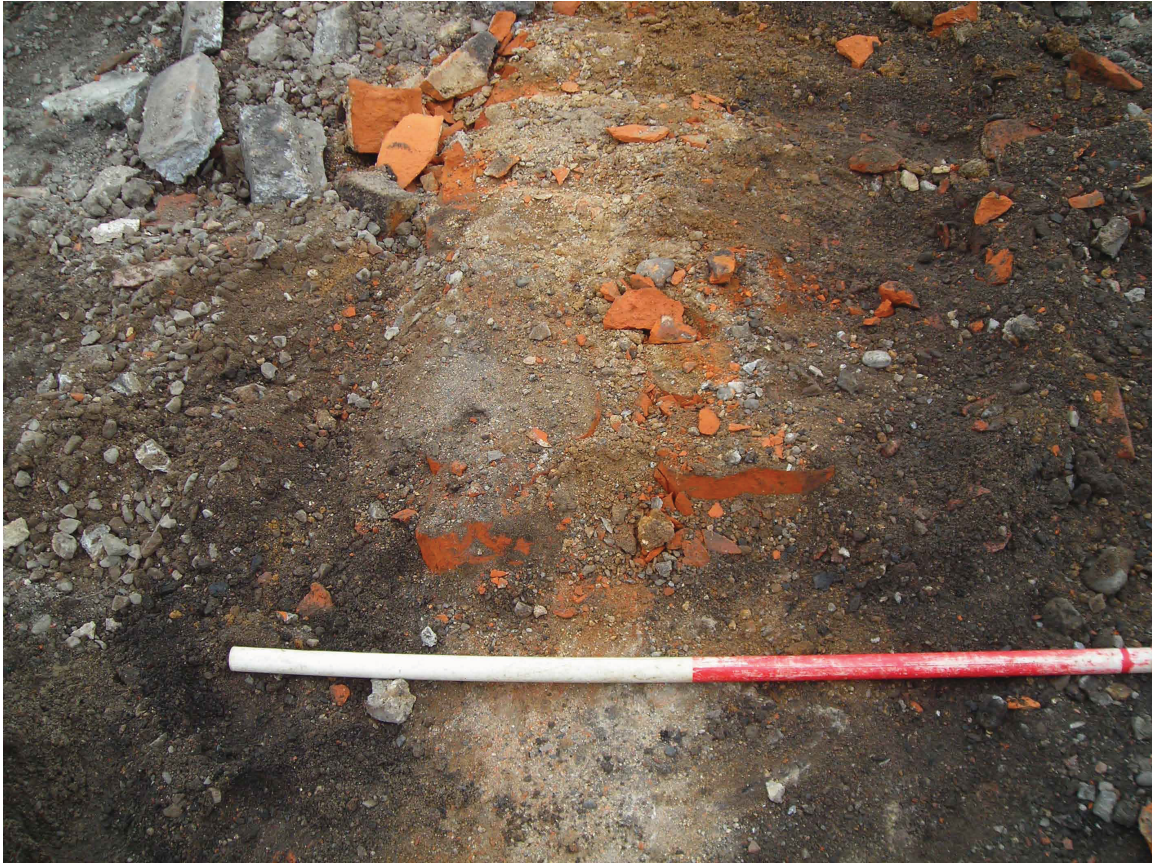
Fig. 2 - Foundation (003) wall footing 004 from the west
