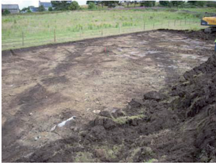
Fig. 4 - Broad rig between Walls 5 & 6
