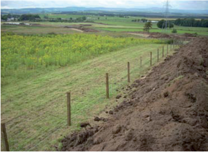
Fig. 2 - General view of the pipeline route looking south-west from near Wall 6
