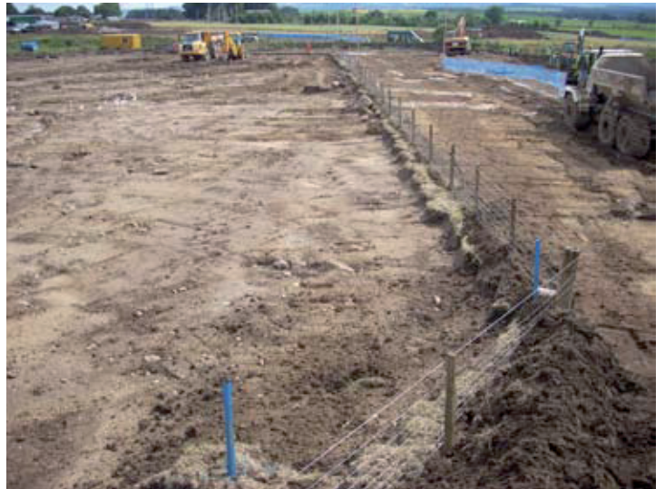
Fig. 5 - Broad rig between Walls 4 & 14 with pond excavation area on the left
