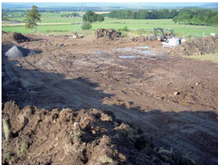
Fig. 6 - Site 2 prior to evaluation
