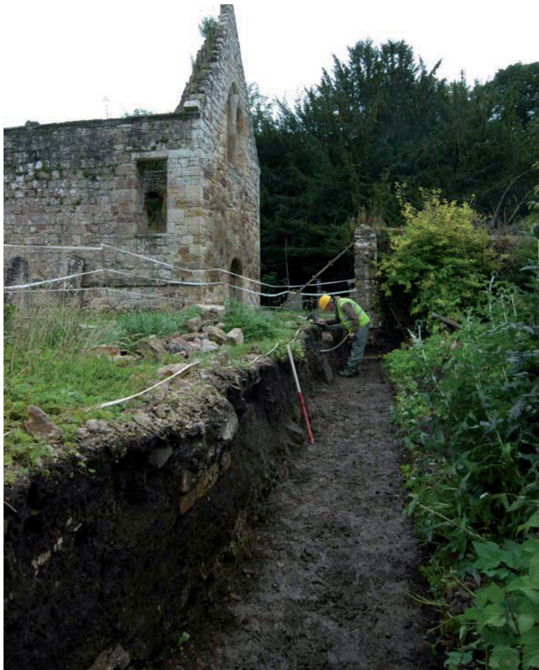
Fig. 12 - General view of foundation trench
