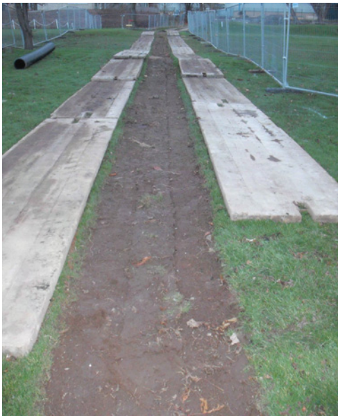
Fig. 3 - Pre-ex shot of drainage trench Area 1 from SE
