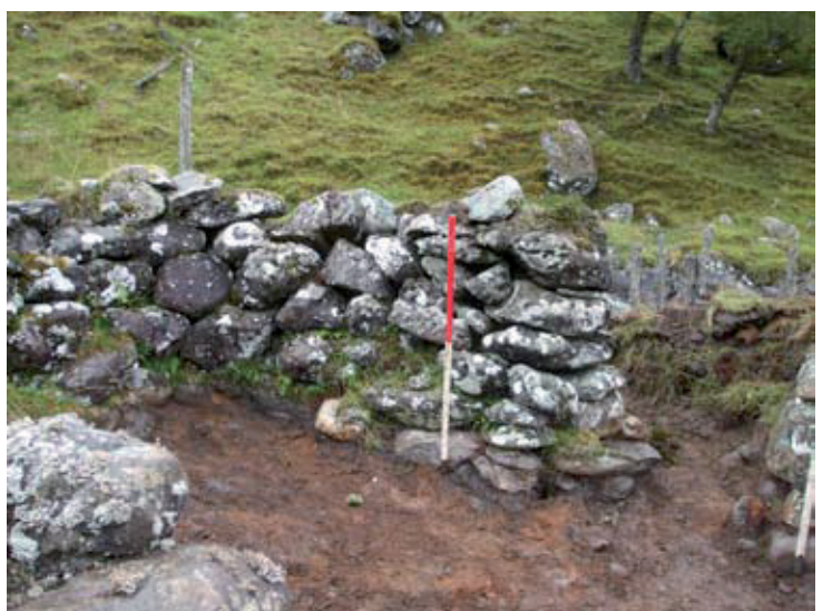
Fig. 9.6 - Internal shot of western corner
