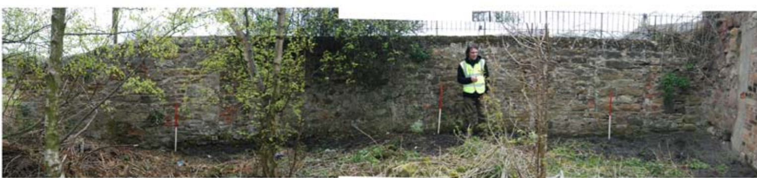
Fig 20b - West Elevation, Photo montage showing the garden wall
