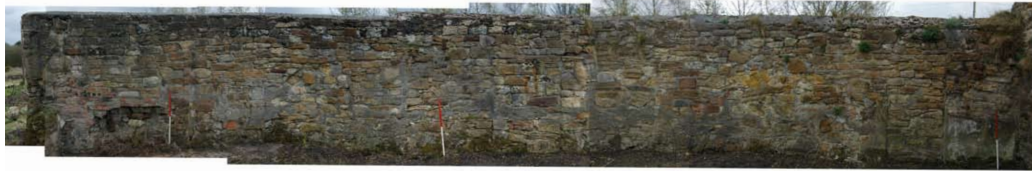
Fig 18b - Montage showing the South internal Elevation of Custom House
