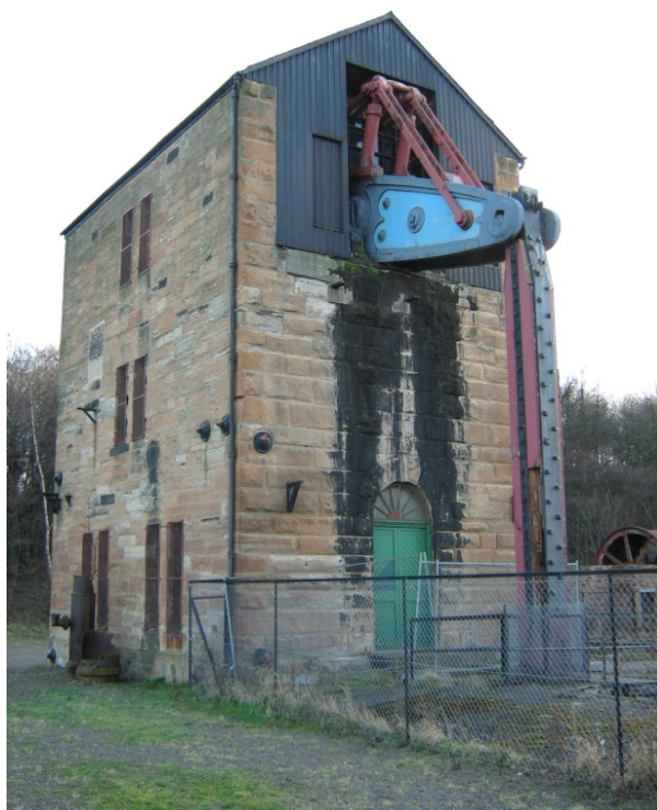
Plate 4 - Cornish beam engine
