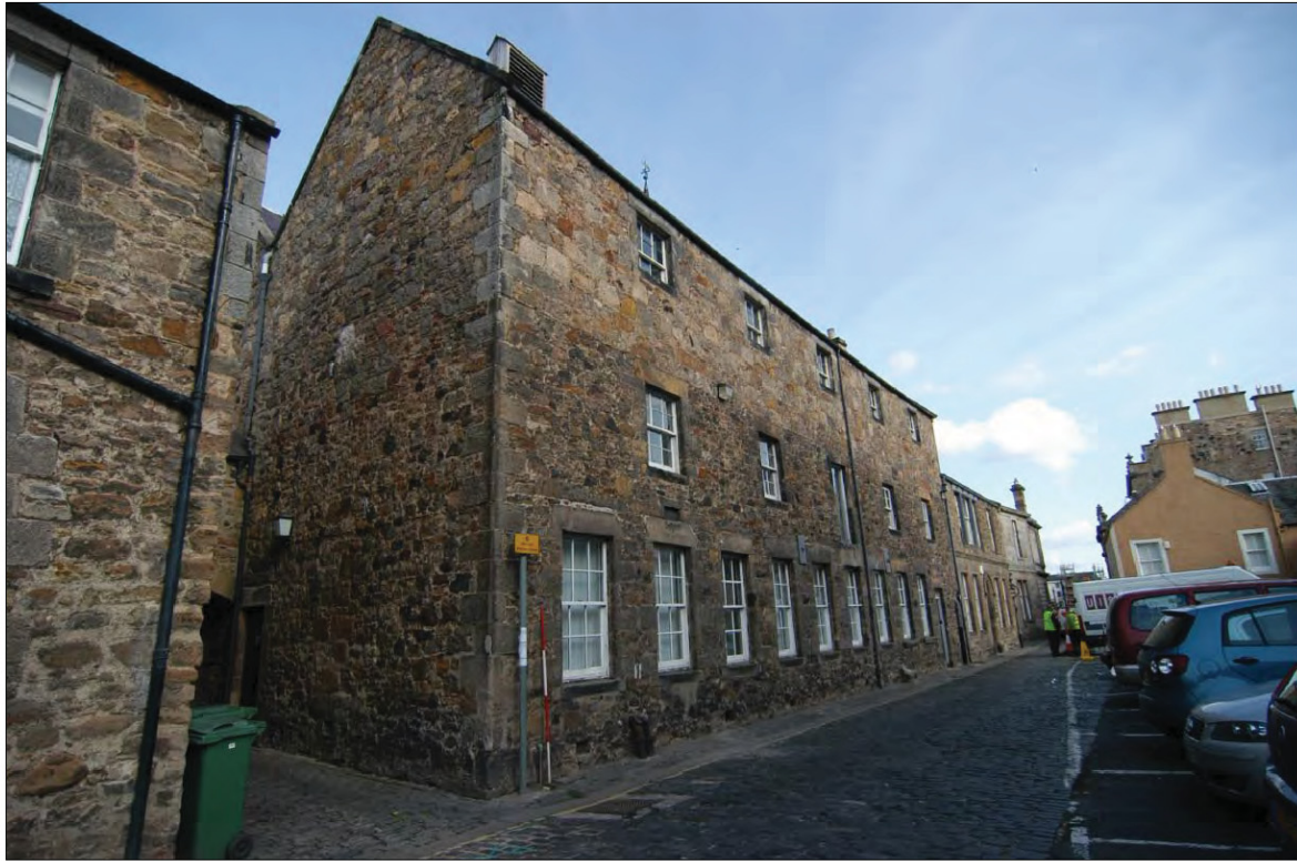
Plate 5 - South-facing elevation of the grain store and buildings Nos 52 and 54 in relation to Lodge Street.
