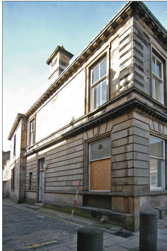
Plate 6 - South-east corner of the former City Bank (No 52).
