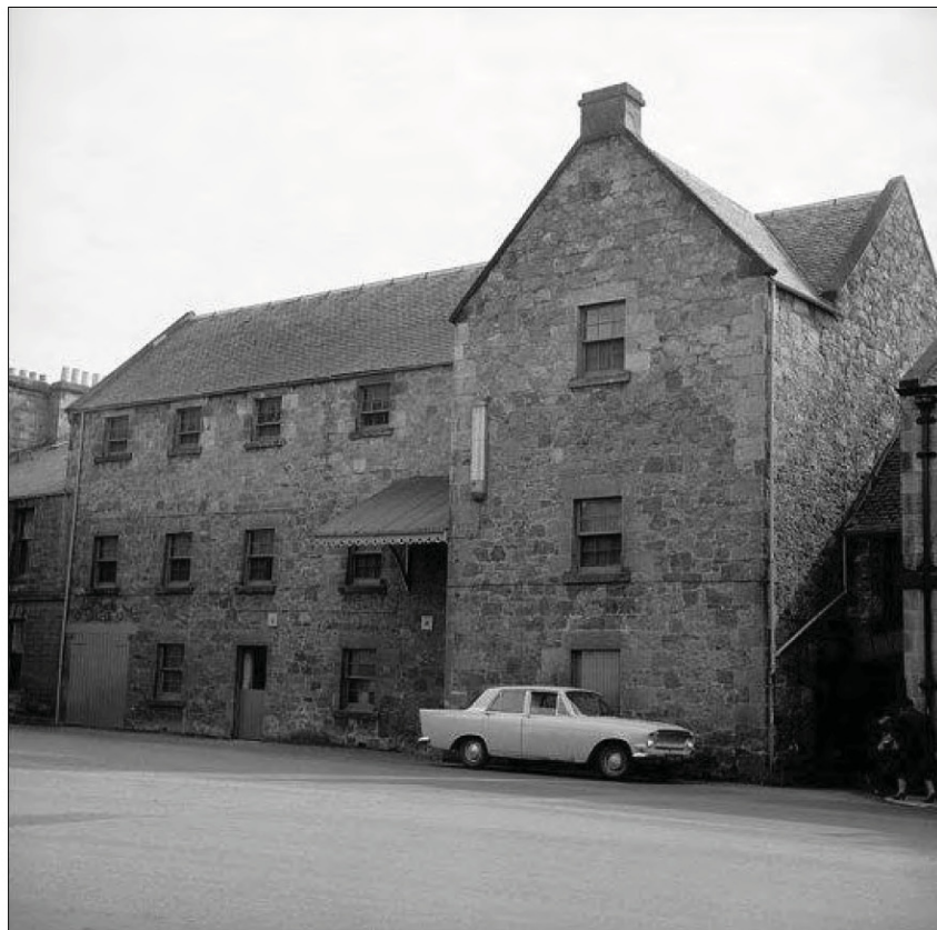
Plate 2 - Historical photograph (1960s) showing the north-facing elevation of the former grain store with a pentice roof.
