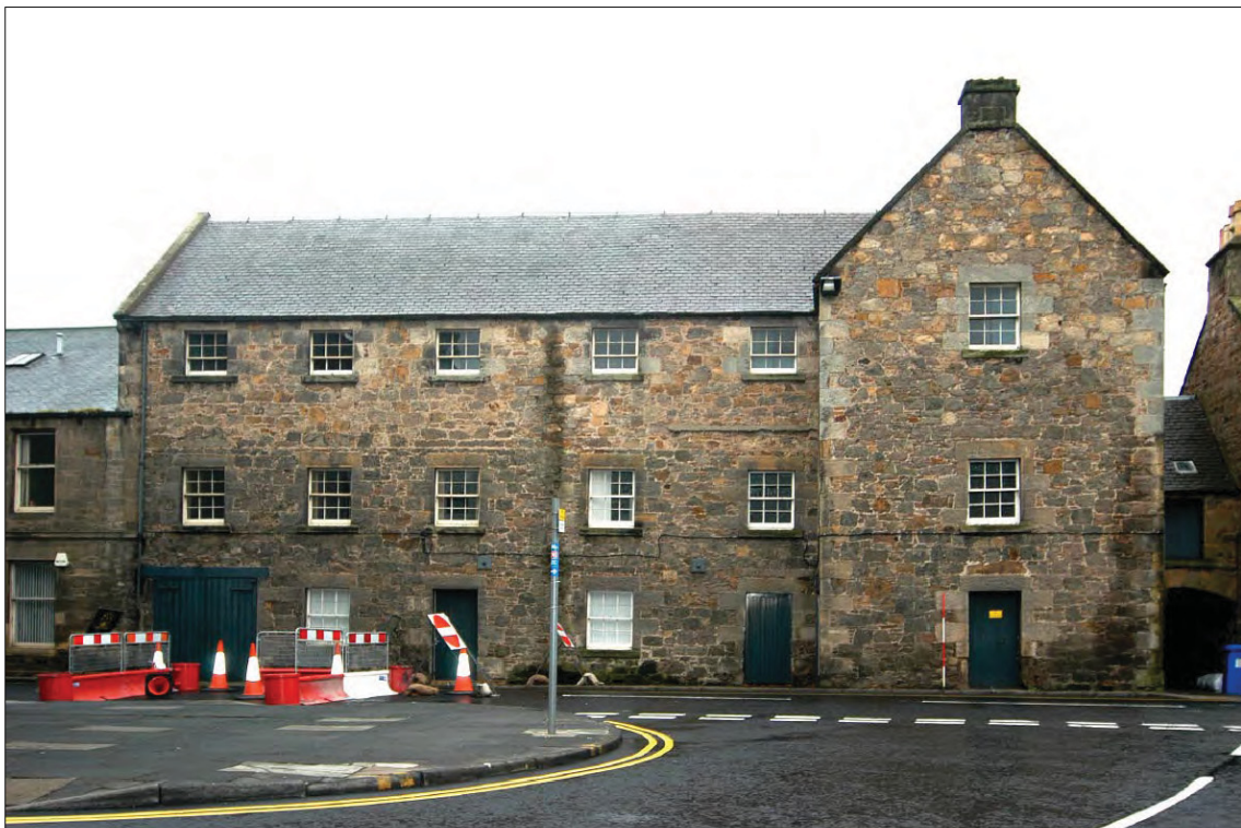
Plate 3 - North-facing elevation of the grain store with contrasting stonework on the second floor.
