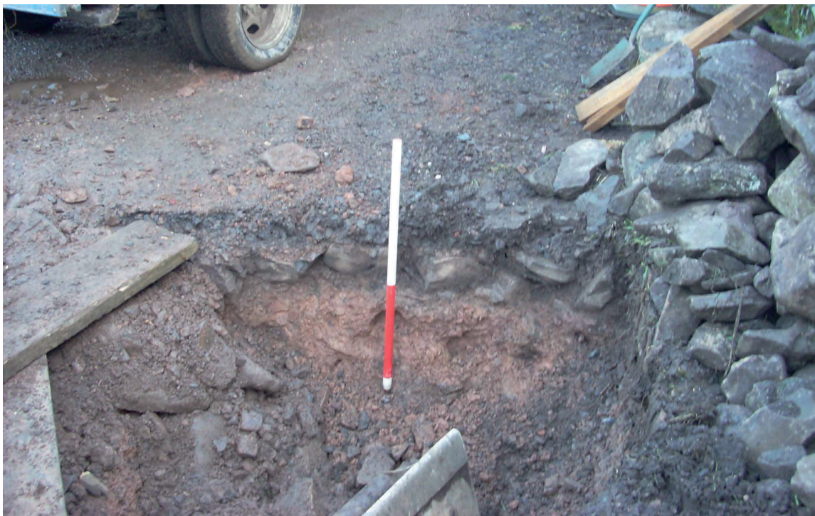
Fig. 4 Section showing the large cobbles of the former yard surface under gravel and over natural subsoil
