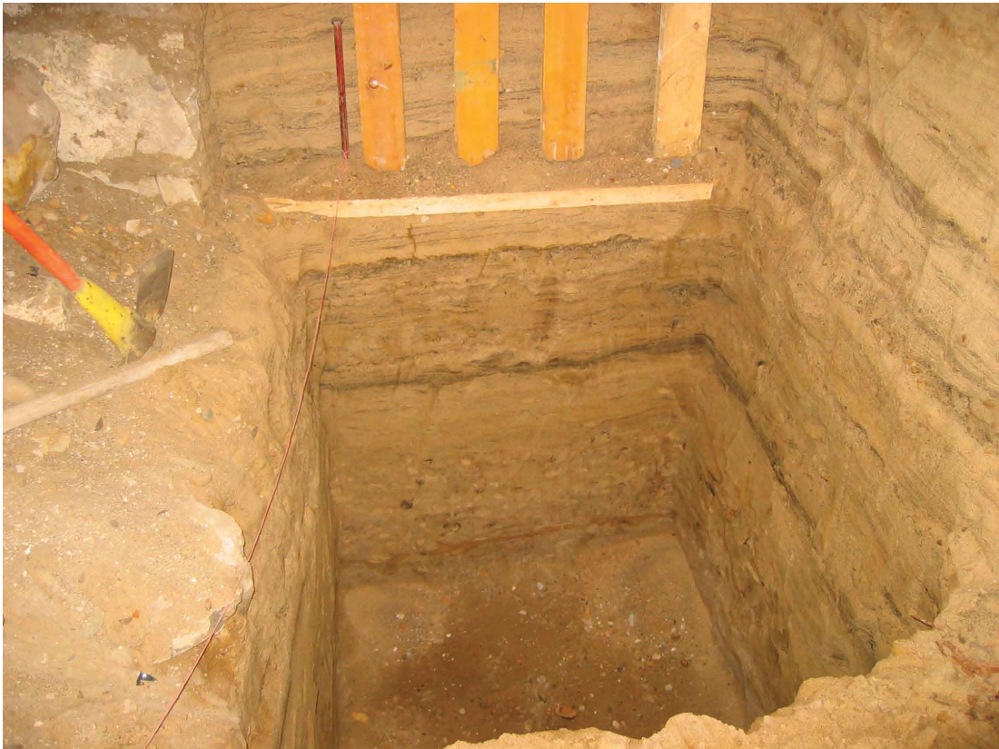
Fig. 3 - Foundation trench of retaining structure
