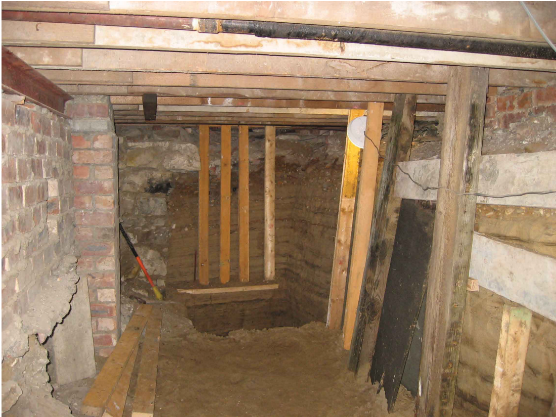
Fig. 2 - Area after removal of bank of sand
