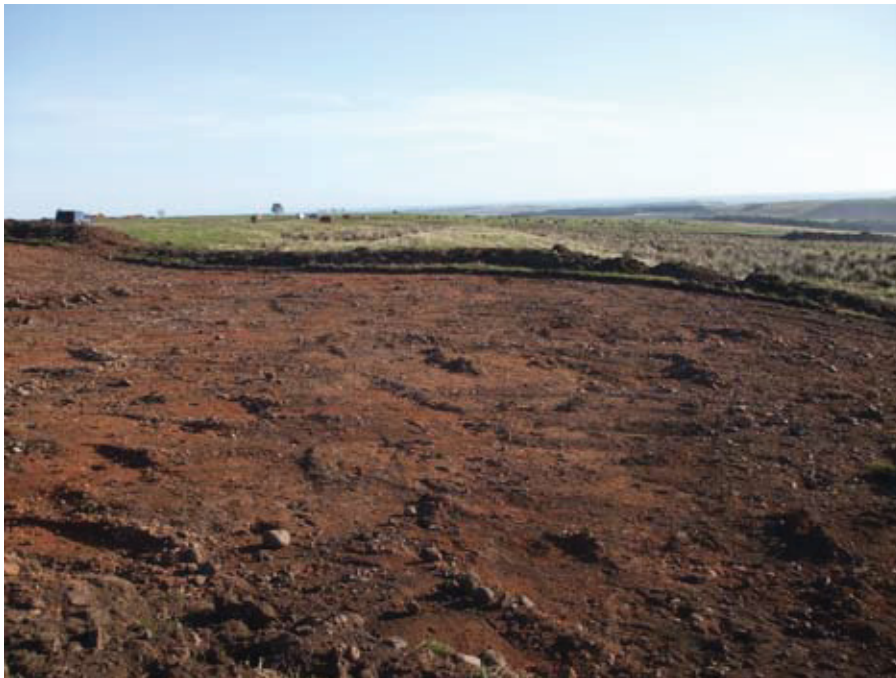
Figure 10 - Area stripped for turbine base 7 showing natural terrace
